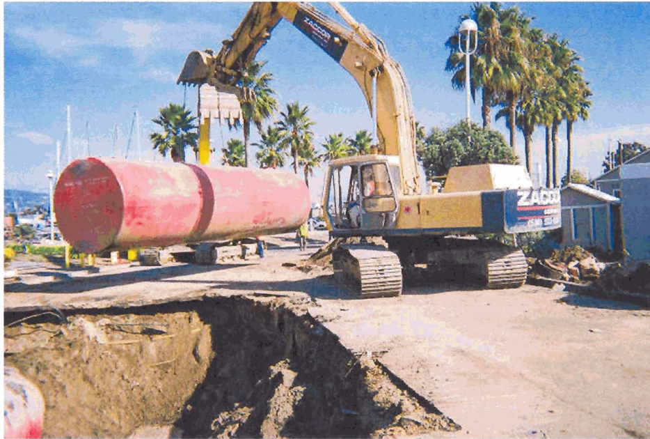
Photo 3 – Diesel UST removed and heading for the transport truck.
