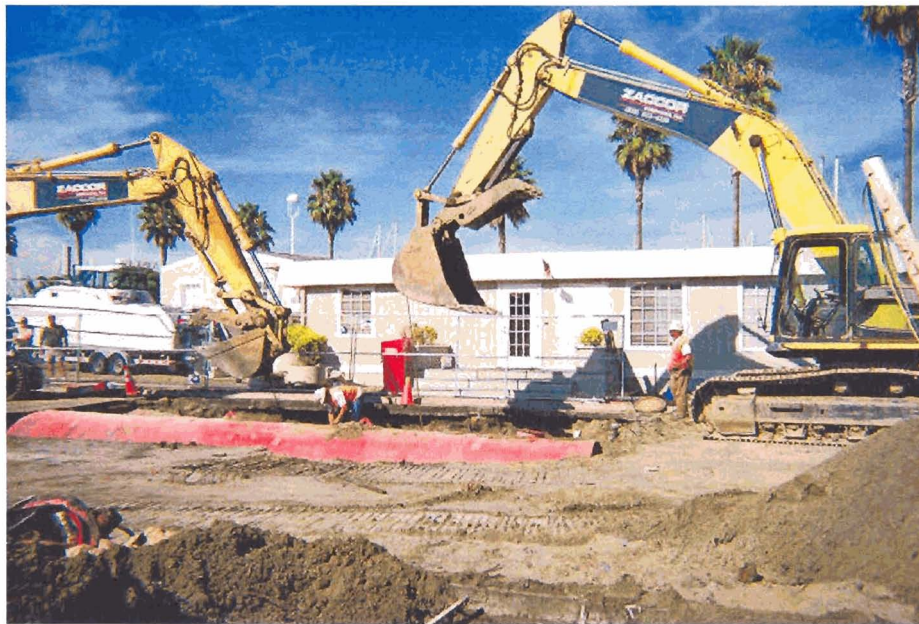
Photo 2 – Preparing for tank removal at Grand Marina
