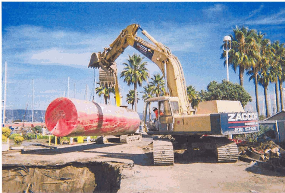
Photo 4 - Gasoline UST removed and being lifted to transport truck.
