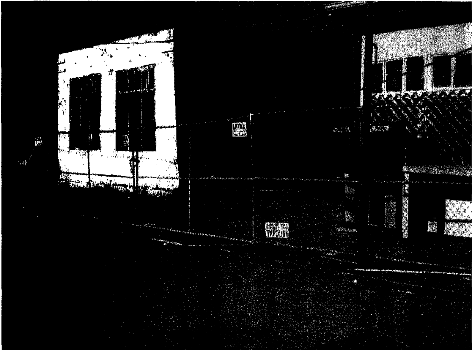
Photograph looking north from 37 th Street. The photograph shows a view of the south side of the repair garage and kiosk..
