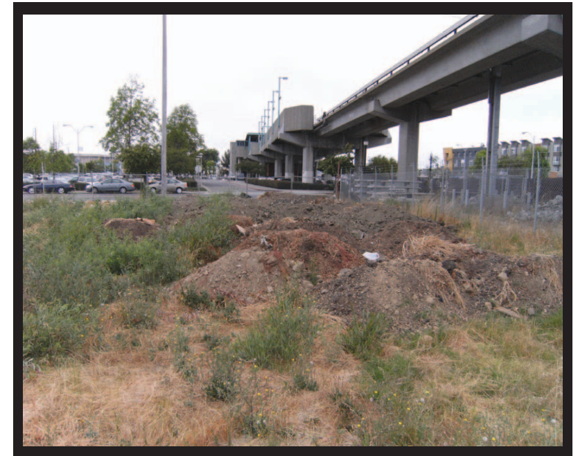
1) View of soil debris piles in the northwestern portion of the Site.
