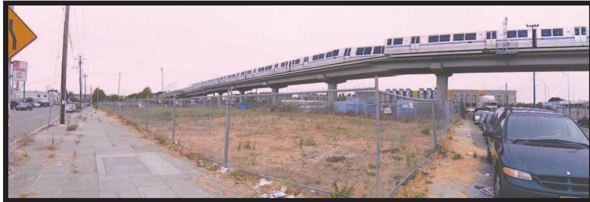
1) View of the Site from the southeast to the northwest.
