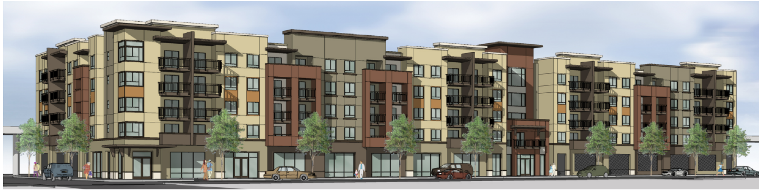
5TH STREET AT CORNER LOBBY
