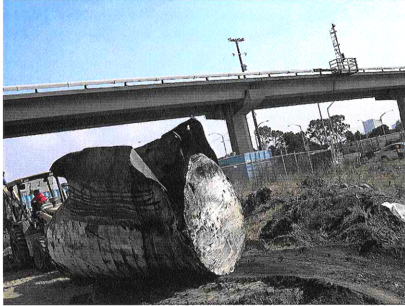
Photograph 3 – 3,000-gallon tank removed.
