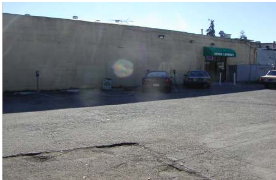
6. North view and rear of subject property.
