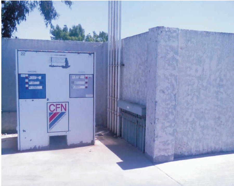
Photo 2. Closer view of vent lines and work area.
