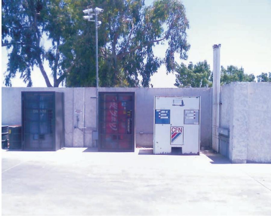
Photo 1. View of vent line area and work area.
