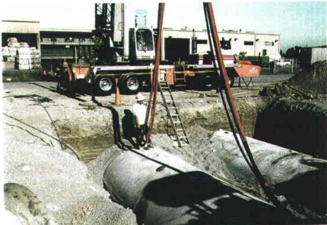
Photograph of tank removal.
