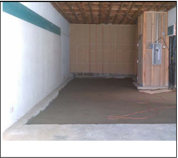
32 - Final Cement Slurry Surface in 1185 Solano (before Future Slab)
