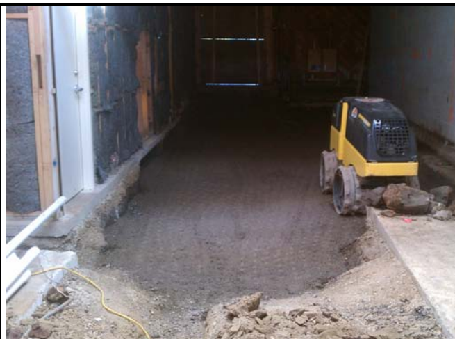
15 - Compaction after Initial Backfilling in 1187 Solano
