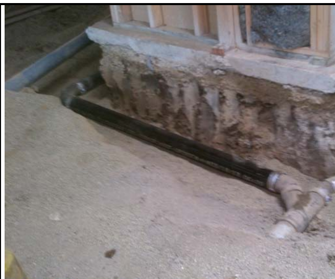
29 - New Sanitary Sewer Piping under 1185 and 1187 Solano
