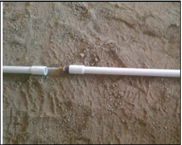
44 - Soil Gas Probe in Gravel Layer before Final Connection
