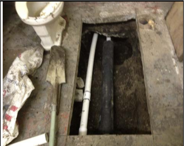
34 - 1191 Solano Vent Pipe before Seal and Sand
