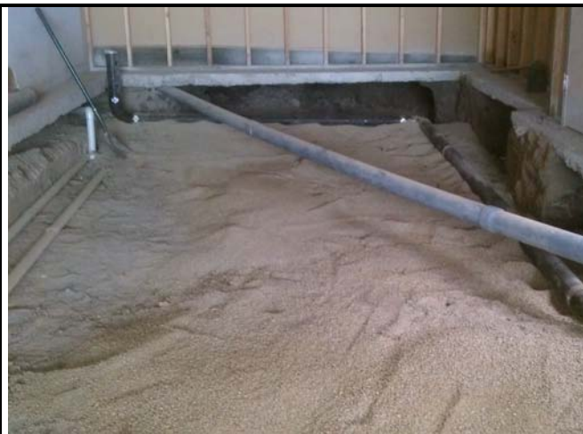
23 - Gravel Installation in 1185 Solano
