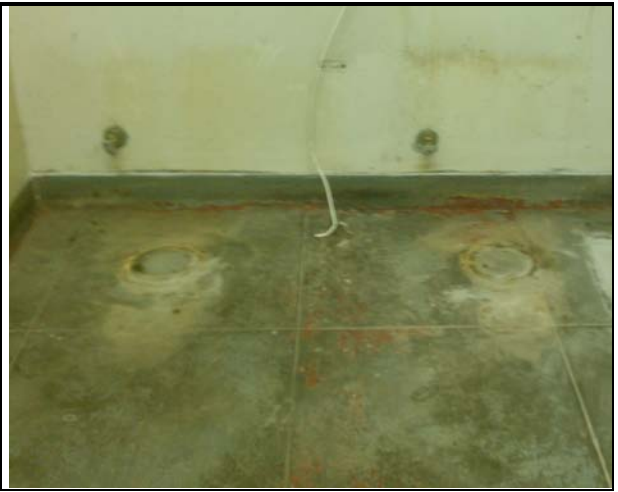
38 - Sealing of Former Toilets and Water Supply in Storage Room in 1191 Solano
