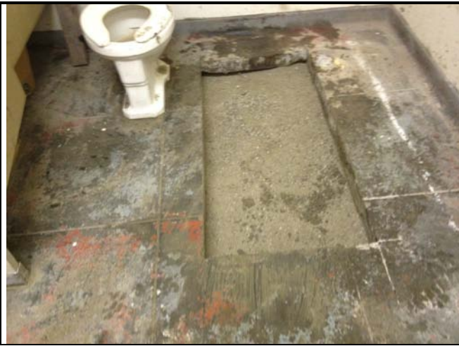
37 - 1191 Solano Vent Pipe after Sand Backfill
