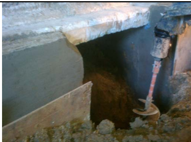
9 - Excavation Augering Between Slots under 1191 Solano
