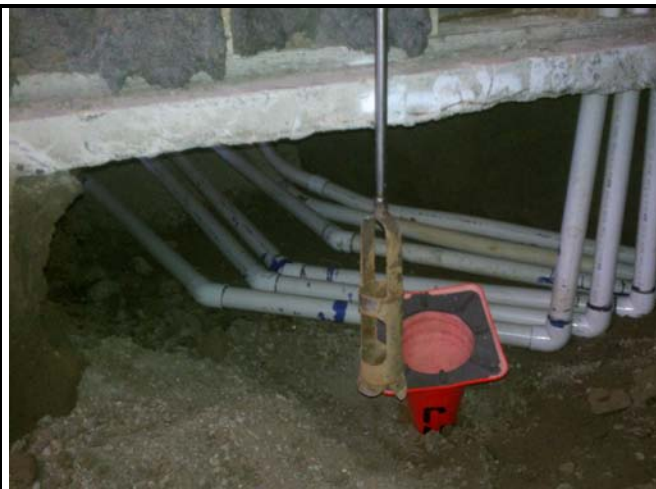
25 - Manifold of Vent Piping from All Units
