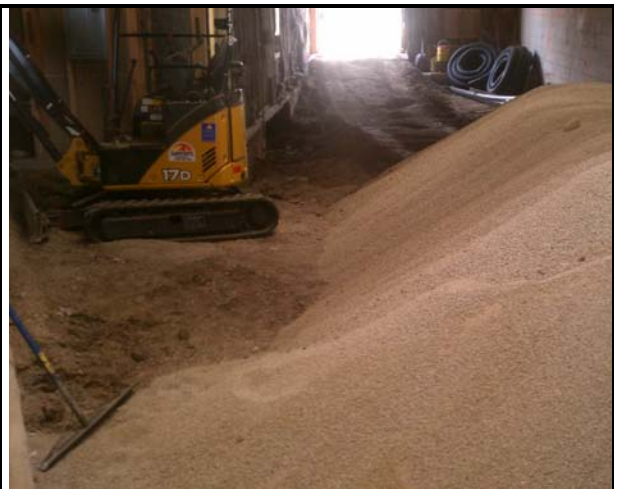
22 - Gravel for Passive Venting System under 1185 and 1187 Solano
