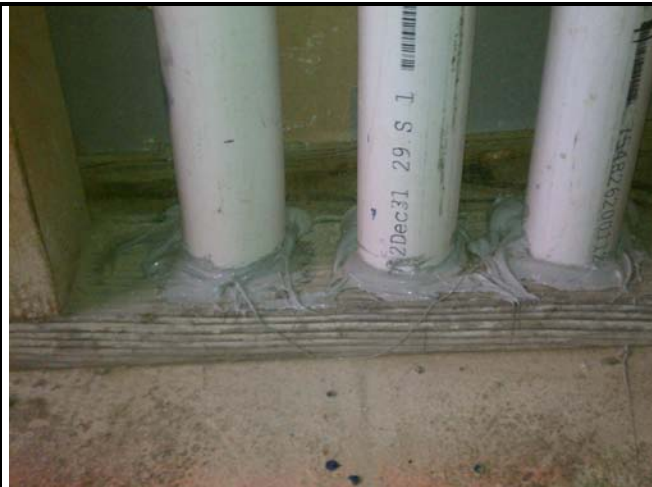
41 - Sealing of Vent Piping Penetrations
