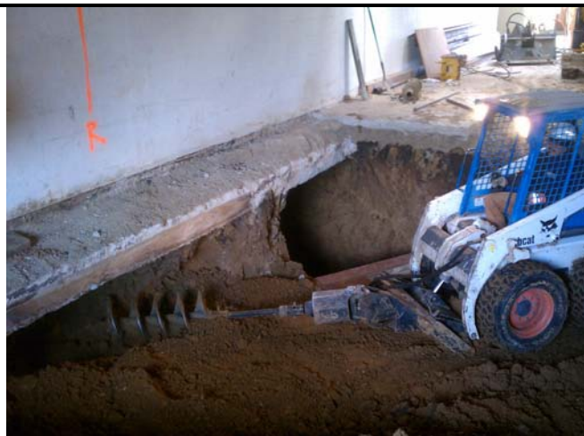
7 - Initial Auger Excavation in Slots under 1191 Solano
