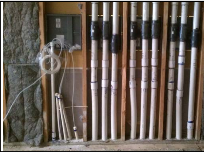
43 - Manifold Piping w probes and MW-4
