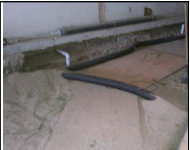
26 - Passive Ventilation System in 1185 Solano
