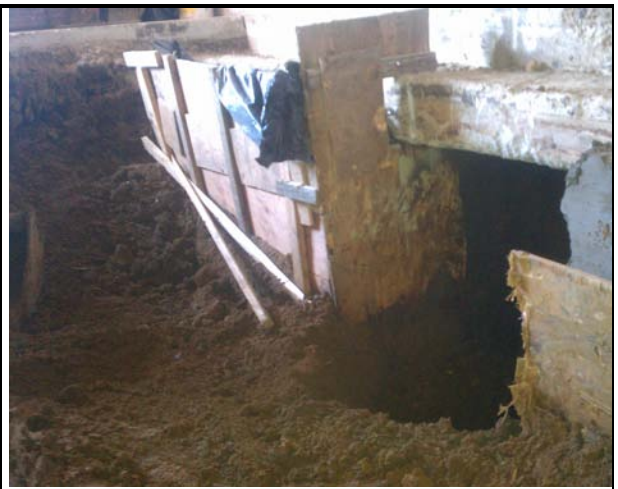
8 - Forming Cement Slurry Slots under 1191 Solano
