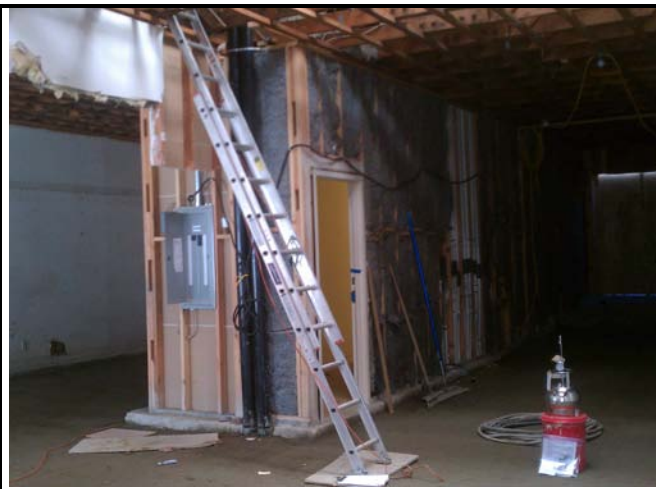
45 - Passive Vent Risers and Indoor Air Sampling
