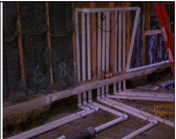
16 - Piping Manifold for Temporary Ventilation System (later removed)
