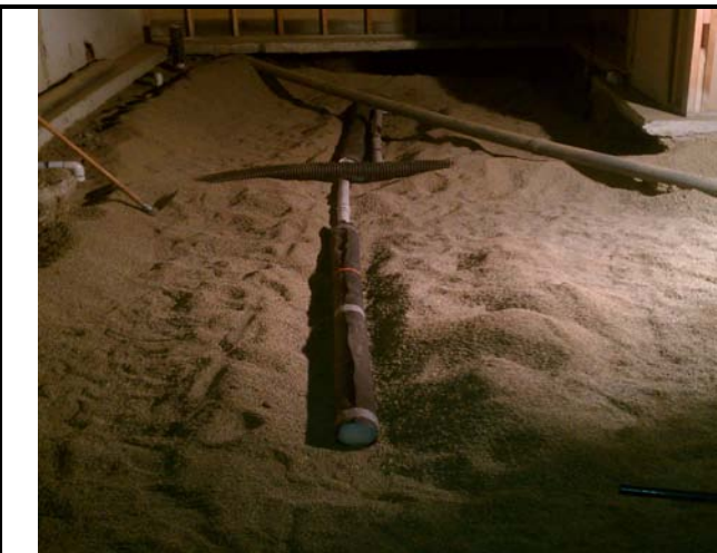
27 - Vent Piping for Active or Passive Extraction in 1185 Solano
