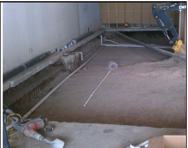
24 - Vent Piping Installation after Backfilling with Sand in 1185 Solano
