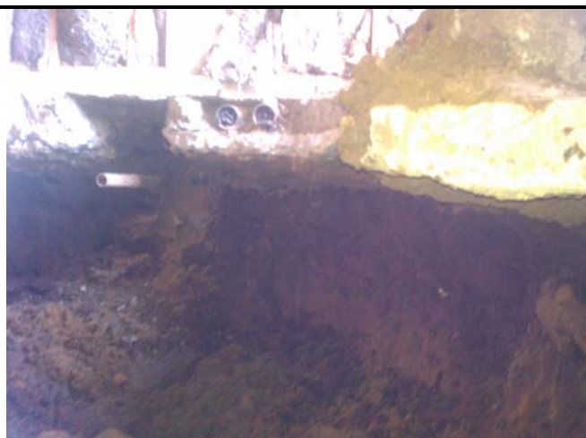
9 - Excavation Augering Between Slots under 1191 Solano
