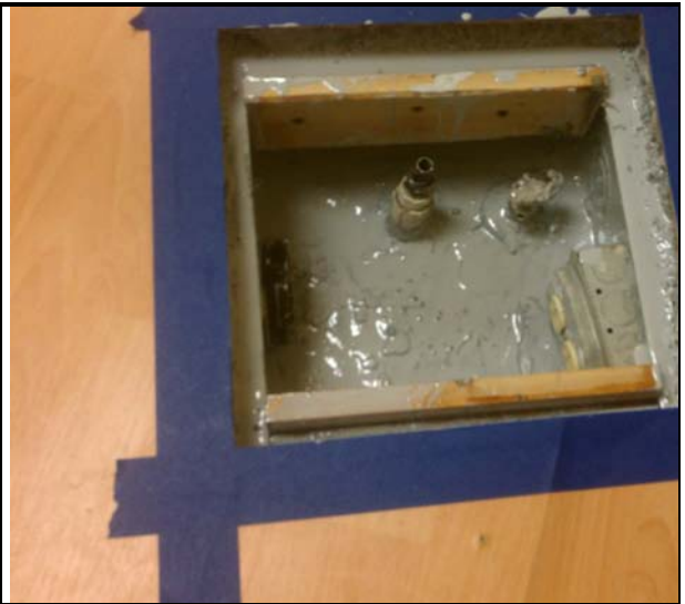
40 - Sealing of Chair Utilities in 1183 Solano
