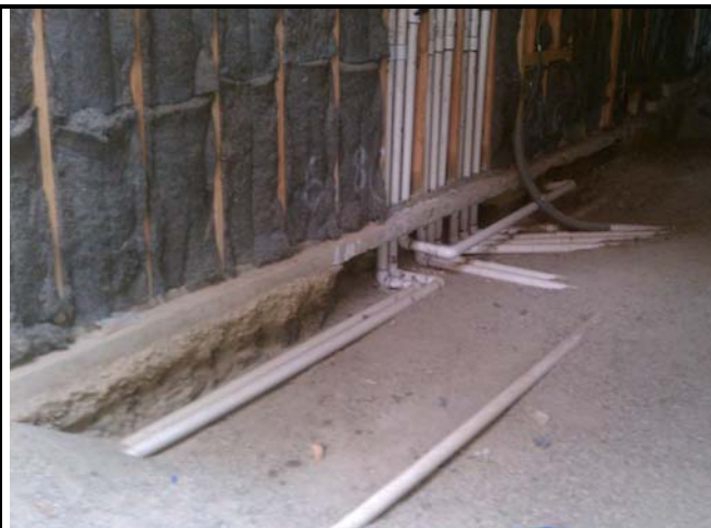
17 - Temporary Vent Piping After Initial Excavation (later removed)
