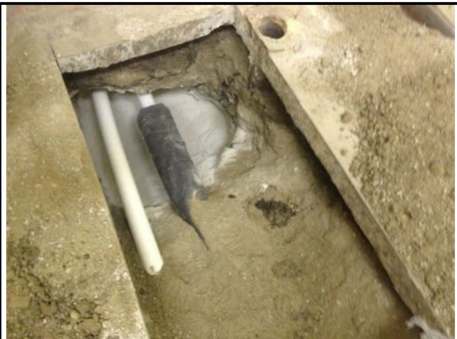
35 - 1191 Solano Vent Pipe with Bentonite Seal
