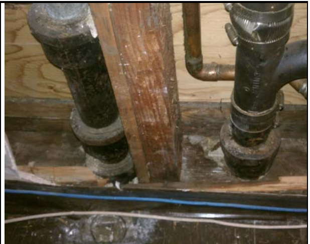
42 - Slab Penetrations before Sealing in 1191 Solano
