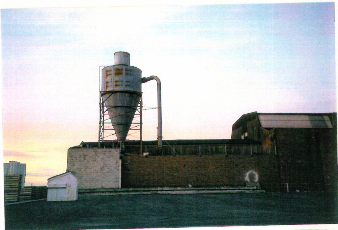
Photograph #2: West wall of the former Rifkin building. Note the cyclone separator on top of the building.
