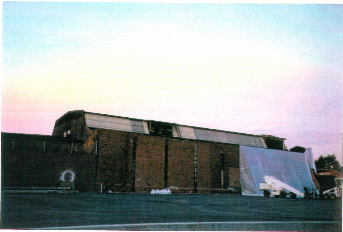
Photograph #1: East wall of the former Rifkin building. The first three bays are covered by polycurtains.
