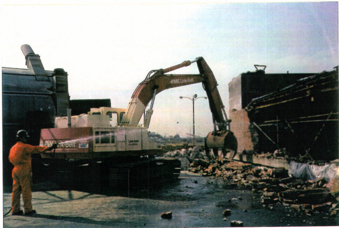
Photograph #4: Excavator demolishing the west wall of the former Rifkin building.
