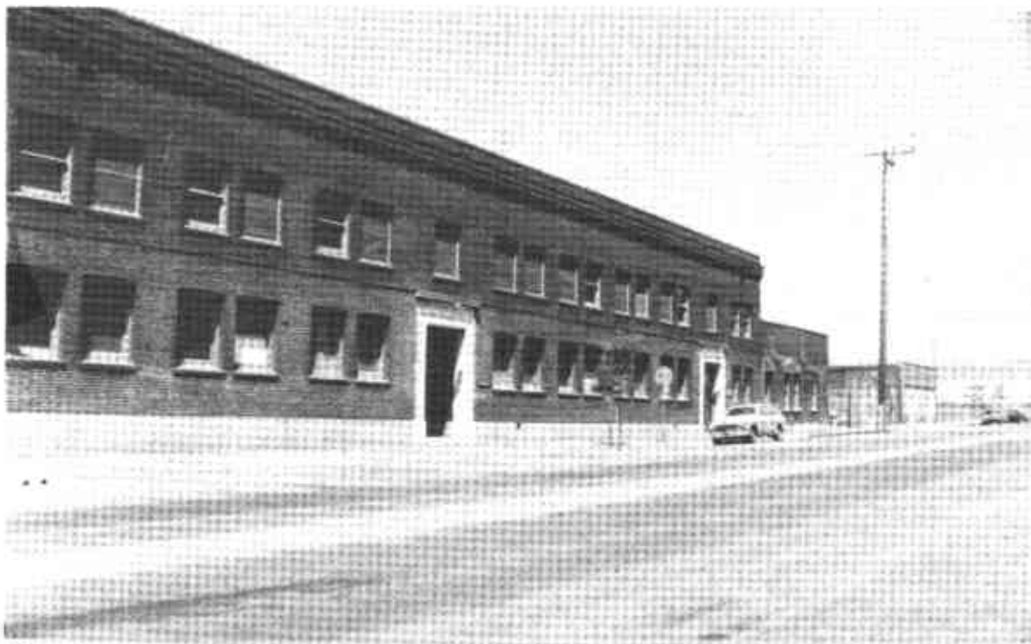
B. Existing Cannery building looking northeast along Park Avenue
