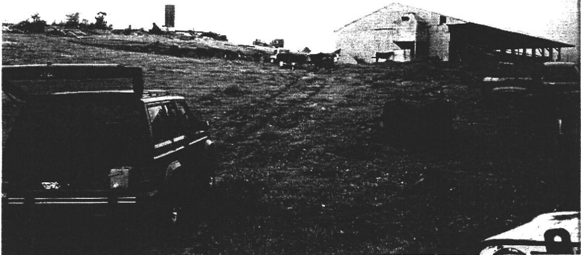
PHOTOGRAPH #3 Northernmost barn/stable located on Soda West Property.
