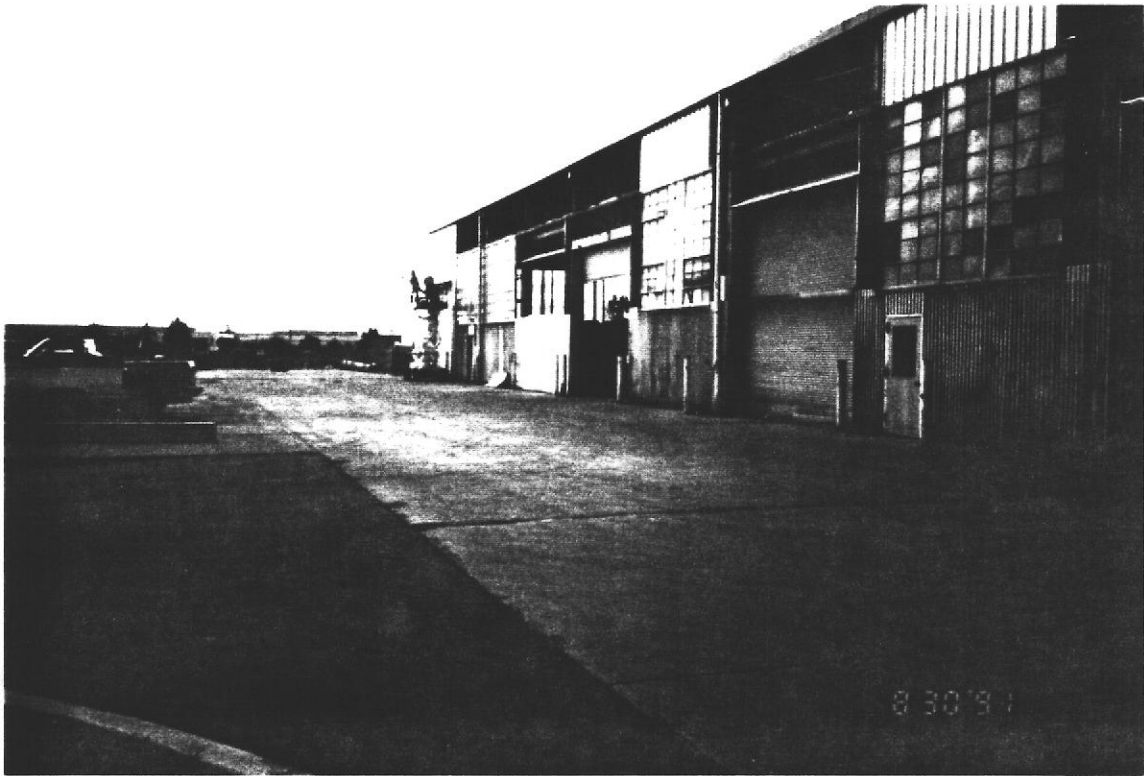
1. Looking south at east side of Building 1
