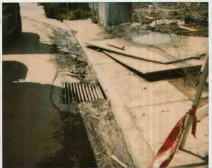
5/13/98 Storm drain along Filadelfia St near Pavell St.
