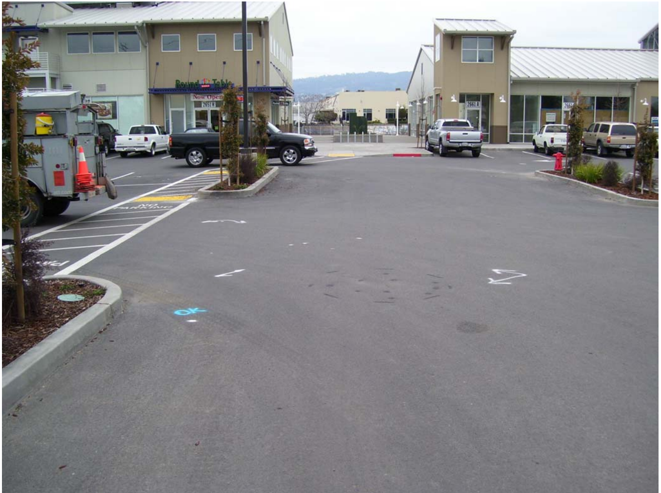
Photo 8 (MW-3). The photo above shows the survey area of MW-3. The anomaly identified in this area is denoted by the black spray paint shown on the asphalt pavement near the center of the photo. This photo was taken looking northeast.
