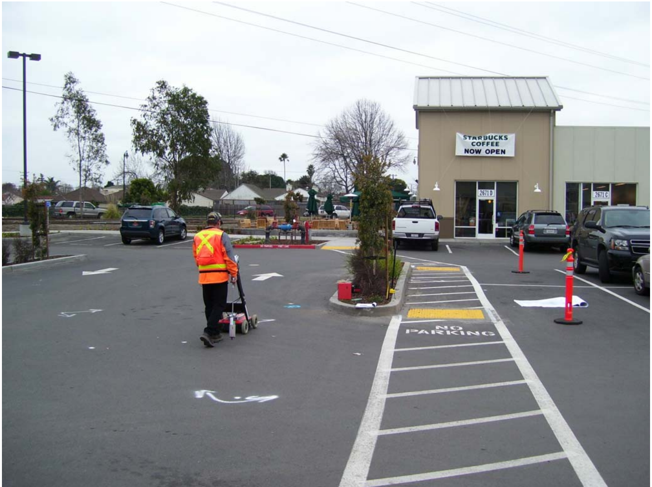
Photo 7 (MW-3). The photo above shows the GPR survey is being performed in the survey area of MW-3. The survey was conducted around the entire boundary of the parking lot island shown in the center of the photo. Photo was taken looking southwest.
