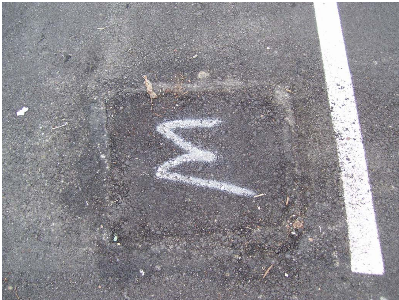
Photo 2 (MW-1). The photo above shows the cut area in the asphalt parking lot where Mid-State Construction stated that MW-1 was buried beneath approximately 2' to 3' of base rock and asphalt cover. Photo was taken looking northeast.
