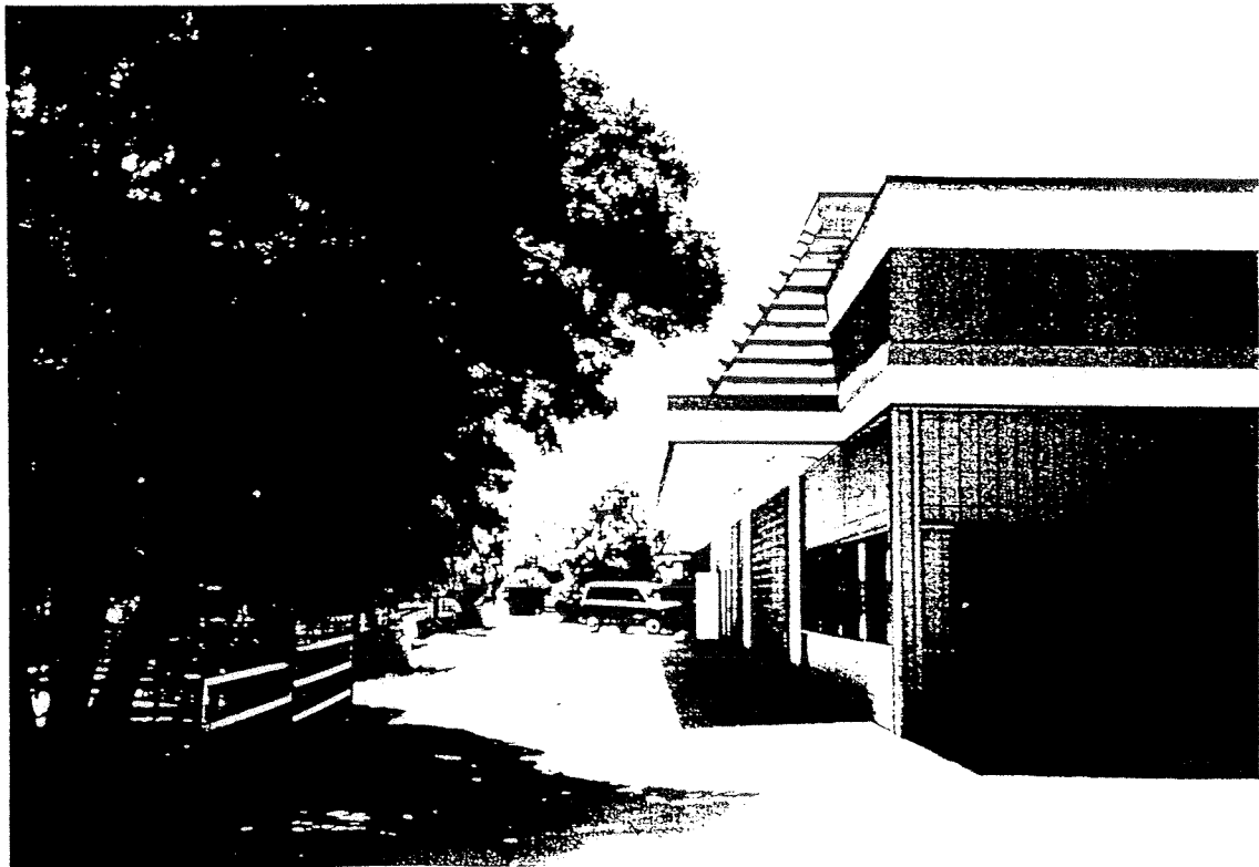
Photograph No. 6 Rear view of Building "B".
