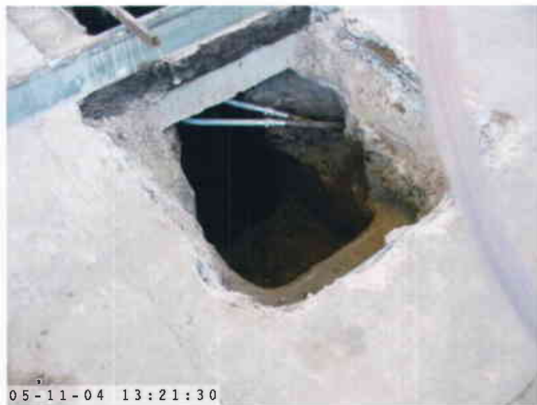
EBMUD 589 LEWELLING BLVD., SAN LORENZO MAY 11, 2004 DIESEL UDC OVEREXCAVATION FOR SOURCE REMOVAL
