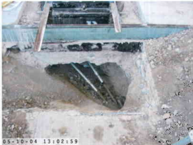
EBMUD 589 LEWELLING BLVD., SAN LORENZO MAY 10, 2004 UDC INSTALL, DIESEL DISPENSER SOIL EXCAVATION
