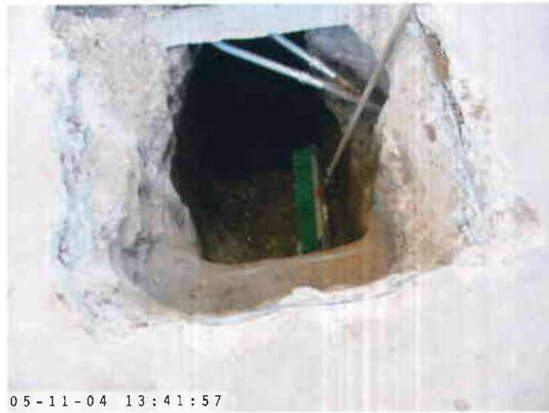
EBMUD 589 LEWELLING BLVD., SAN LORENZO MAY 11, 2004 DIESEL UDC OVEREXCAVATION FOR SOURCE REMOVAL
