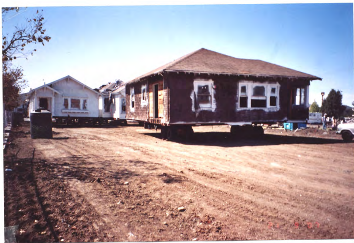
PLATE 5 Residence Being Transported for Restoration at 1085 41st. Street
