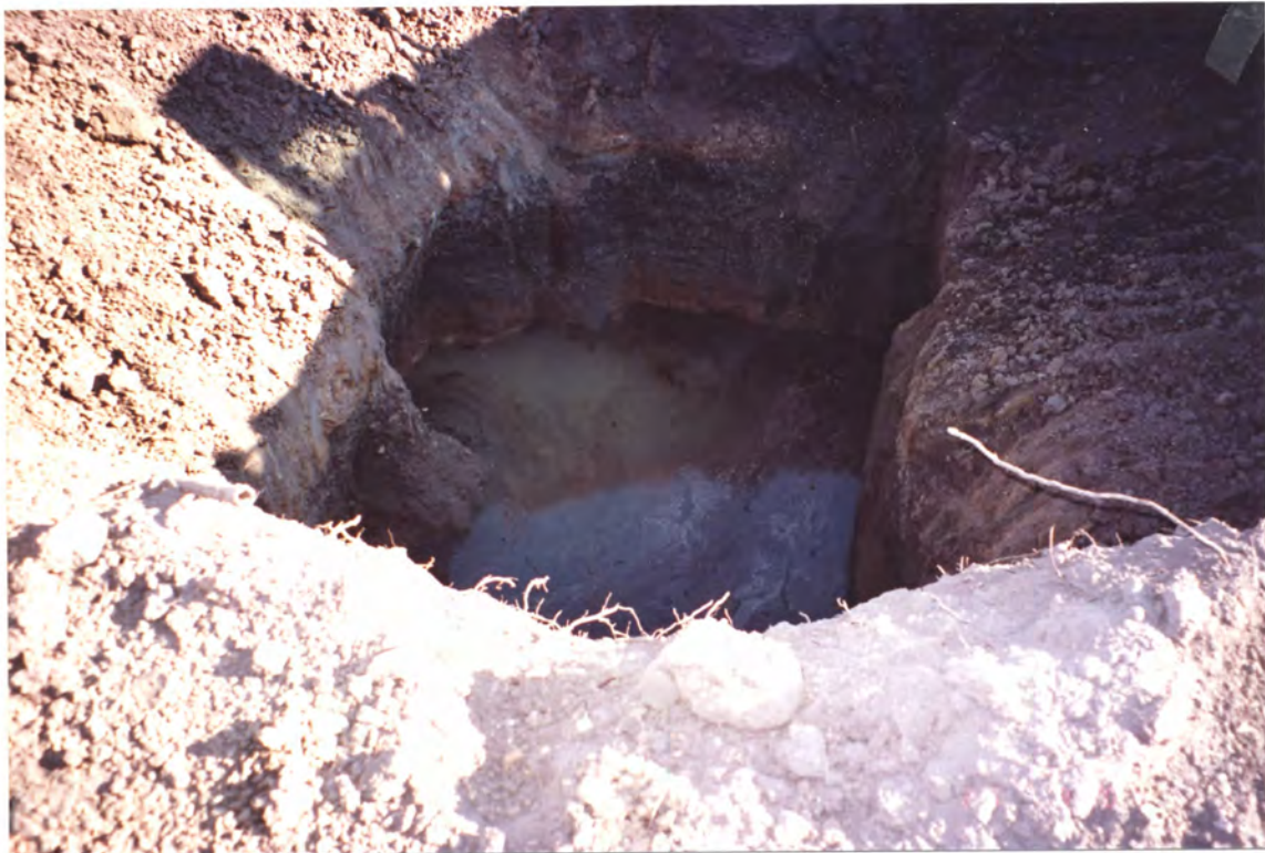
PLATE 4 Groundwater Extraction Pit (Note: Groundwater became clear after extraction of 21,000 gallons.)
