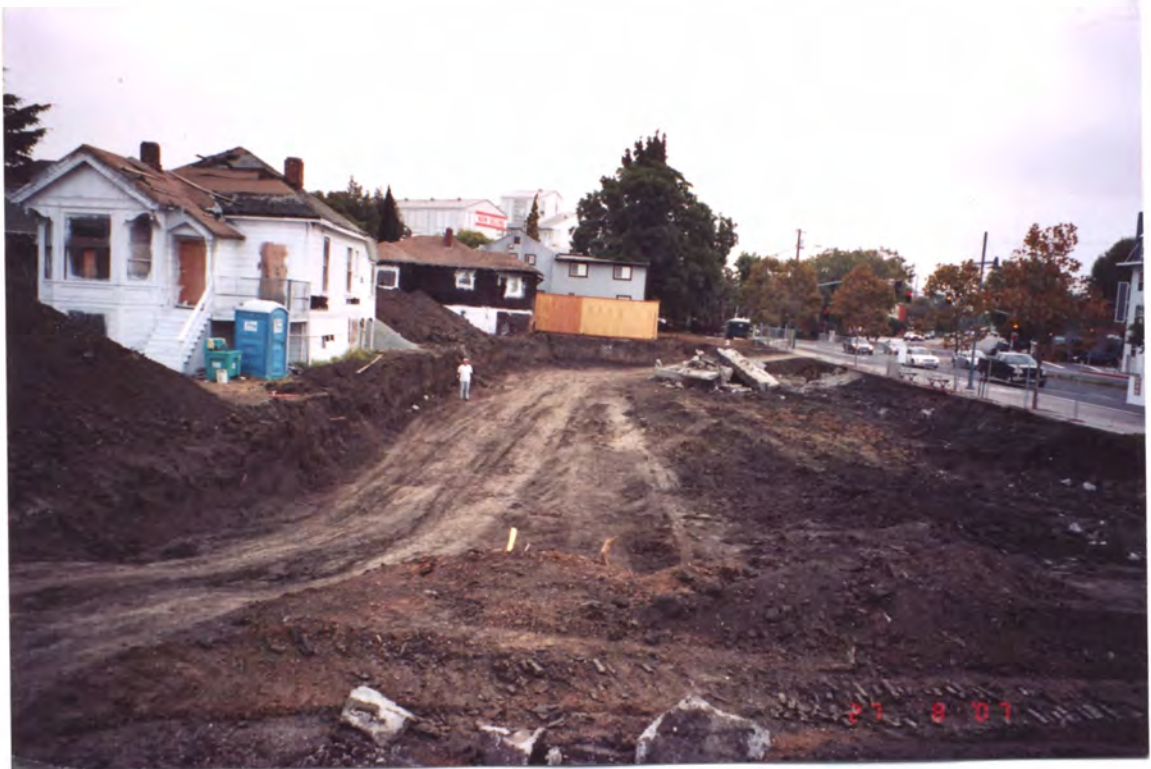
PLATE 3 Remedial Excavation No. 2
