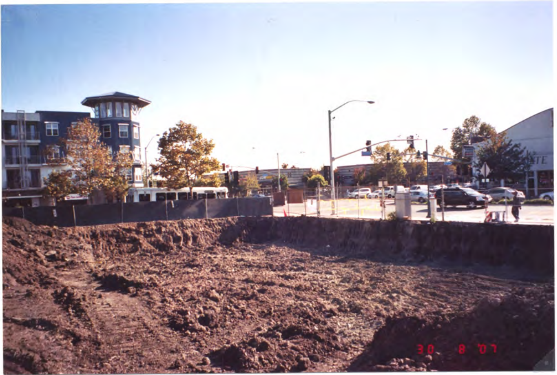
PLATE 2 Remedial Excavation No. 1
