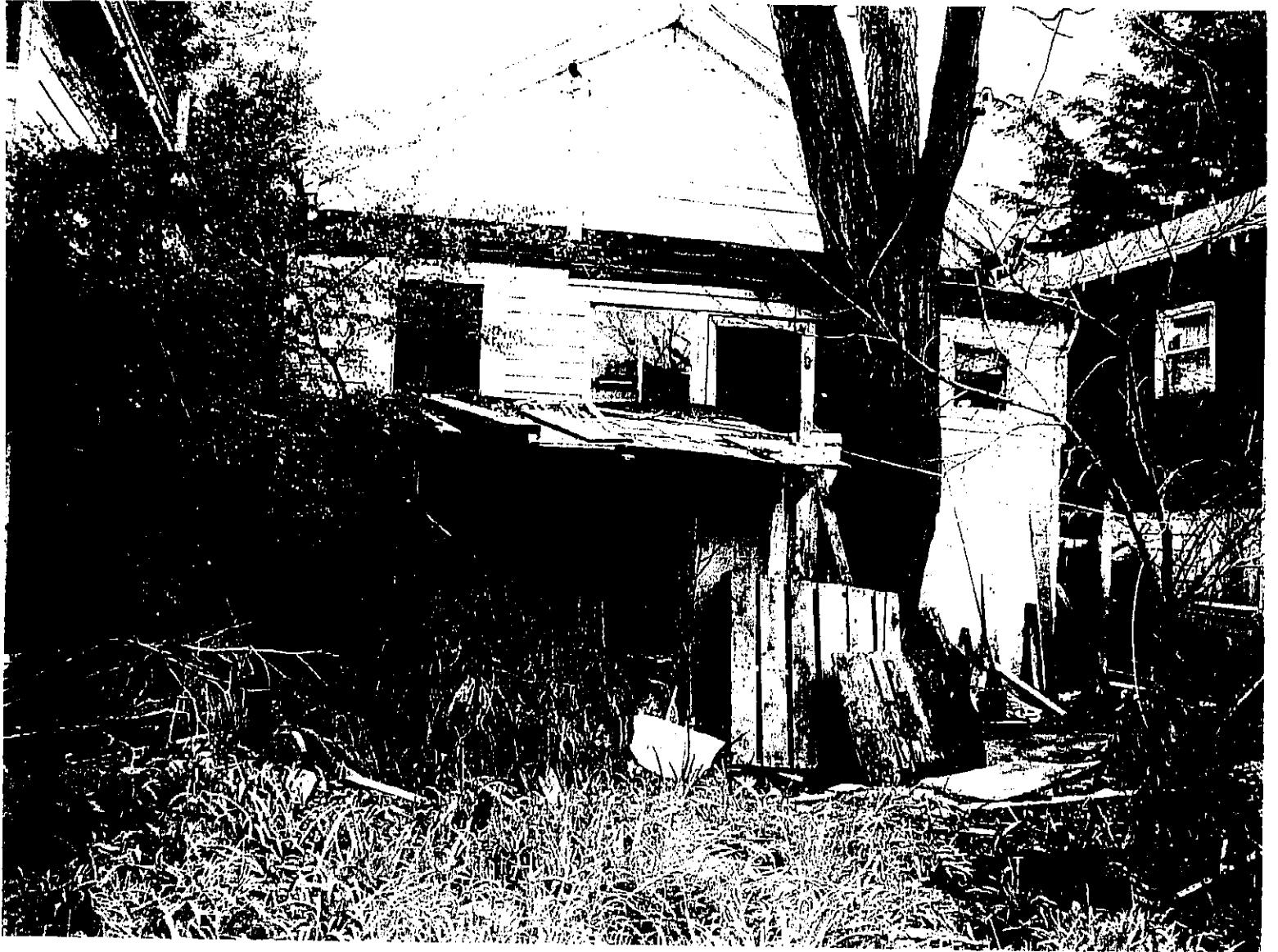
1081 41ST STREET - BACK OF BUILDING
