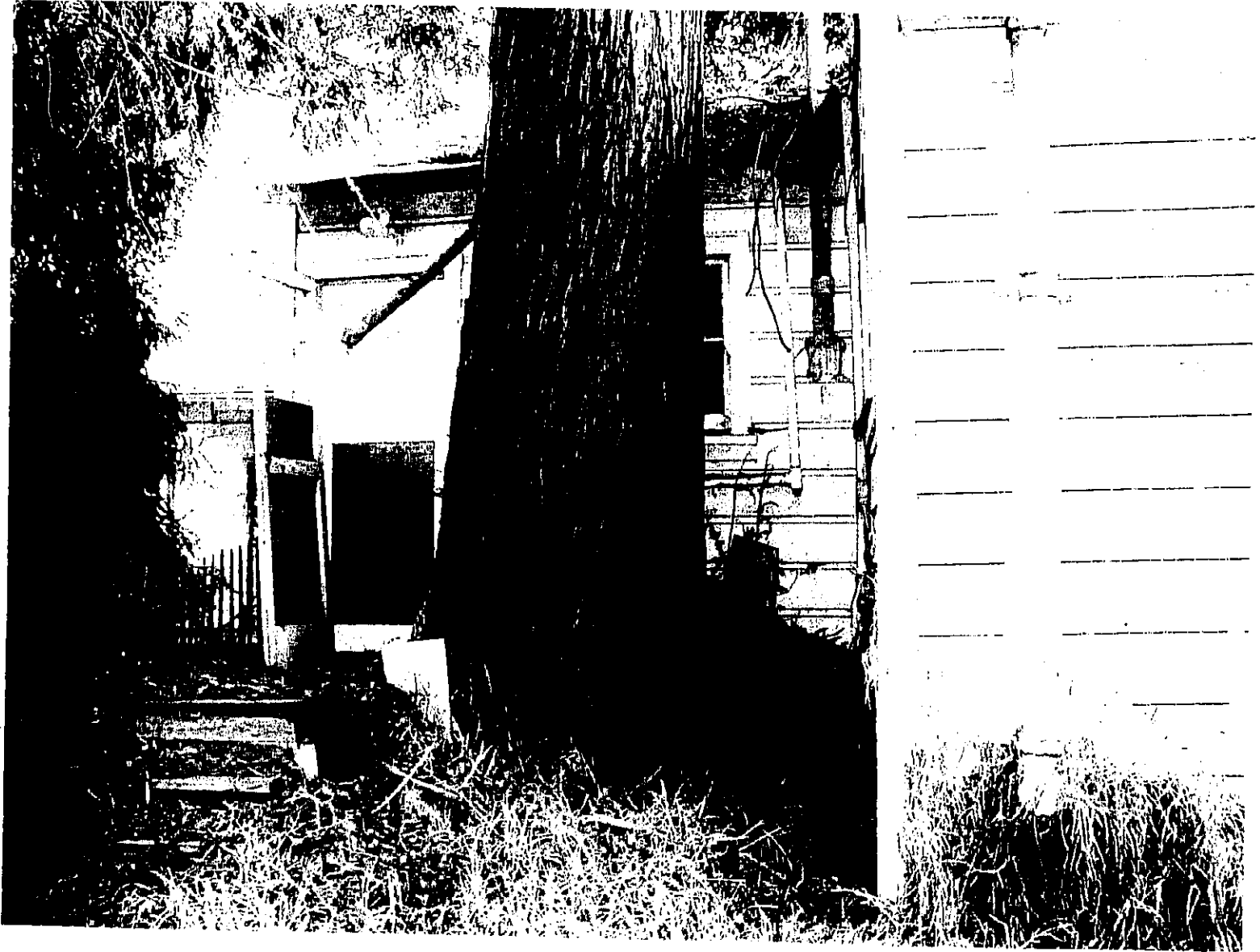
1085 41ST STREET - BACK OF BUILDING
