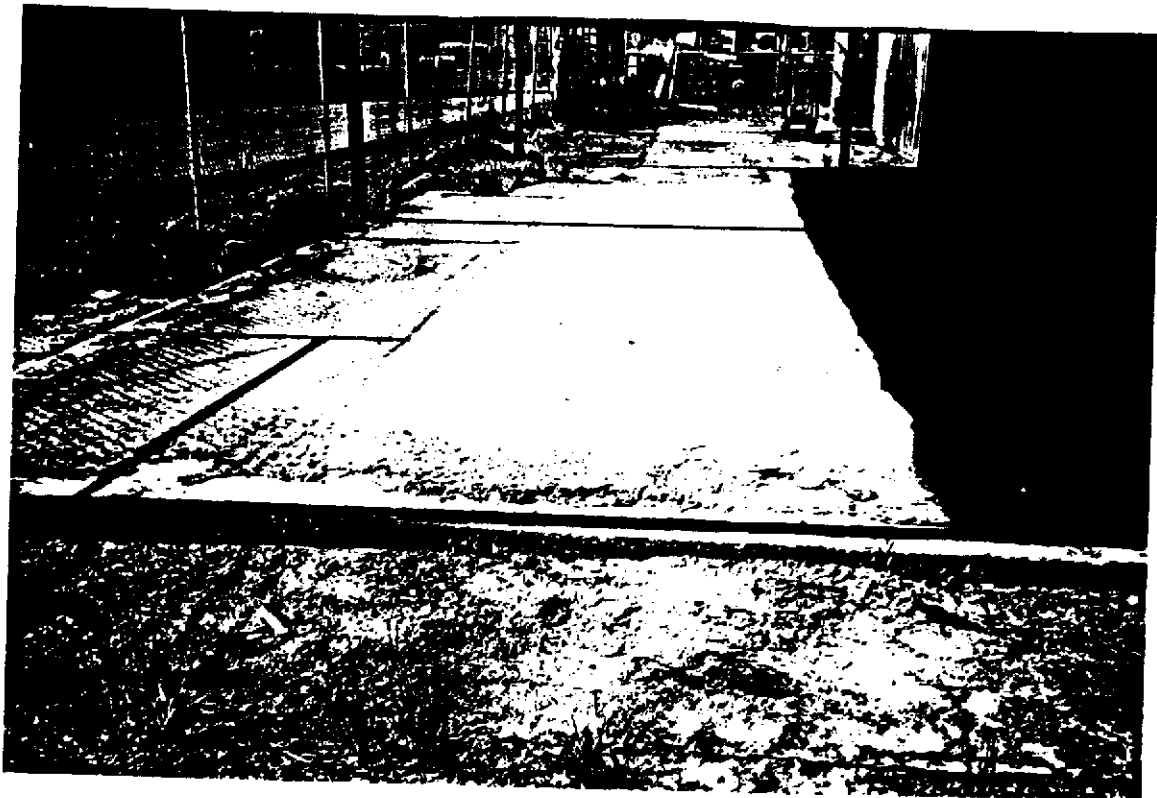
SOUTH CANOPY AREA LOOKING WEST
