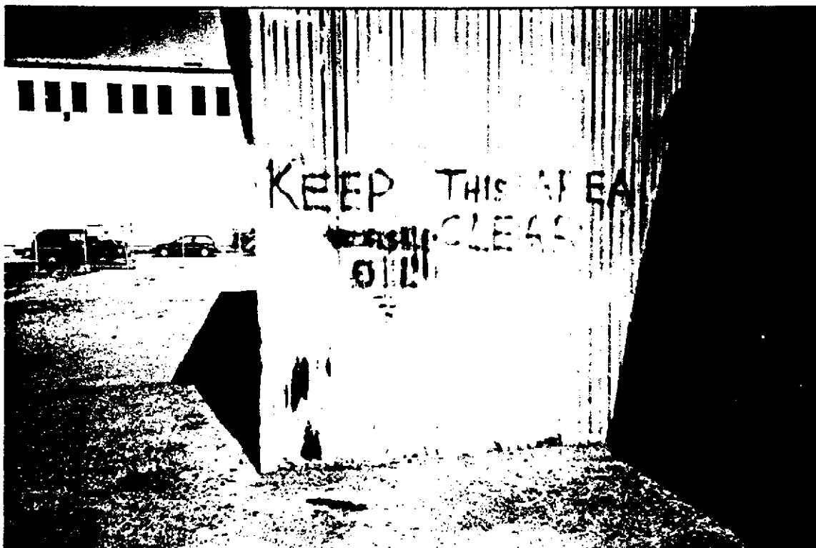
SOUTH WALL OF EAST CANOPY AREA FACING NORTH
