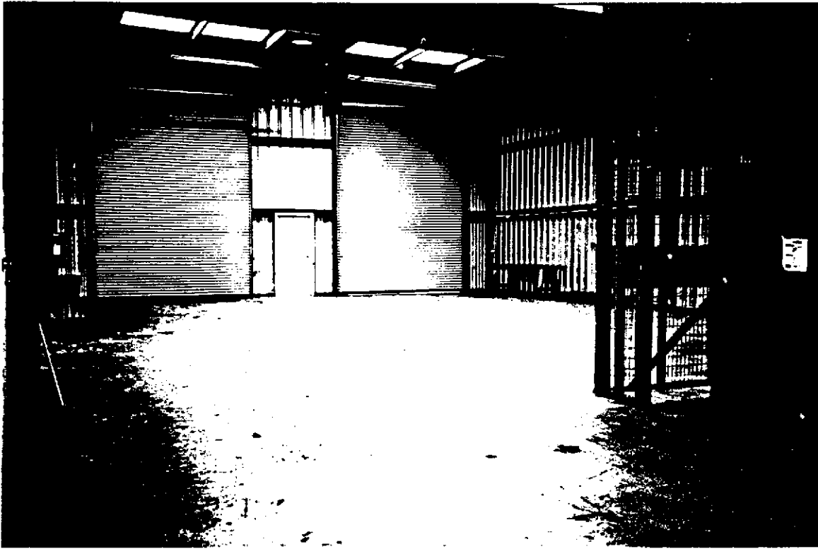
EASTERN BUILDING ADDITION LOOKING NORTH
