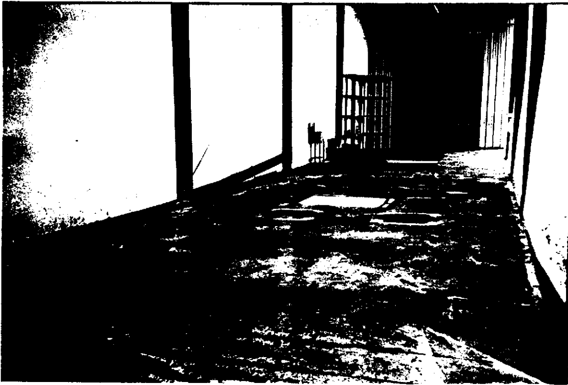
EAST CANOPY AREA LOOKING NORTH
