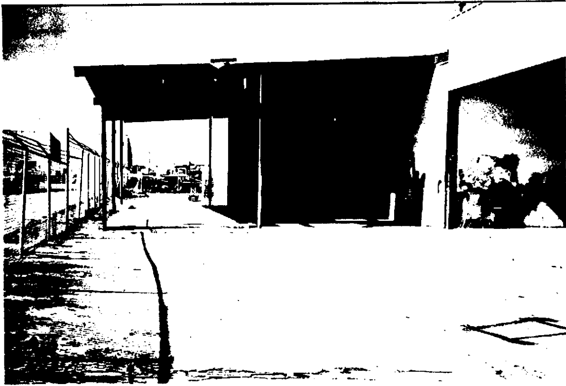
SOUTH SPRAY BOOTH AREA
