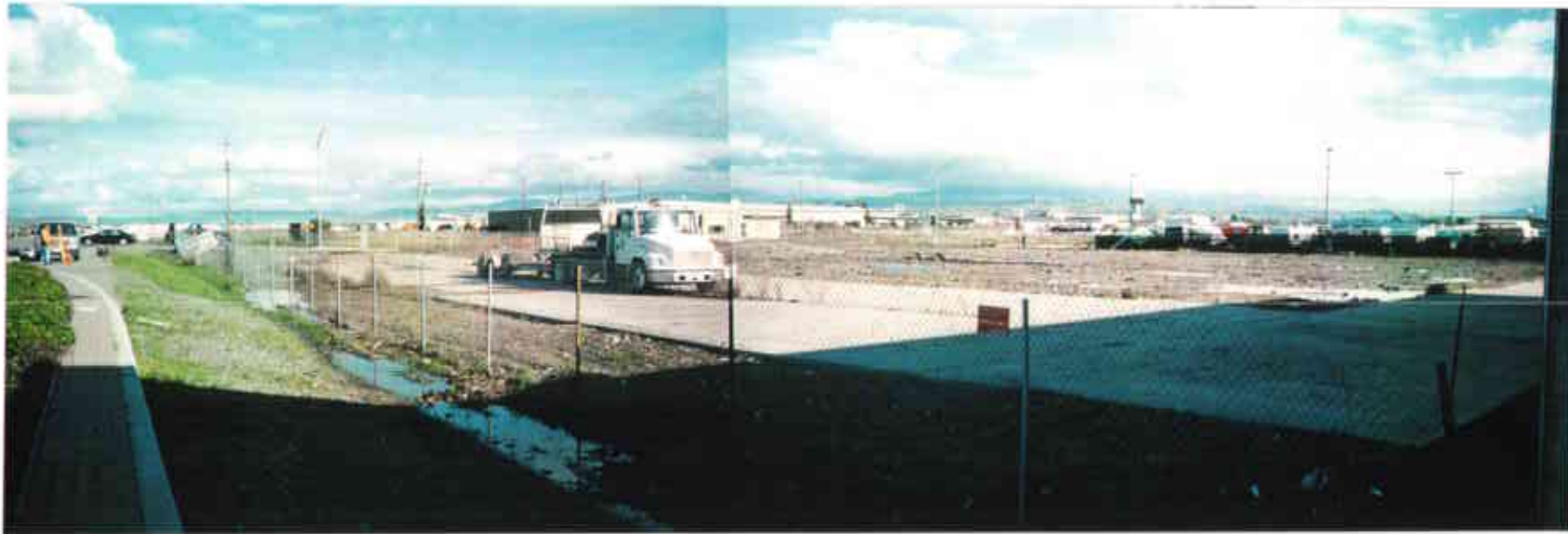
Photo 2. View across site from northwest corner.
