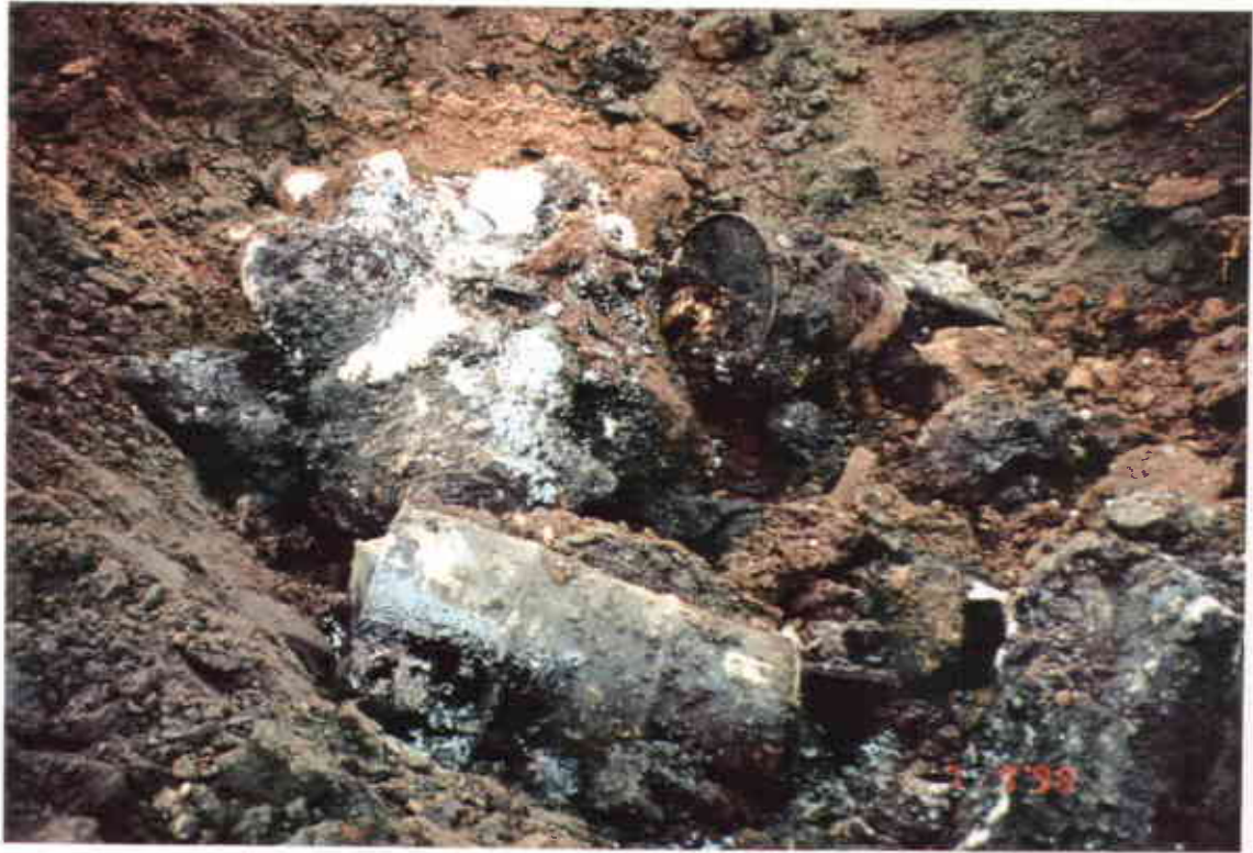
Photo 13: Buried drums and debris
