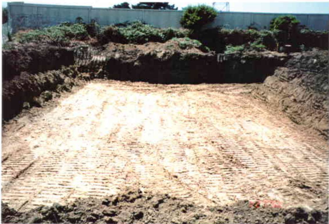
Photo 19: Roofing shingles trench in the southern portion of the Site
