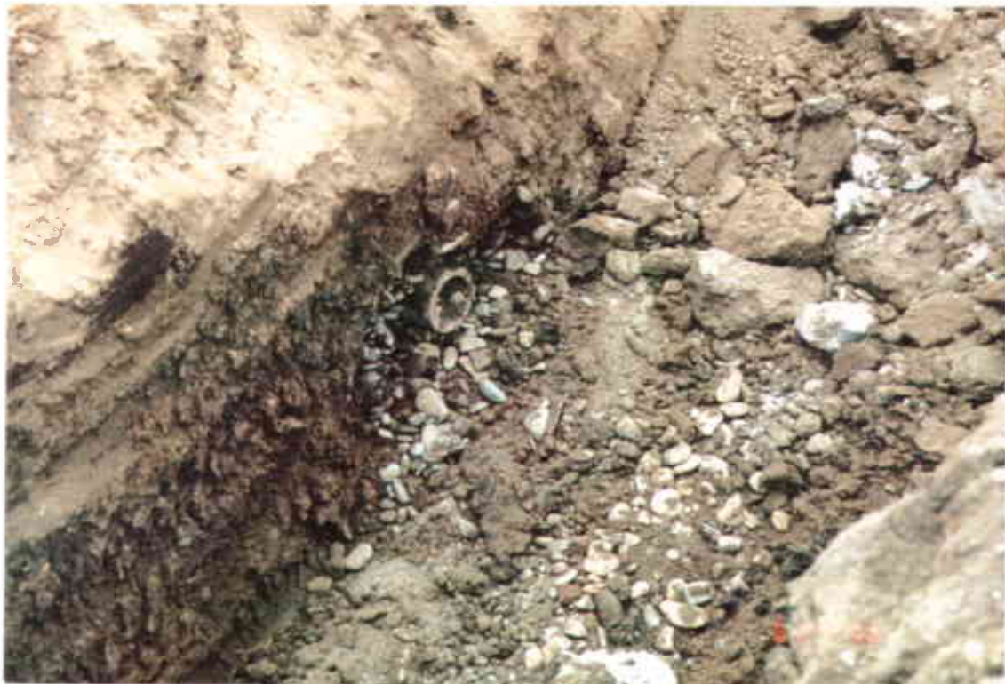
Photo 9: Sewer system leach field located to the west of the former concrete building pad
