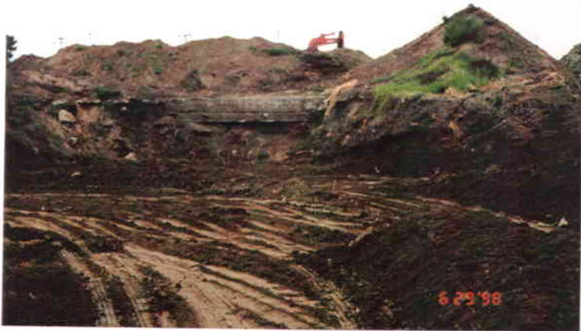
Photo 4: Concrete footings located at the northern boundary of the former excavation
