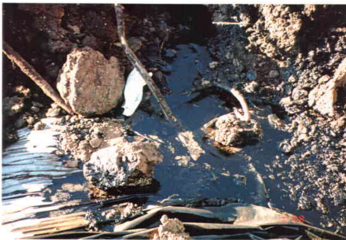
Photo 12: Tar material and product delivery pipes excavated from the subsurface
