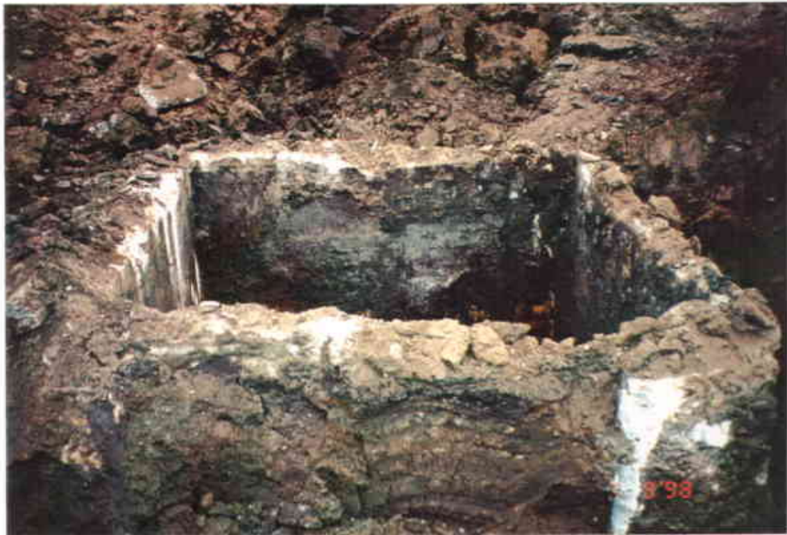
Photo 5: Concrete vault located at the northern boundary of the former excavation
