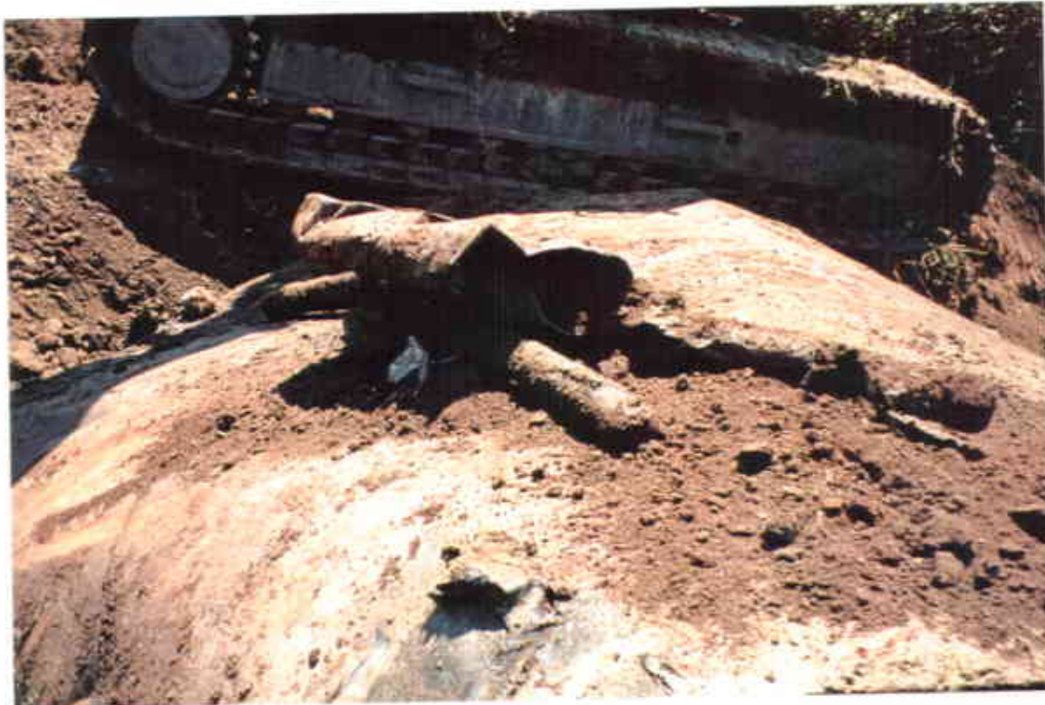
Photo 11: Top of former cistern located in the southwestern corner of Site
