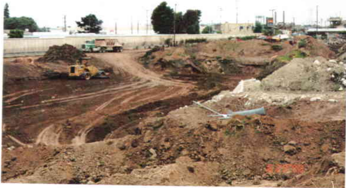
Photo 3: Northern portion of the excavation pit
