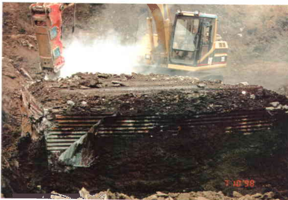
Photo 8: Concrete footings located at the northern boundary of the former excavation
