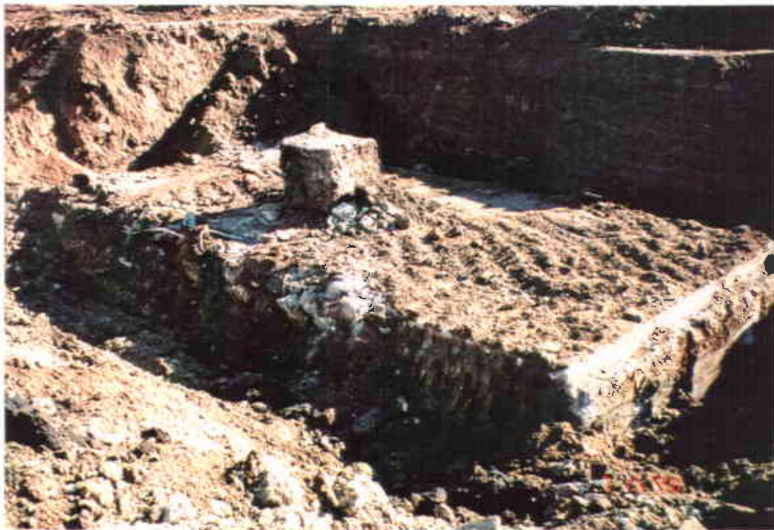
Photo 7: Concrete footings located at the northern boundary of the former excavation
