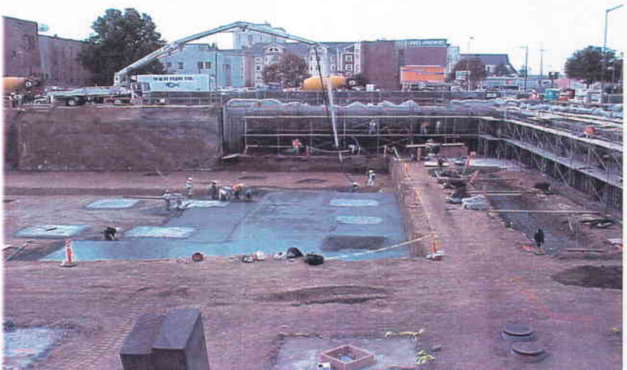
Photo 4 – Final Excavation Depth With Initial Foundation Work (southwest corner)
