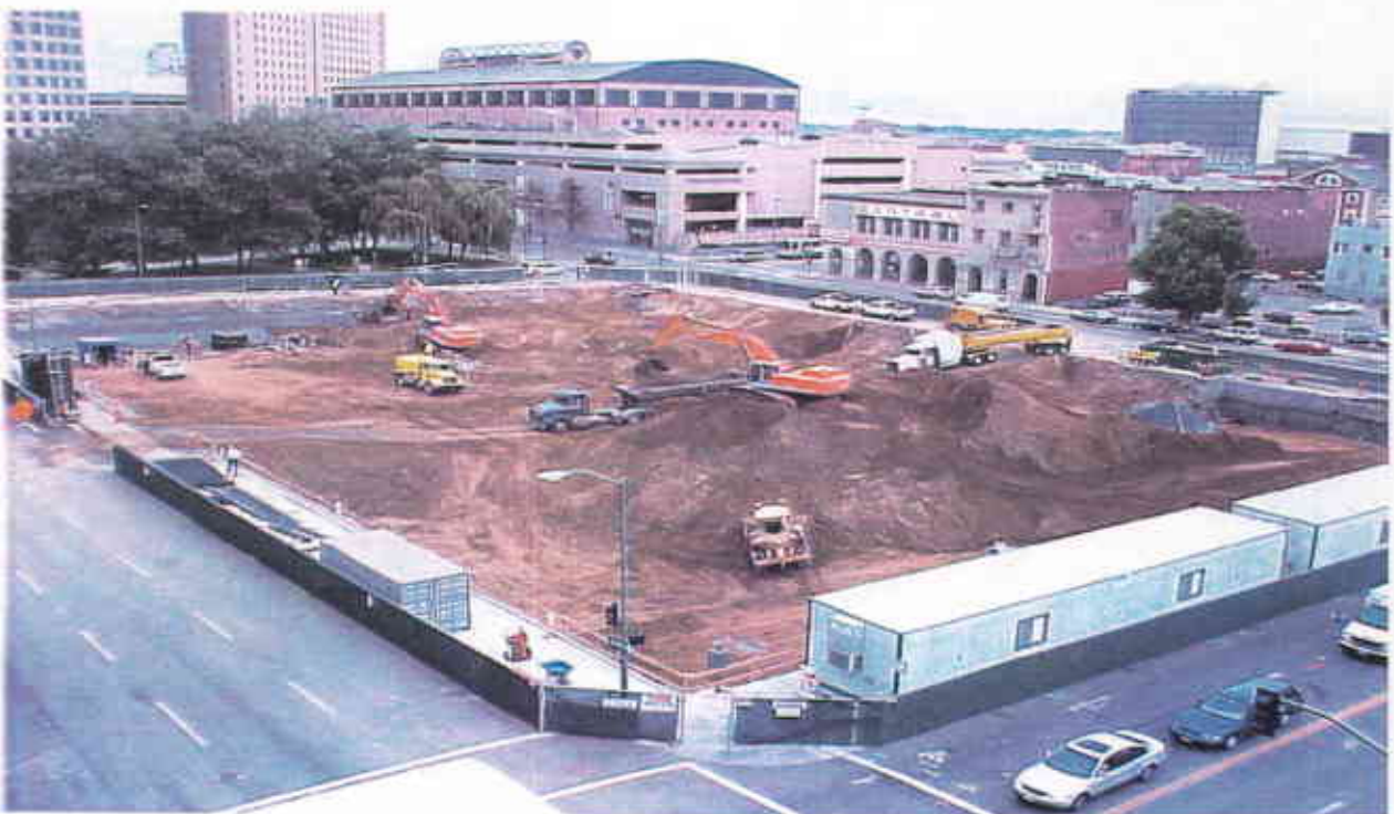
Photo 2 – Excavation Work in Progress (Hydrocarbon Impacted Soil Located Underneath Plastic Sheetting)
