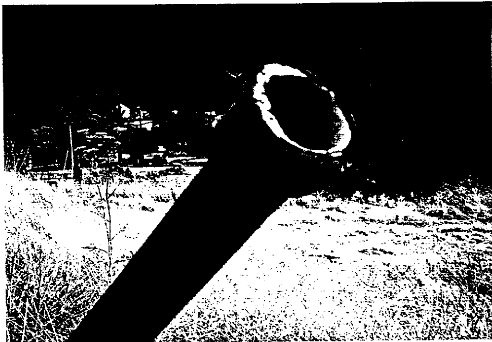
Photograph 3. Looking at the top of the east end of the tank. The 4-inch cast iron pipe has slip connections on each end of the pipe elbow.
