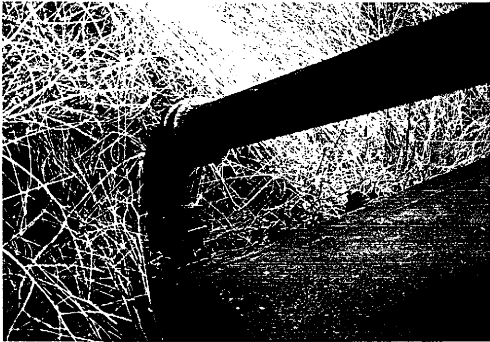
Photograph 3. Looking at the top of the east end of the tank. The 4-inch cast iron pipe has slip connections on each end of the pipe elbow.
