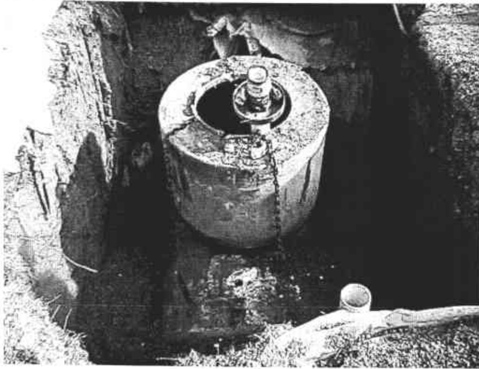
Tank in Excavation; Ready for Removal
