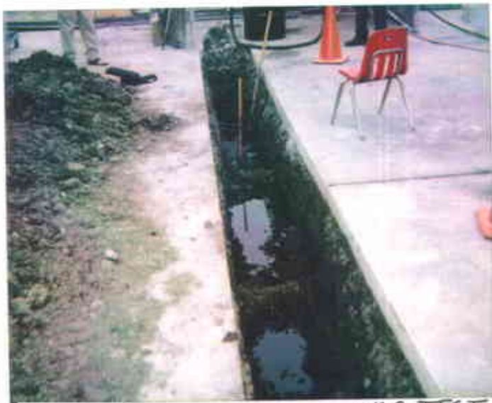
FREE PRODUCT IN TRENCH - NAC TEST 10/1/98 3:40P.M. - DH FACILITY
