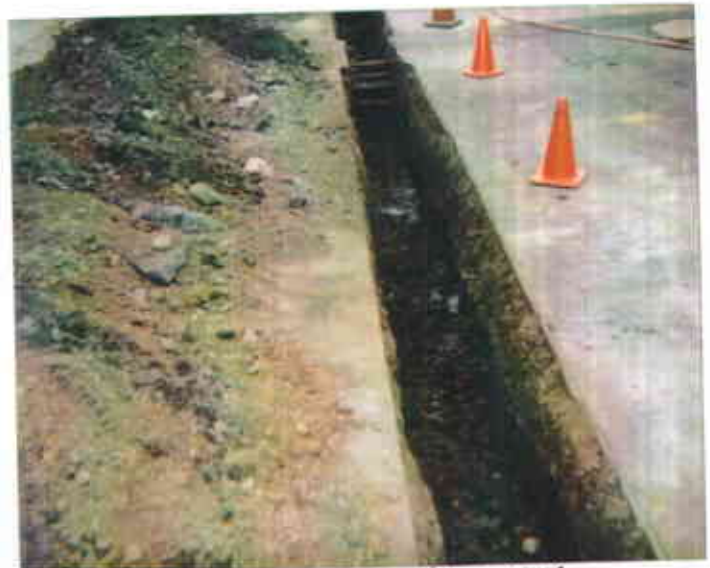
TRENCH - NAC TEST FACILITY 10/1/98 3:45P.M. - D. HERMAN
