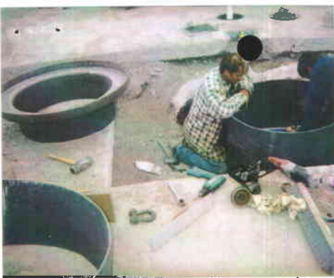
RETROFIT OF EXISTING 10K-GALON VST NAC FACILITY - TEST CENTER 10/1/98 3:50P.M. - D. HERMAN
