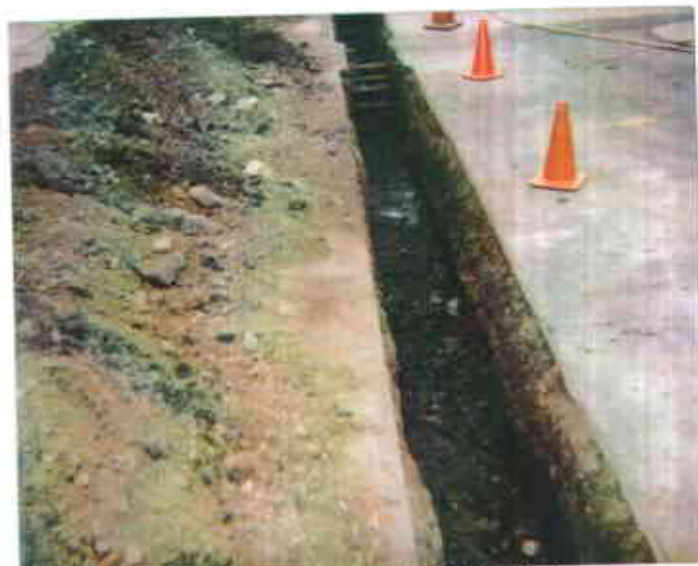
TRENCH - NAC TEST FACILITY 10/1/98 3:45P.M. - DHERMAN
