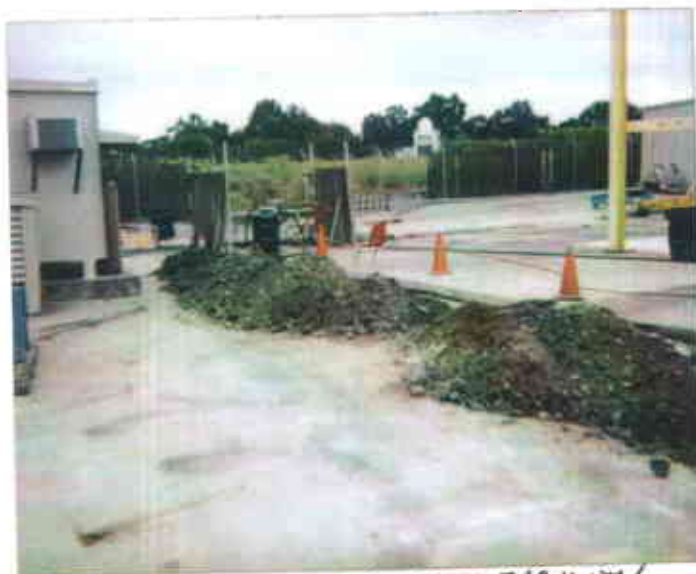
TRENCH SPOILS NAC TEST FACILITY 10/1/98 3:45P.M. - D. HERMAN
