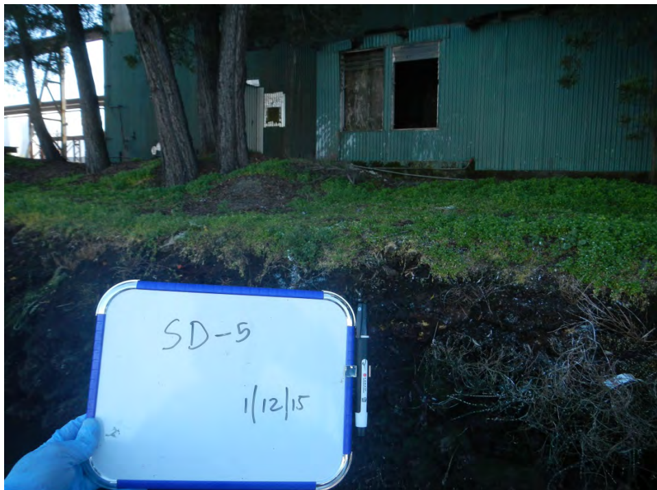
Photograph 28. SD-5 Location (January 12, 2015)
