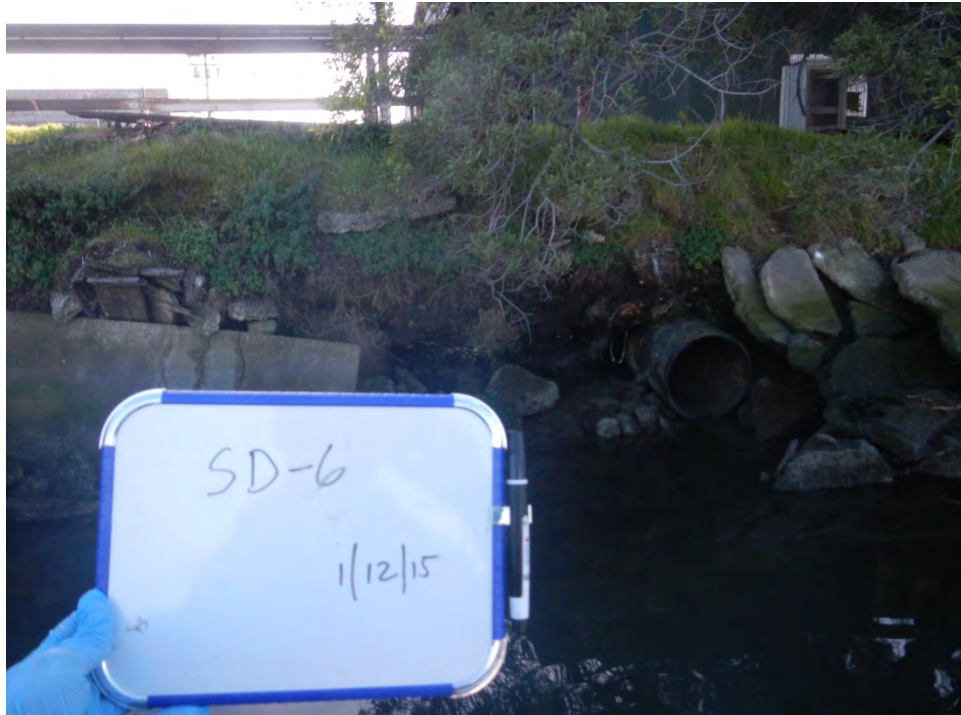
Photograph 31. SD-6 Location (January 12, 2015)
