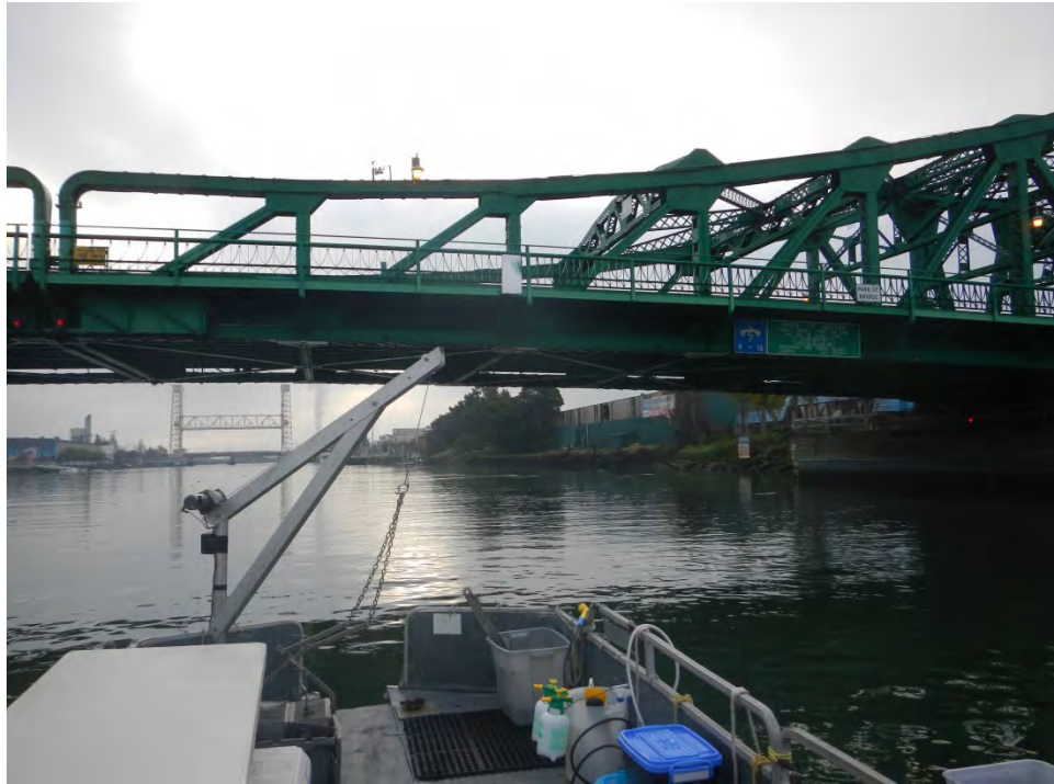
Photograph 3. Site Approach with Bridge (January 12, 2015)
