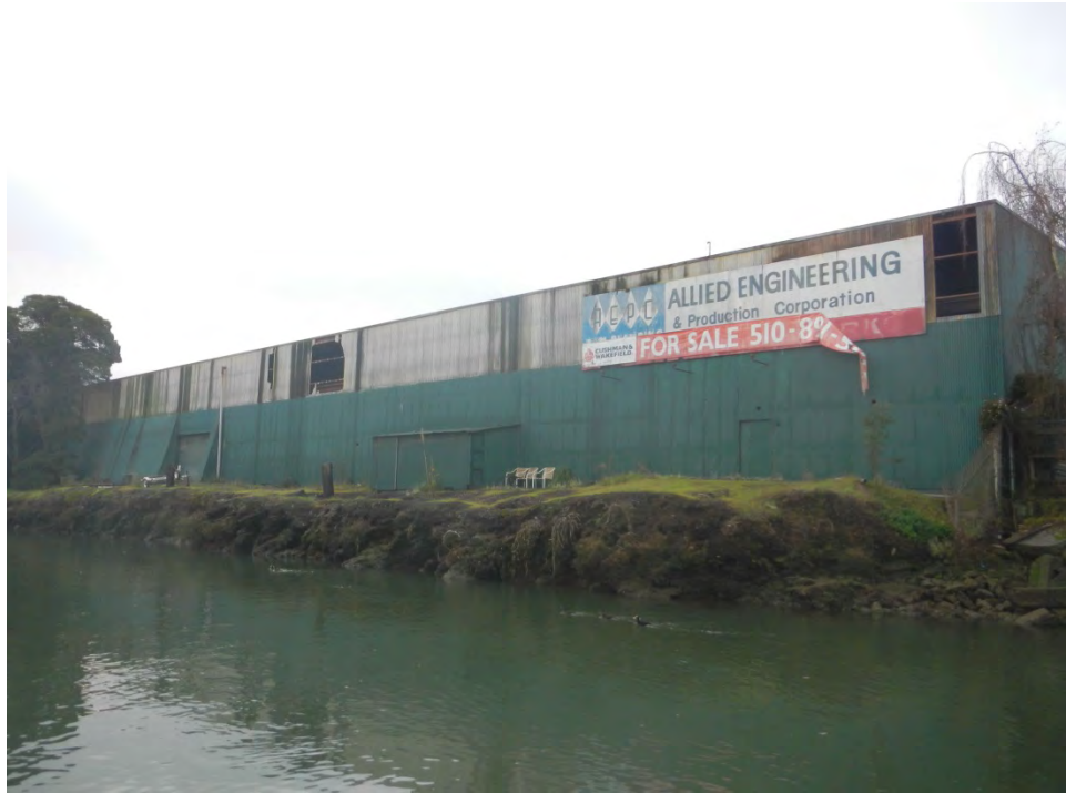
Photograph 5. Western Portion of Site Approaching SD-1 (January 12, 2015)
