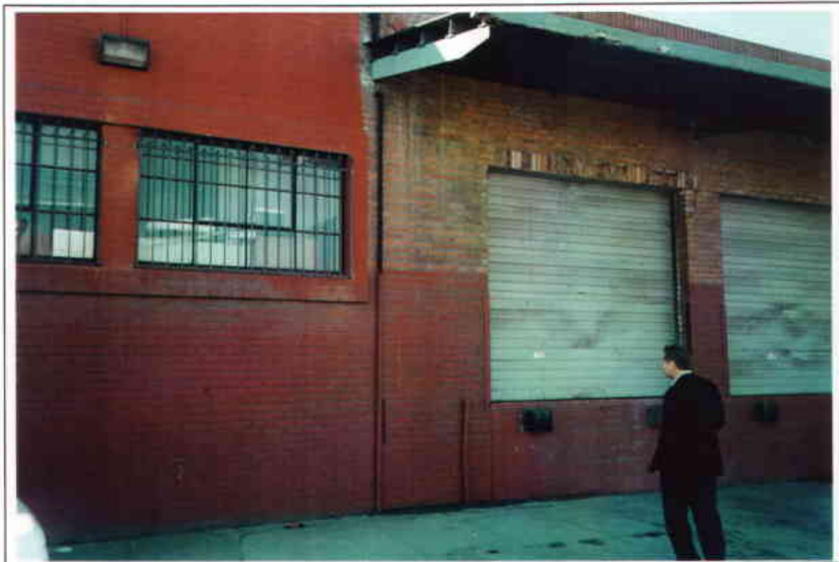
Photo 4: View of vent pipe located on the north side of the warehouse of Thai Kitchen.
