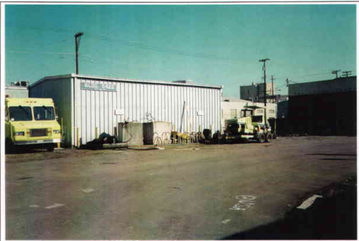
Photo 14: View to the northeast of Building E422.
