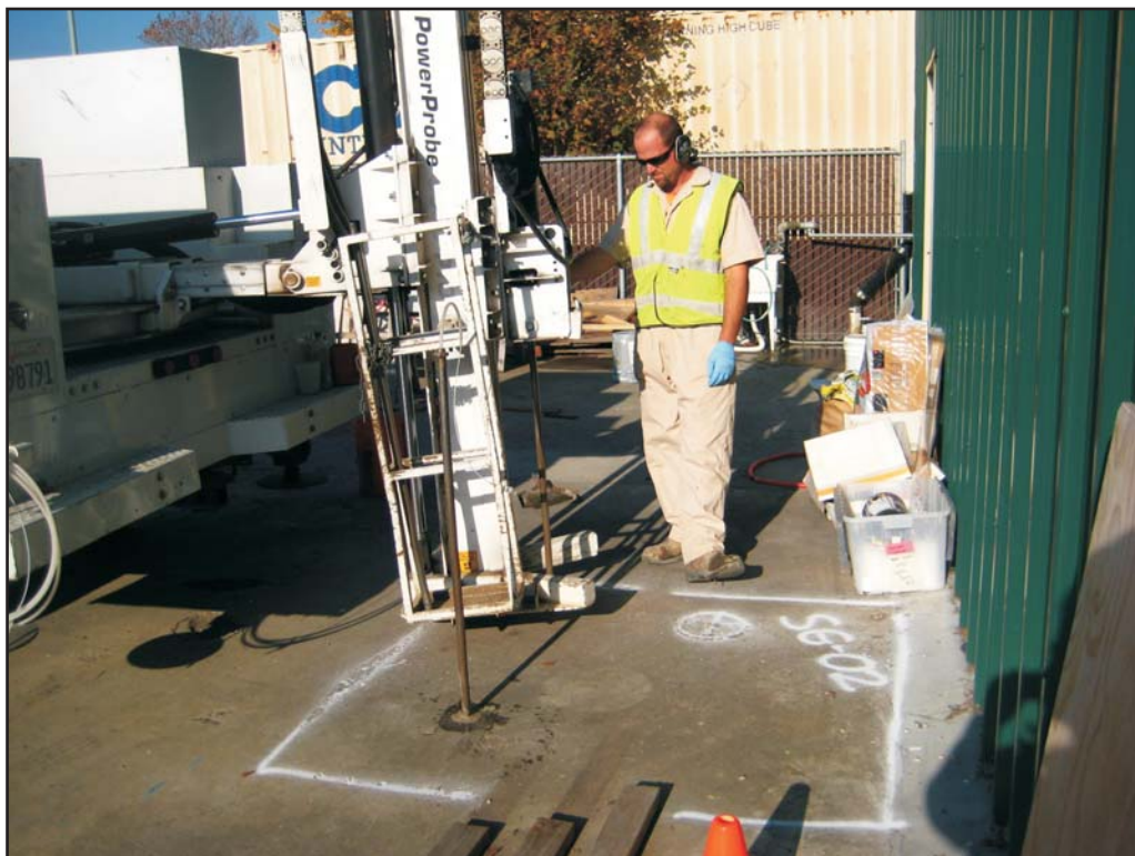
Photograph 28: TEG installing deep probe at SG-02.
