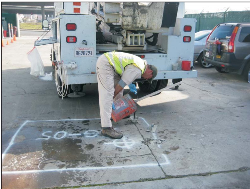
Photograph 16: TEG grouting of deep boring at SG-05.
