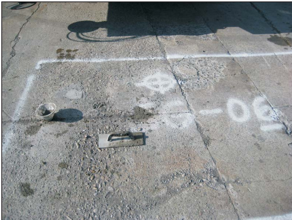
Photograph 21: Abandonment of boreholes at SG-06.
