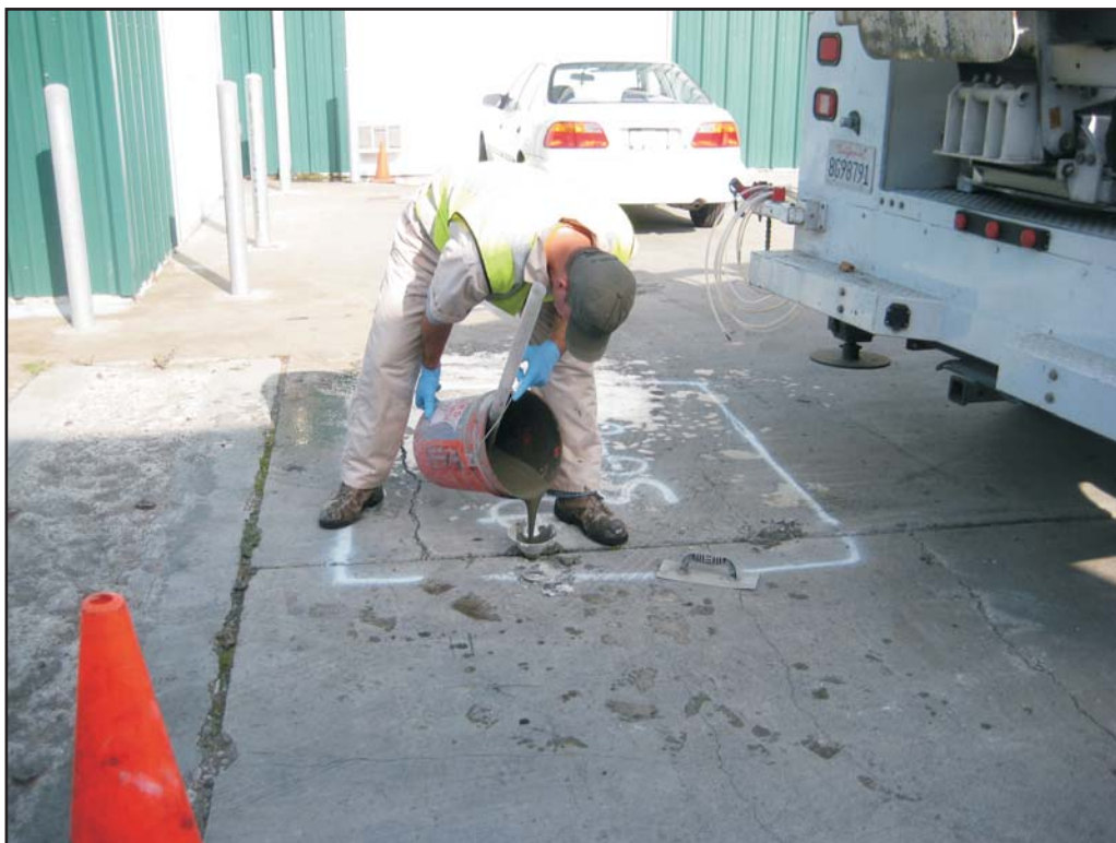
Photograph 17: TEG grouting of shallow boring at SG-05.
