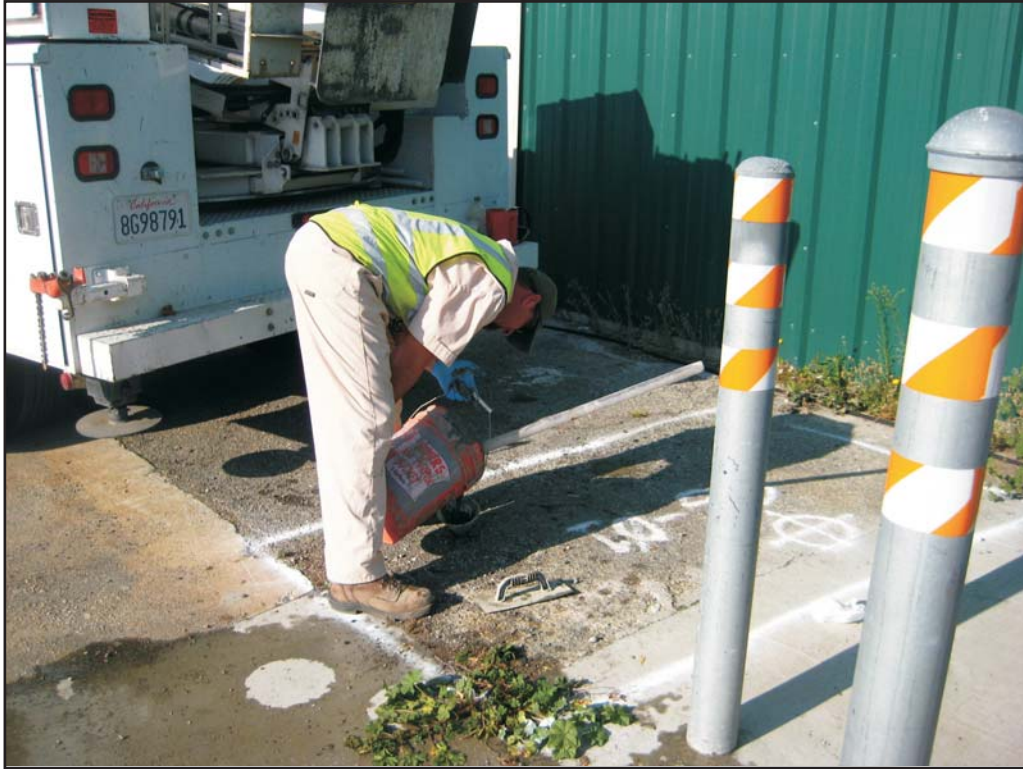
Photograph 25: TEG abandoning of boreholes at SG-01.
