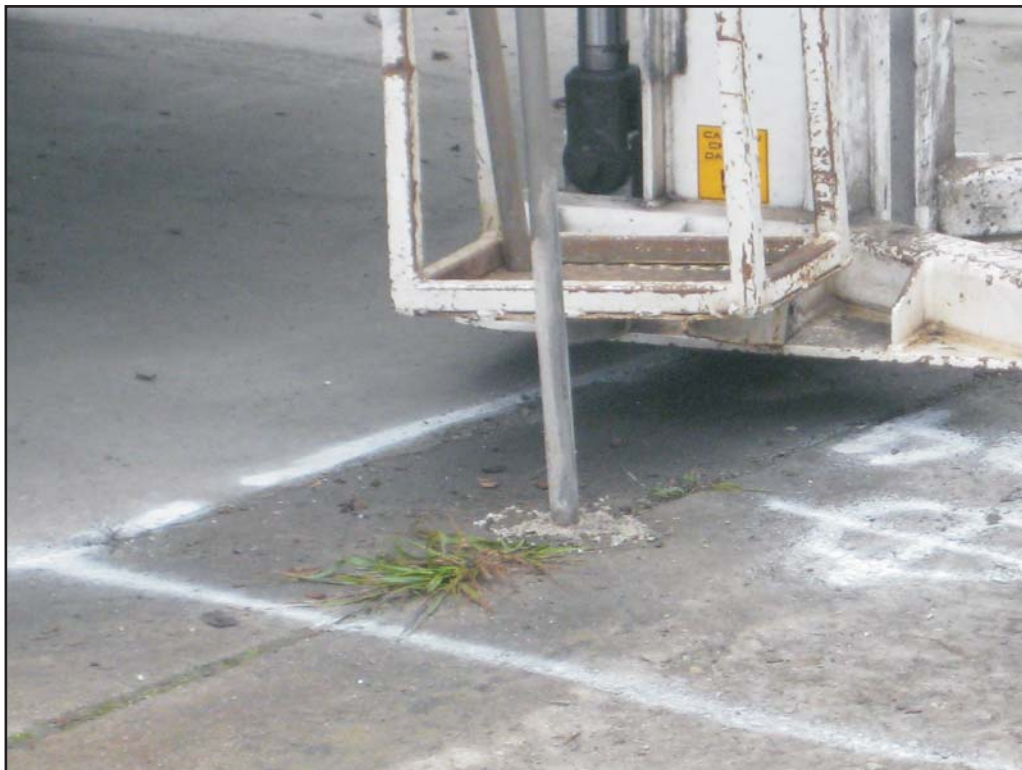
Photograph 5: Bentonite seal at ground surface at SG-04.
