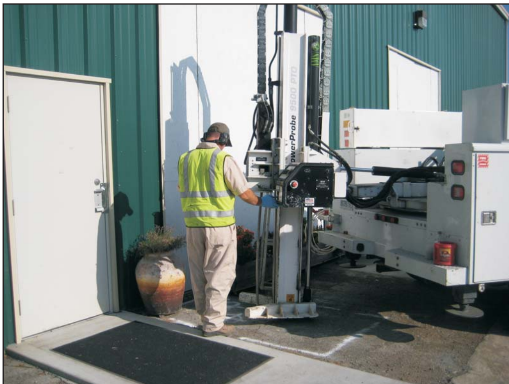
Photograph 22: TEG installing shallow probe at SG-03.
