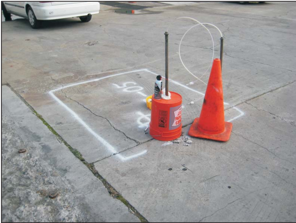
Photograph 11: Leak test at shallow probe at SG-05.
