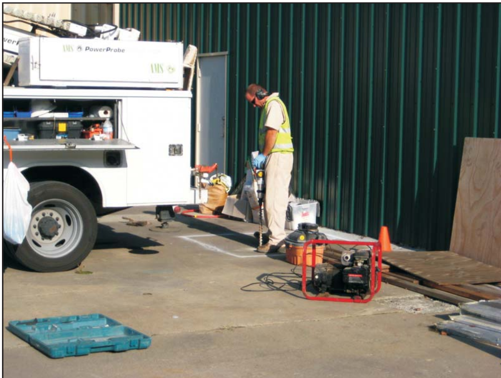
Photograph 26: TEG coring through pavement at SG-02.
