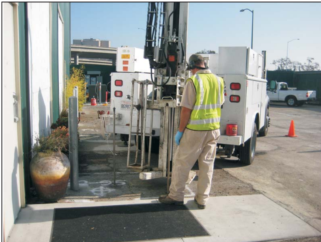
Photograph 23: TEG installing deep probe at SG-03.
