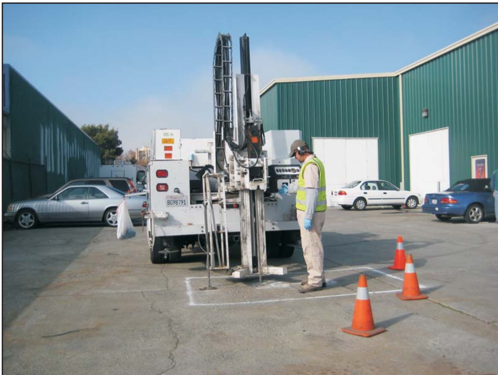
Photograph 13: TEG installing deep probe at SG-06.
