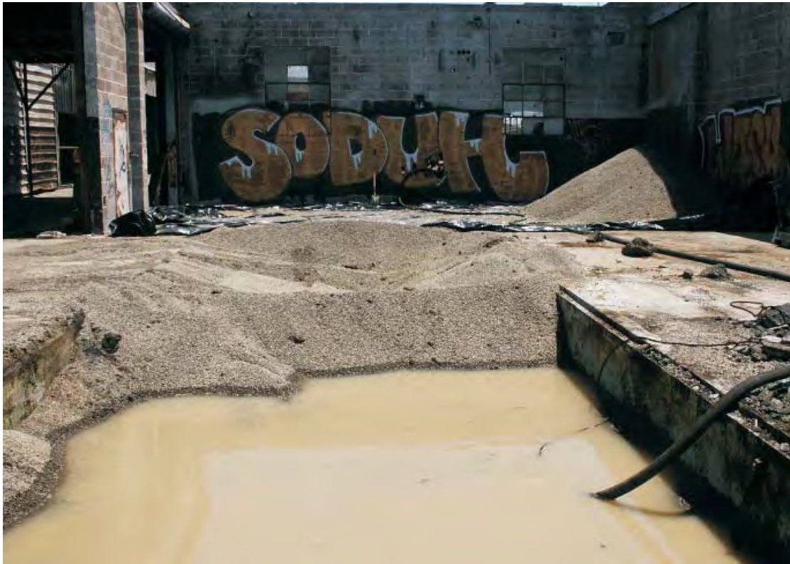
Photo 3: Pea gravel and water in Frog Pond (water being pumped to Baker Tank).
