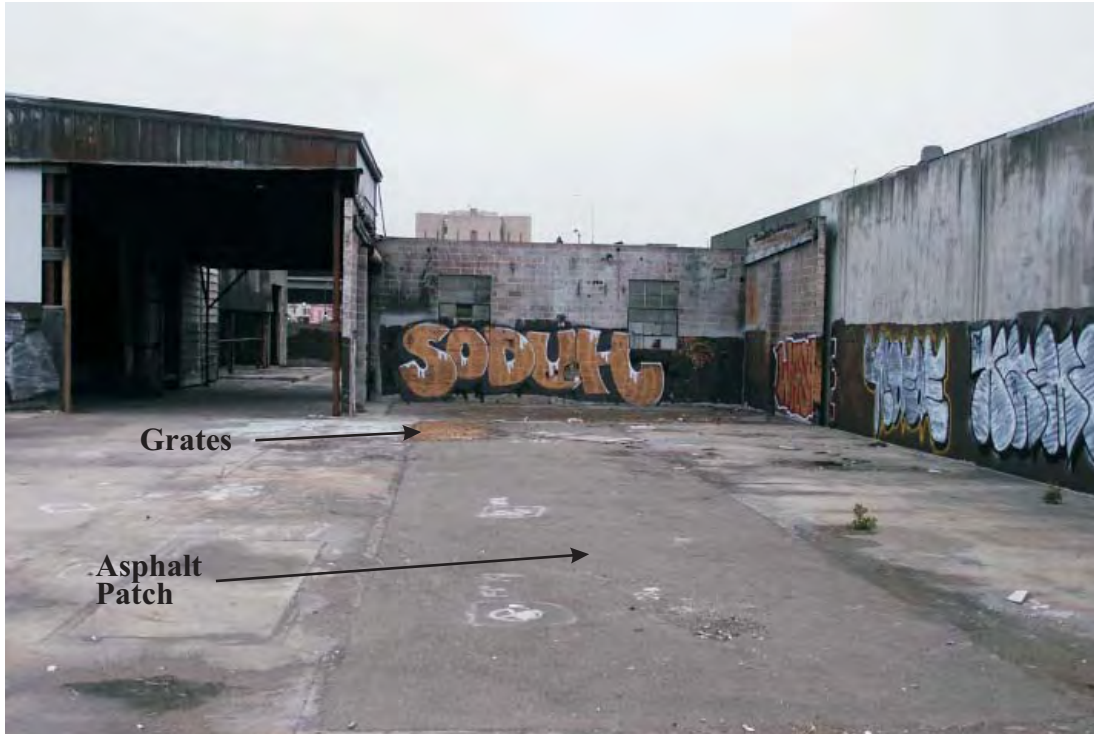
Photo 1: Asphalt patch showing outline of Frog Pond.
