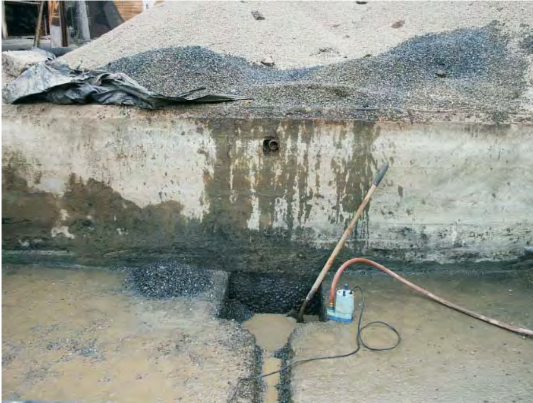
Photo 5: Eastern Sump and PVC pipe penetrating sidewall.
