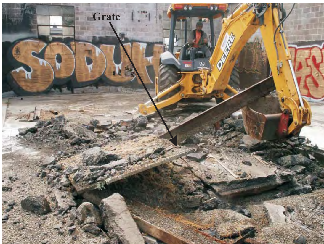
Photo 2: Grates and I-beams being removed at northeastern corner of Frog Pond.
