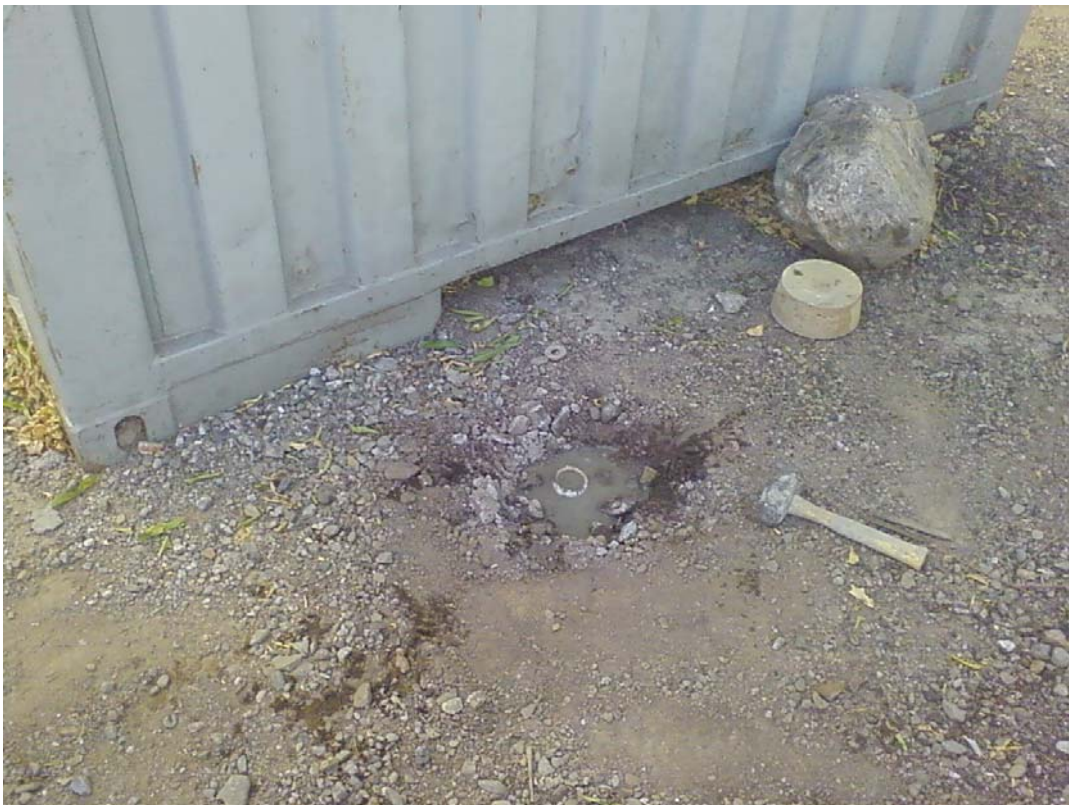
Plate 8. View of MW-2 after pressure grouting
