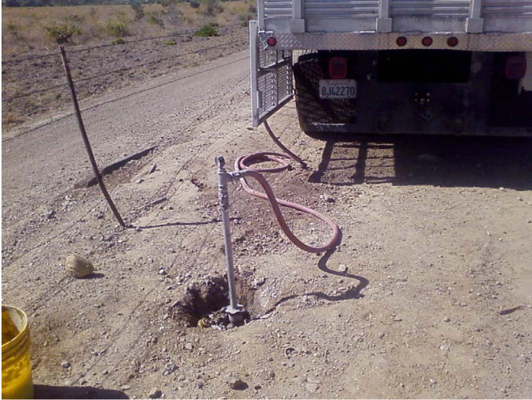
Plate 13. View of MWS-2 during pressure grouting
