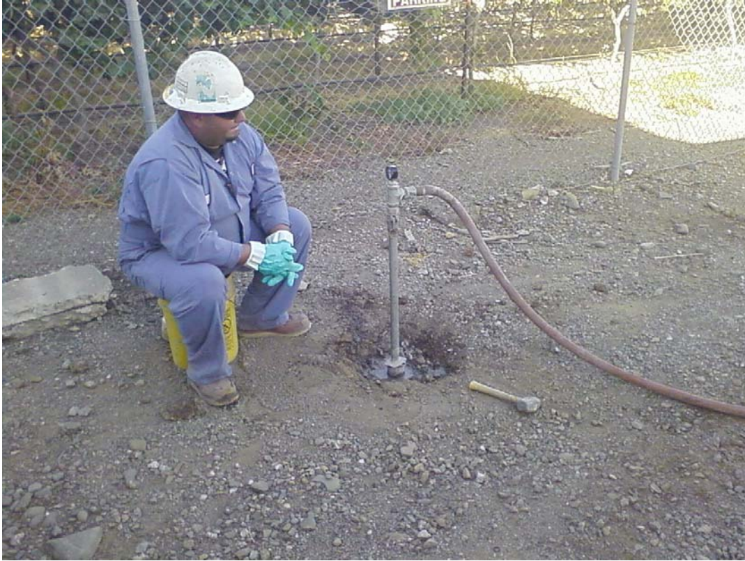
Plate 1. View of MW-1 during pressure grouting
