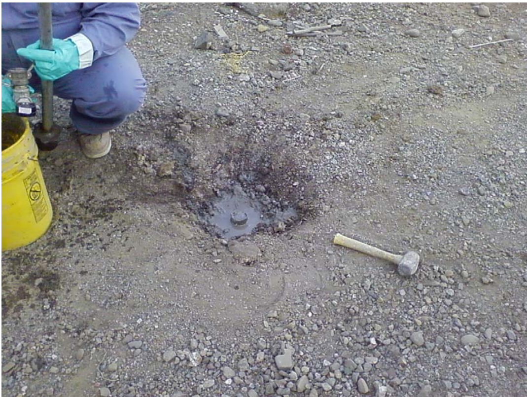
Plate 2. View of MW-1 after pressure grouting
