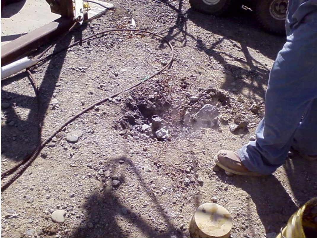
Plate 11. View of MWS-1 after pressure grouting
