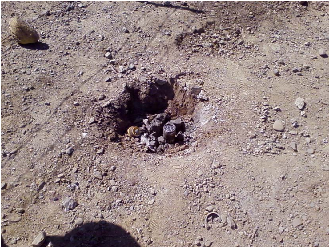
Plate 14. View of MWS-2 after pressure grouting
