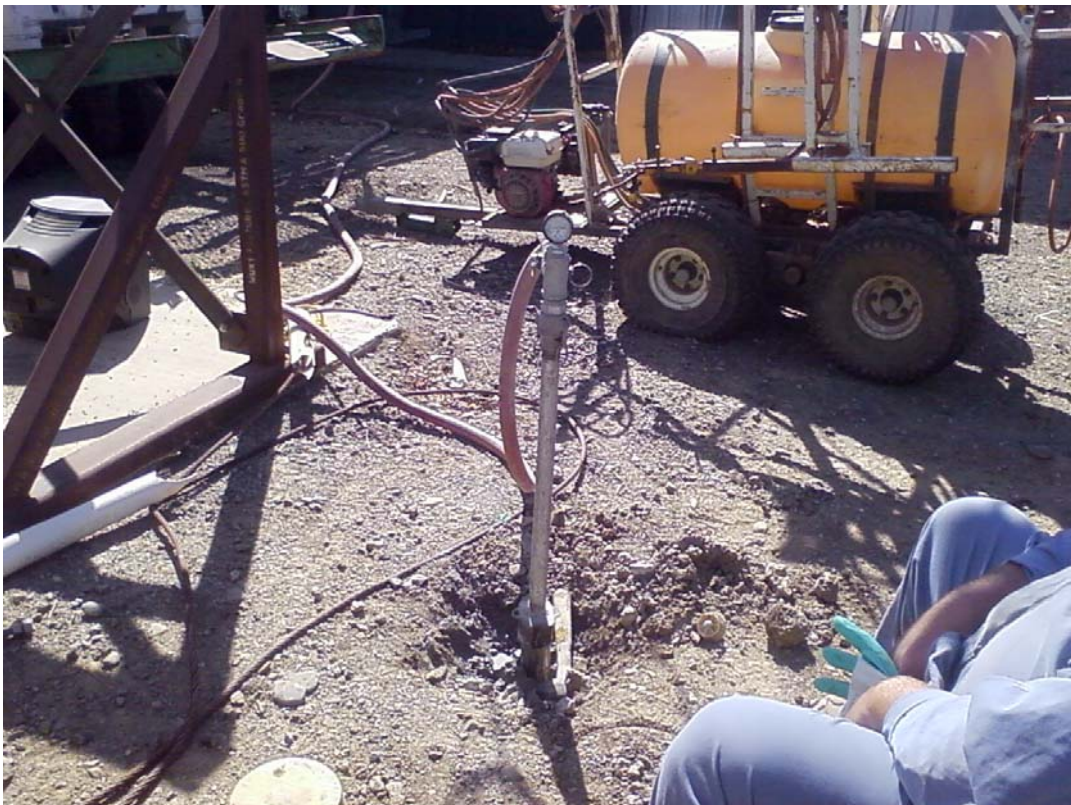
Plate 10. View of MWS-1 during pressure grouting
