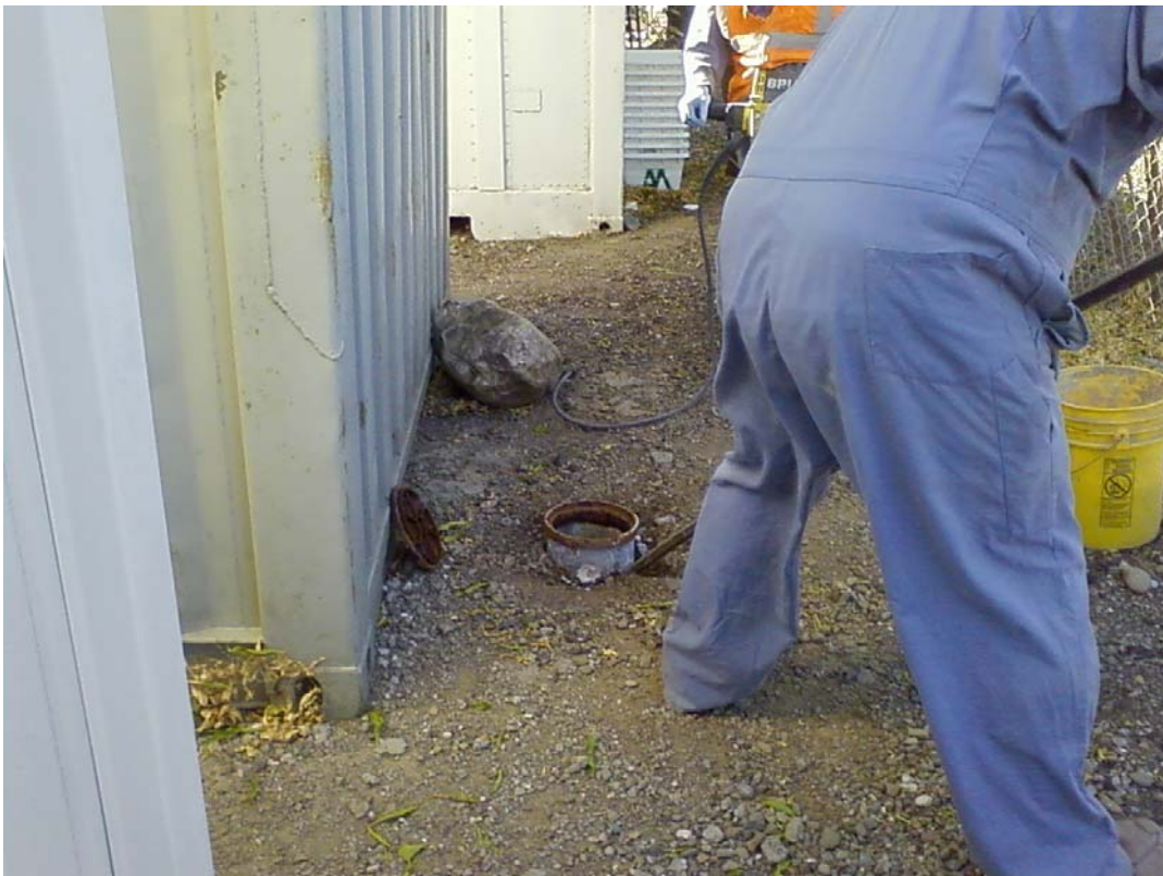
Plate 6. View of well box removal from MW-2
