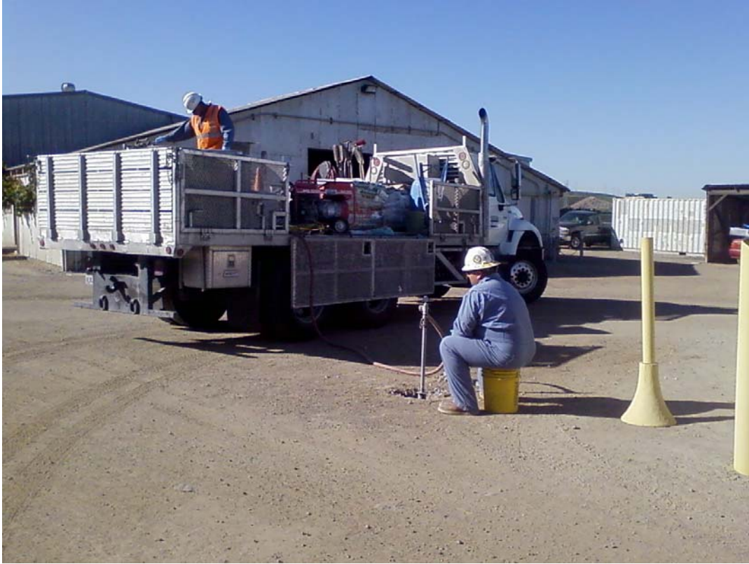
Plate 3. View of MW-3 during pressure grouting
