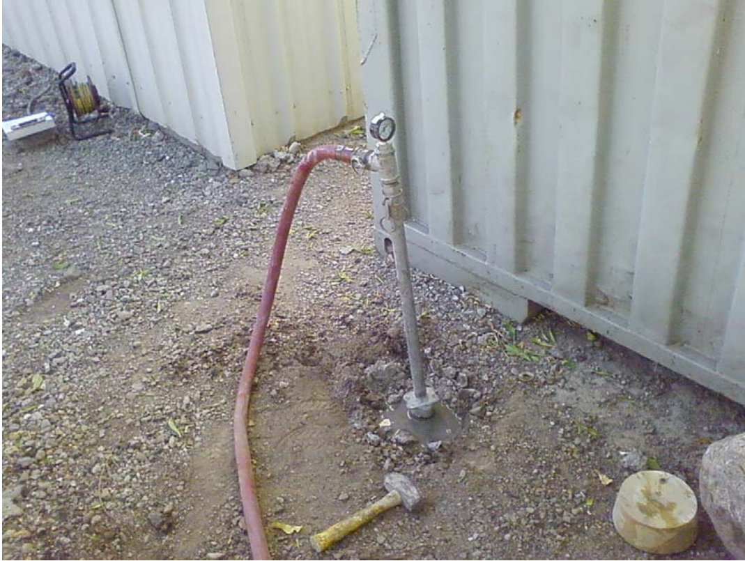
Plate 7. View of MW-2 during pressure grouting
