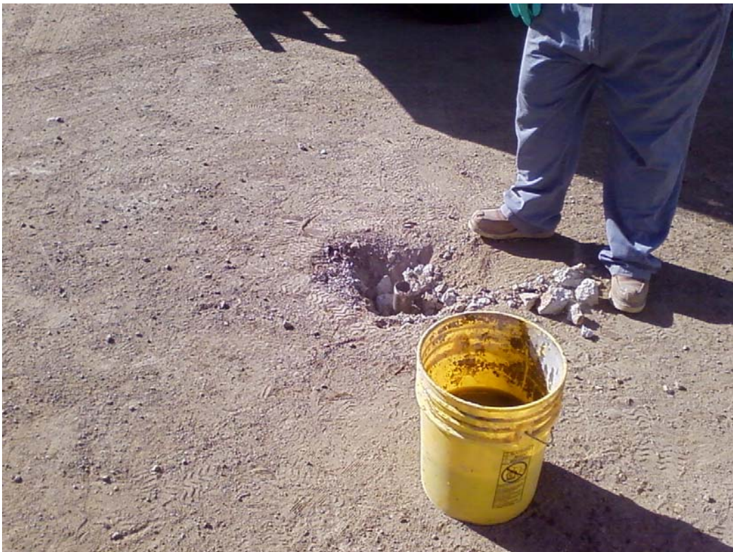
Plate 4. View of MW-3 after pressure grouting
