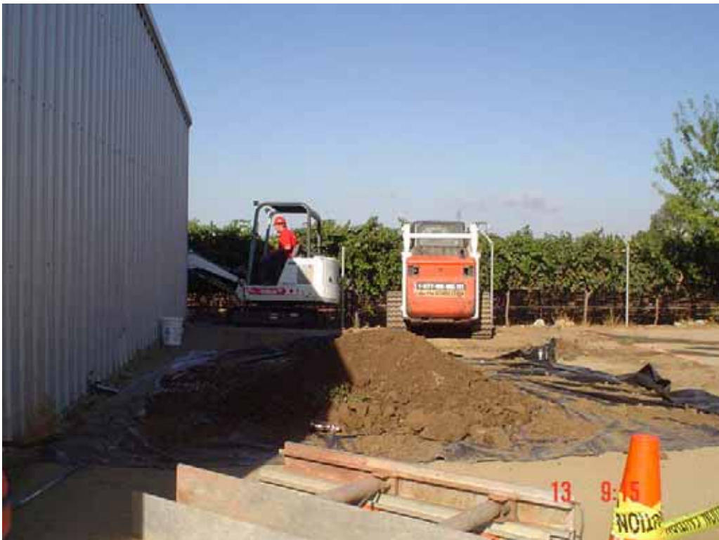
Plastic Sheeting beneath Each Stockpile
