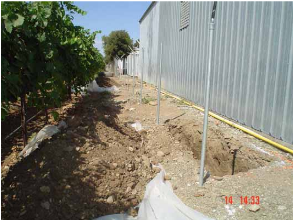
Excavation Areas 2 and 3(View North)
