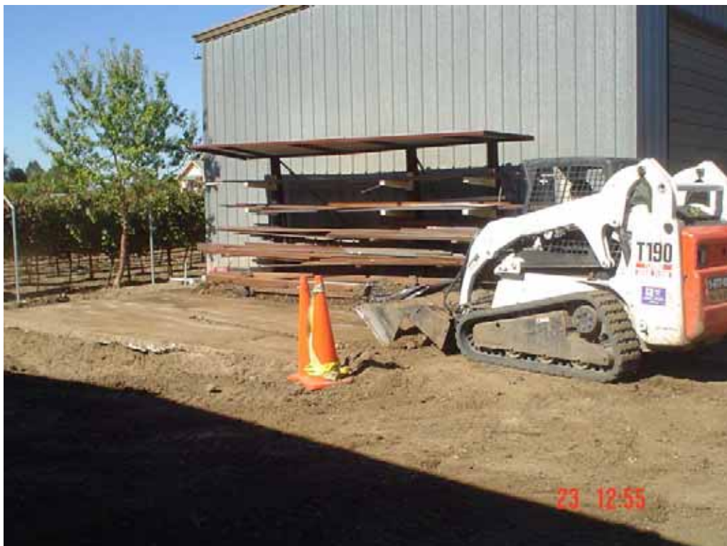
Cleaning the Excavation and Stockpile Areas
