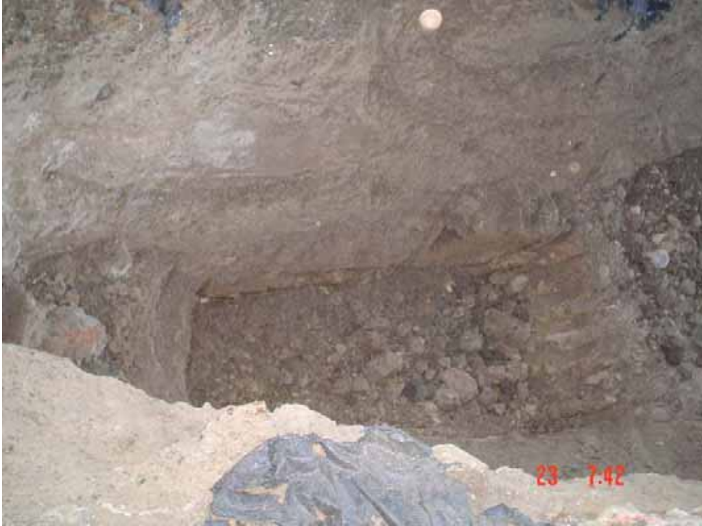
Eastern Portion of Area 4 (Second Excavation Phase)
