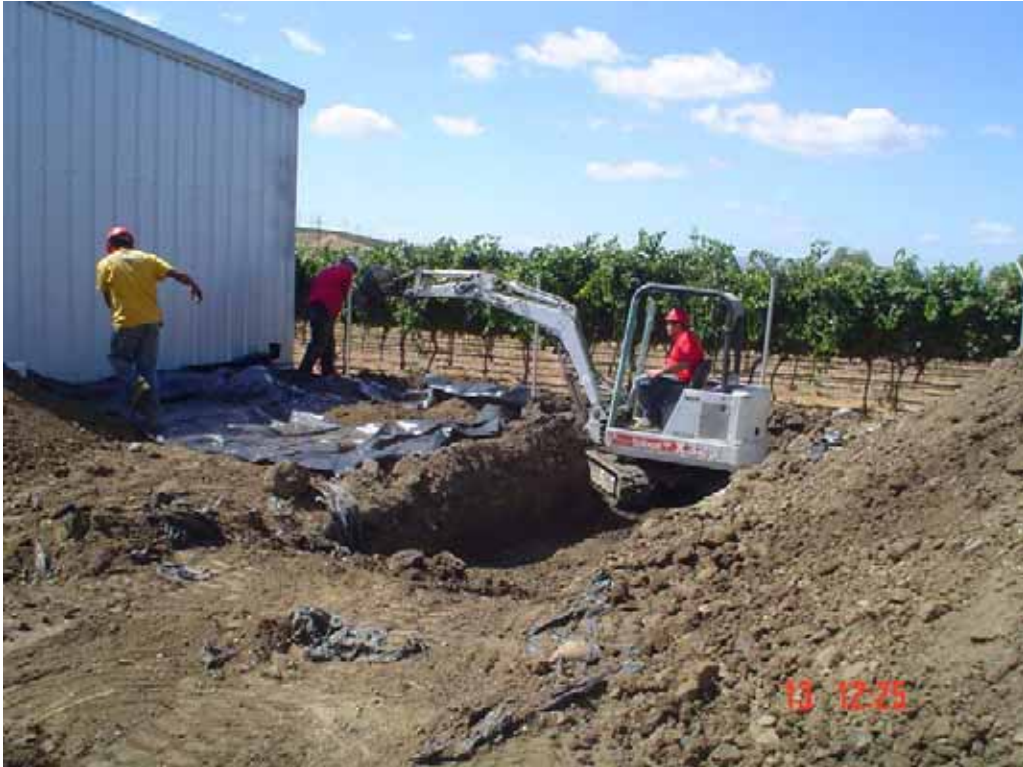
Excavation of Southern Portion of Area 4
