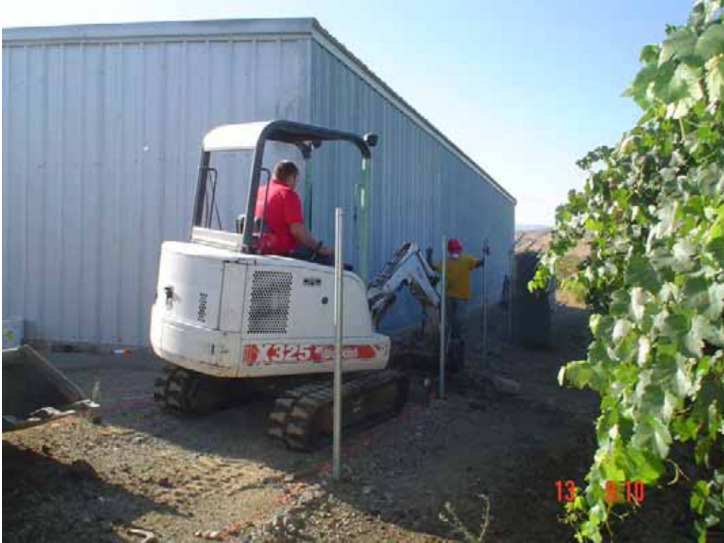
Beginning of Excavation in the Southern Portion of Area 4
