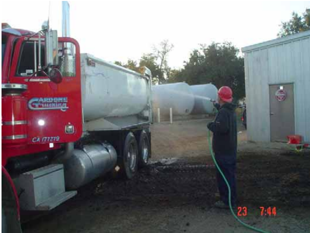
Cleaning Loose Particles from the Truck's Exterior
