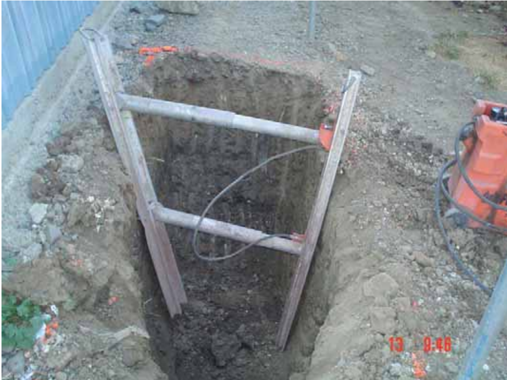
Installation of the Shoring System (Southern Portion of Excavation Area 4)
