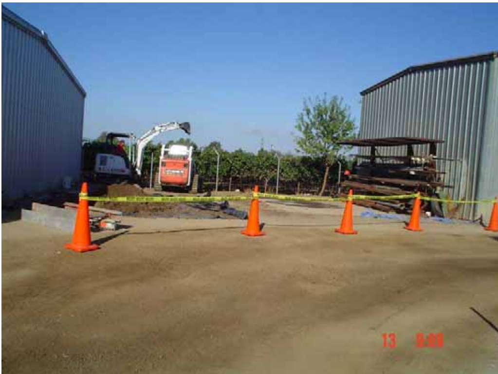
Secured Excavation Area
