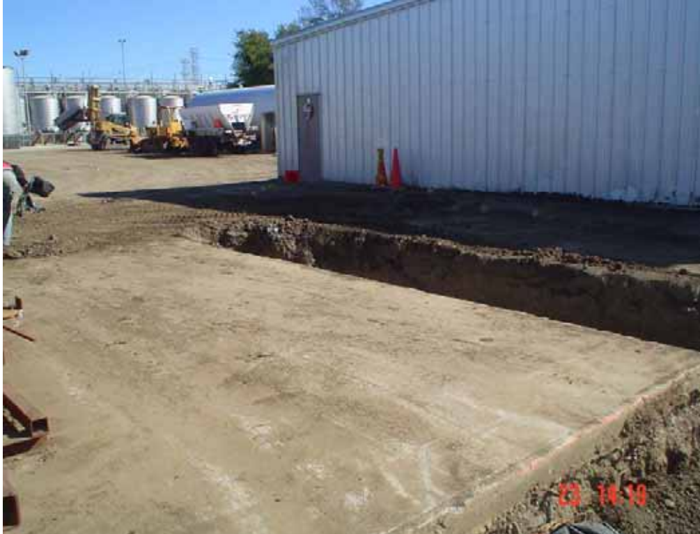
Cleaning the Excavation and Stockpile Areas
