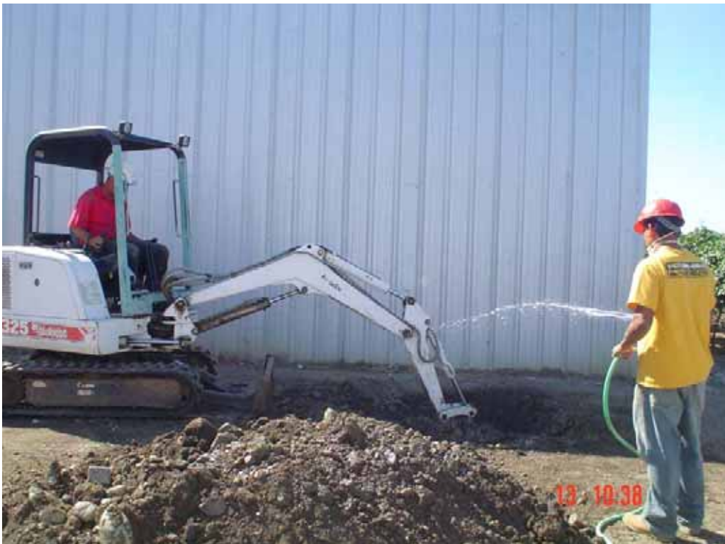
Dust Control Measures during the Excavation Activities
