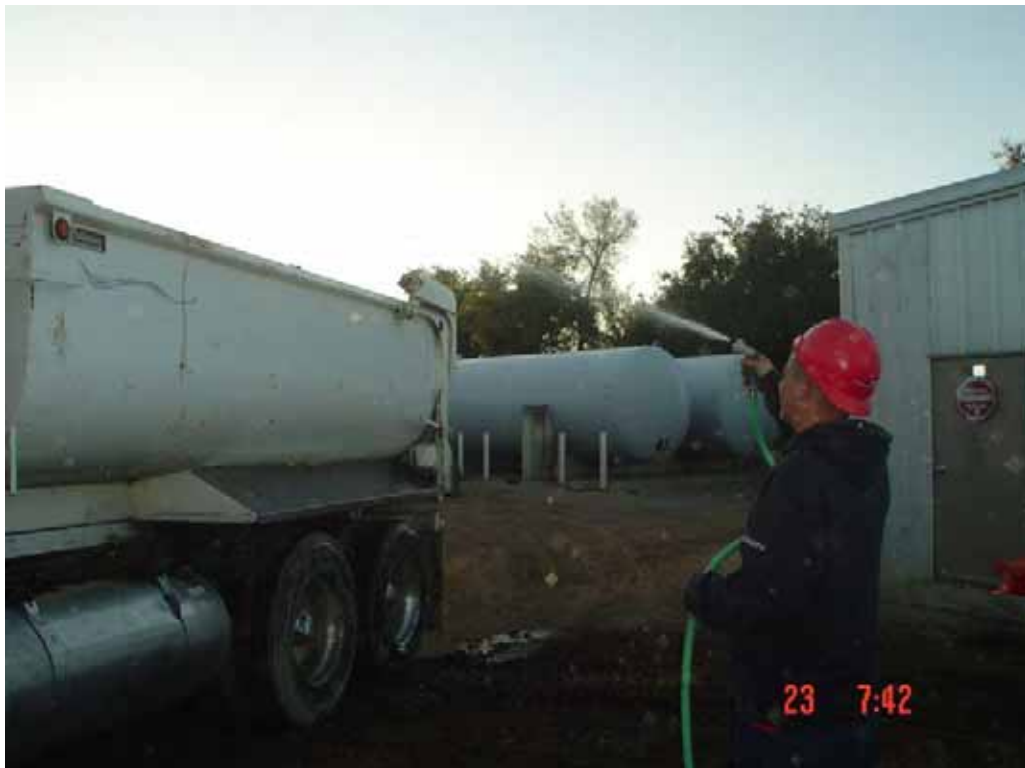
Watering of Soil Prior to Transport
