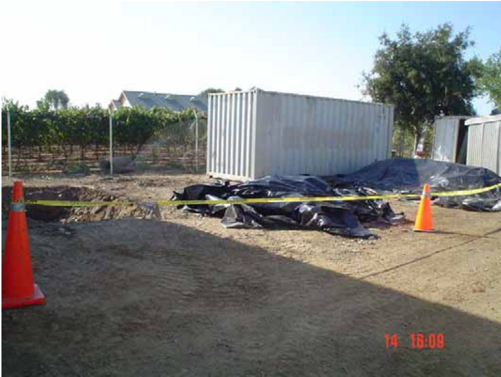
Excavation Area 1(View West)
