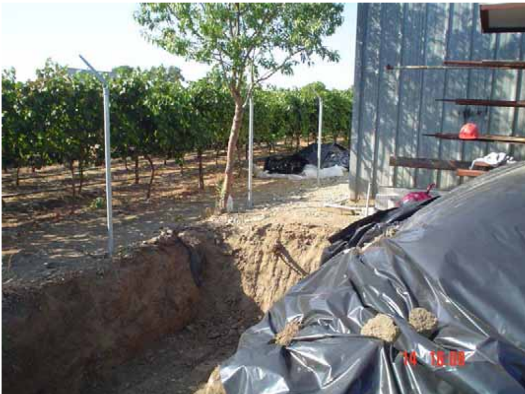
View of the Northern Portion of the Excavation Area 4
