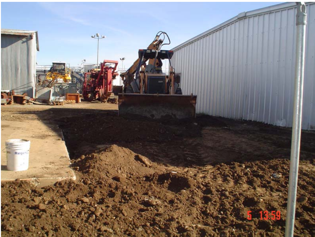
Plate 8: Final grading and re-compaction (view east)
