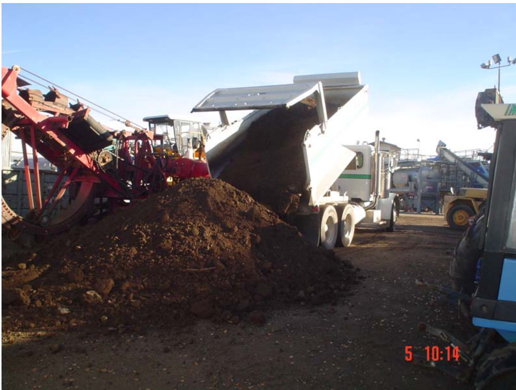
Plate 4: Clean fill stockpile, adjacent to the Area 4
