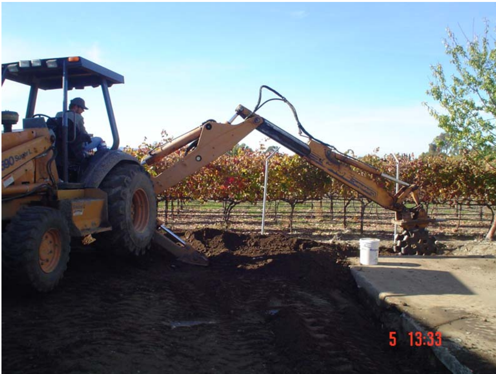
Plate 8: Area 4 being compacted (view west)
