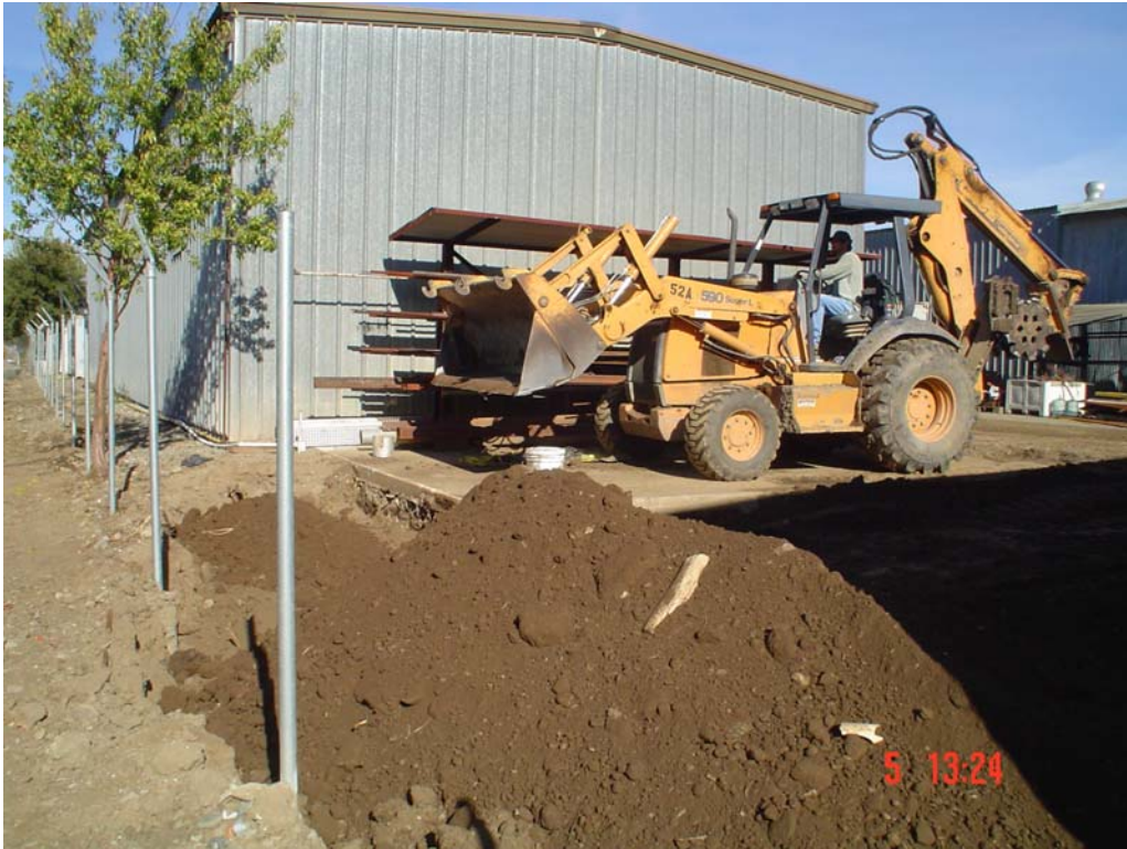
Plate 7: Area 4 being backfilled (view north)
