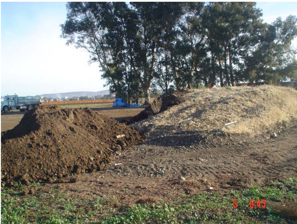
Plate 2: Clean fill stockpile, the side that was used for backfill (view northeast)
