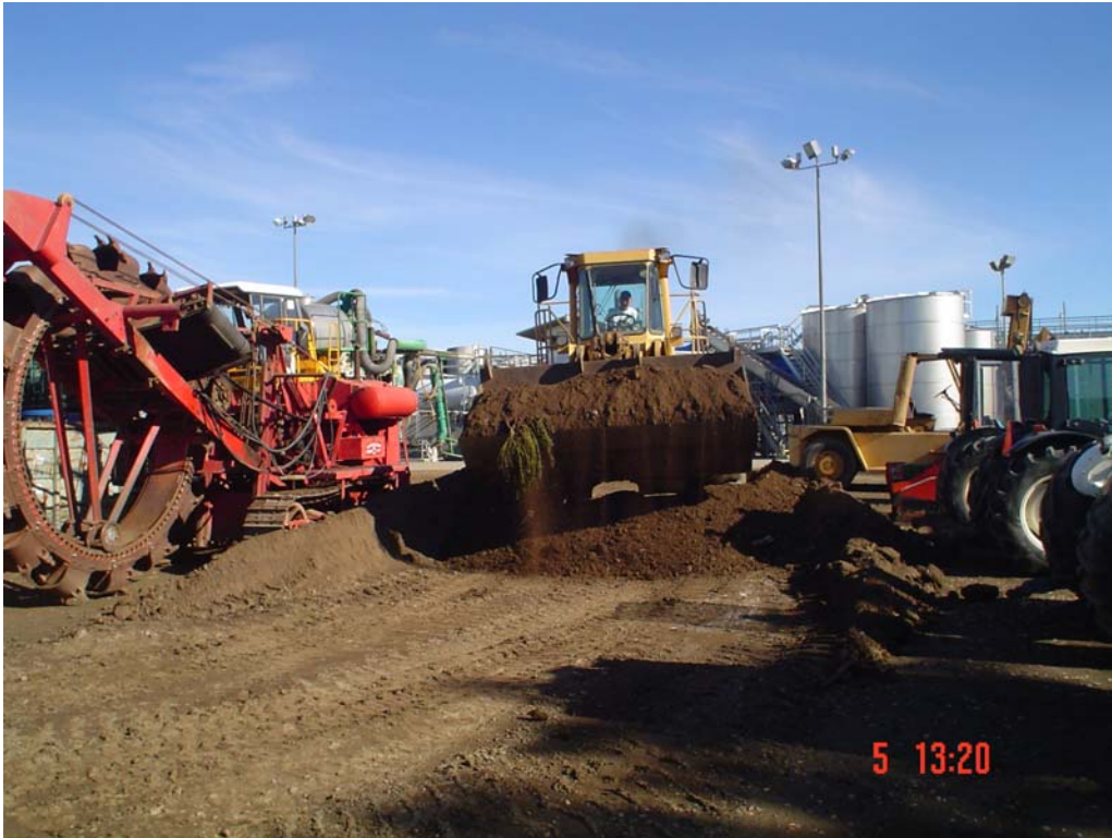
Plate 5: Clean fill being moved to the excavation areas
