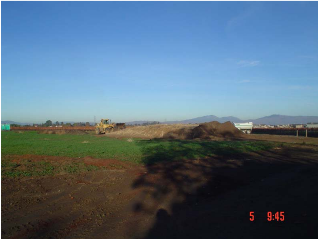
Plate 3: Clean fill being loaded for the transport (view west)
