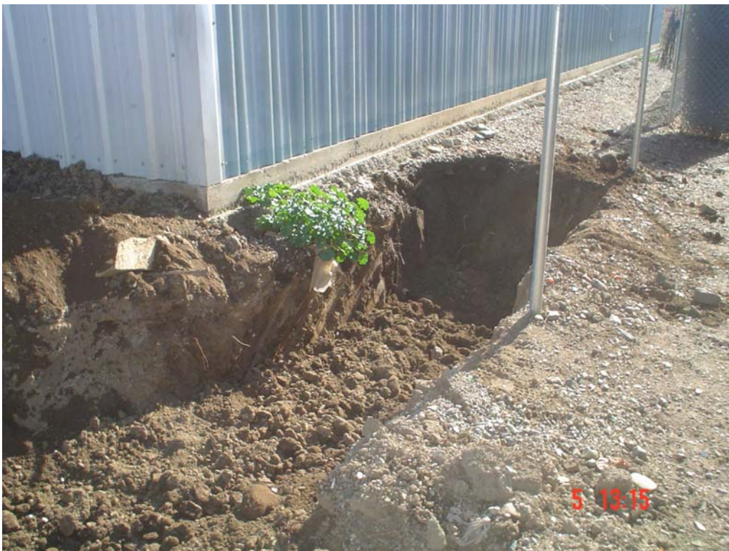
Plate 6: Area 4 backfilled 1/3 of the way (view south)
