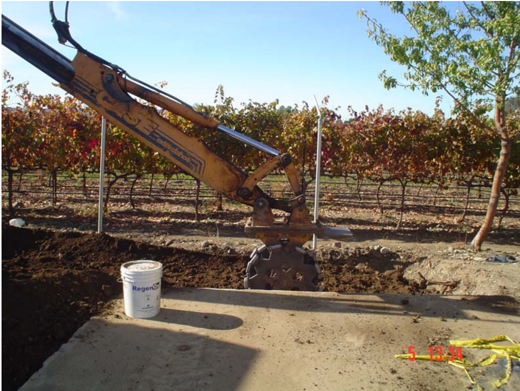
Plate 8: Area 4 being compacted (view west)
