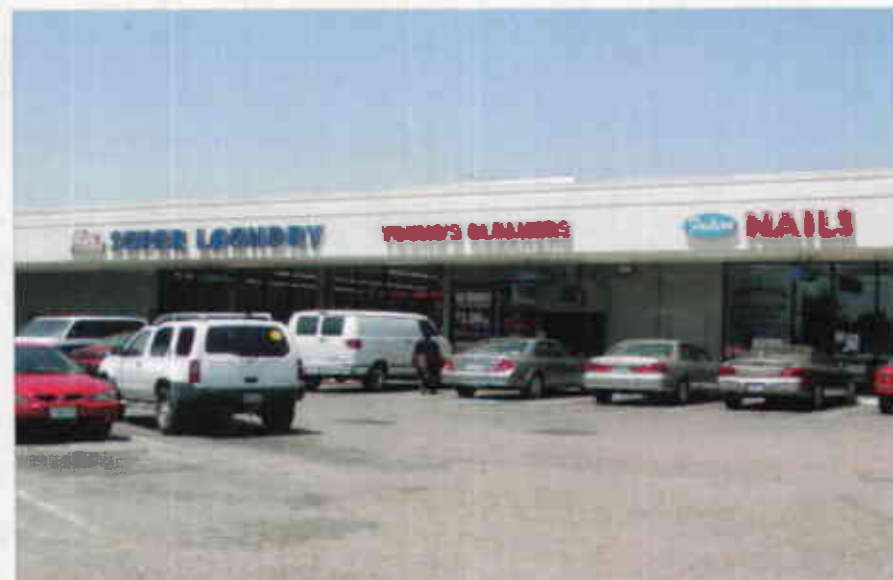
6. A view of the exterior of Young's Cleaners.
