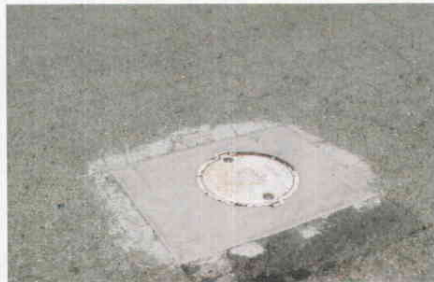
12. A view of another monitoring well located onsite.
