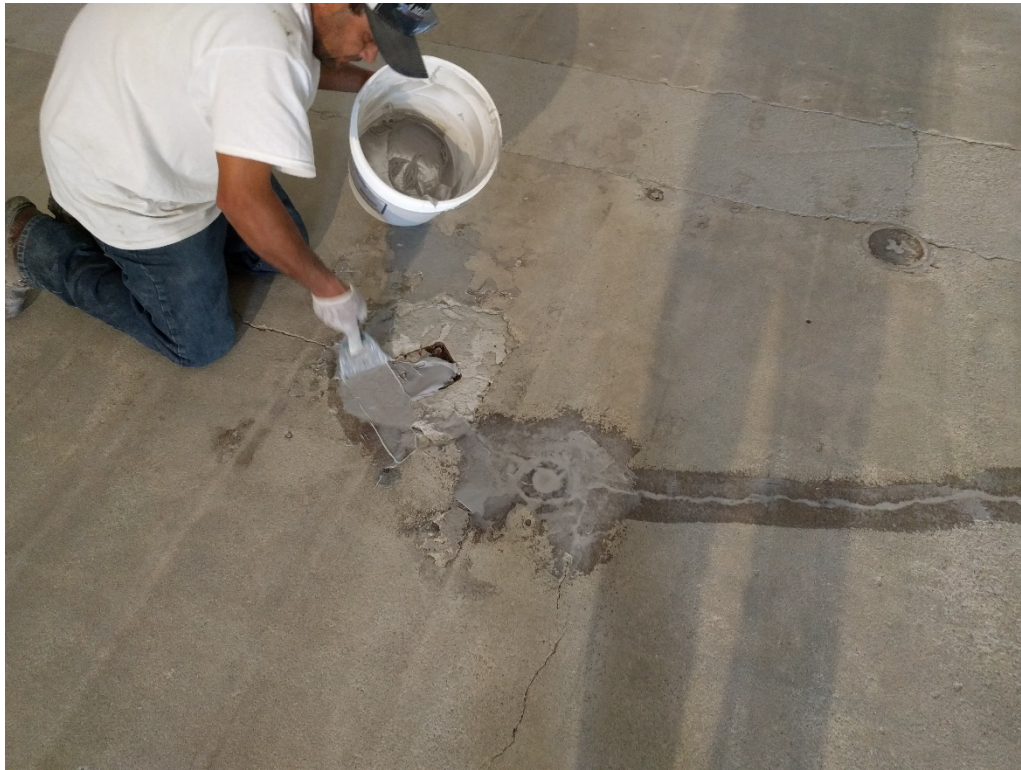
27. Application of Retro-coat Gel post abrasive surface preparation, but prior to primer application (03/11/2017)
