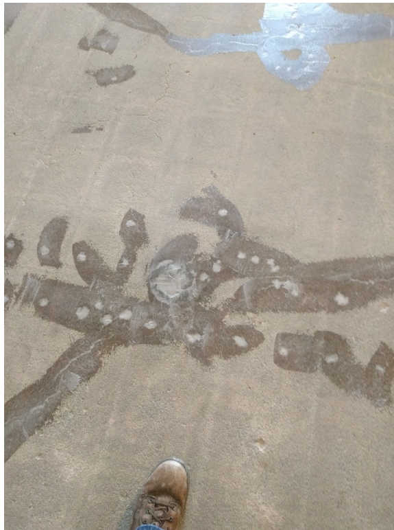
34. Representative close up of concrete repairs using Retro-coat Gel, pre primer application (03/11/2017)
