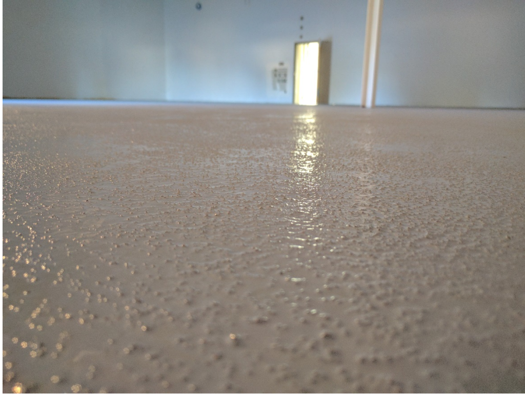
99. Close up of representative aggregate suspended in cured and finished Retro-coat Core layer 2 (03/14/2017)
