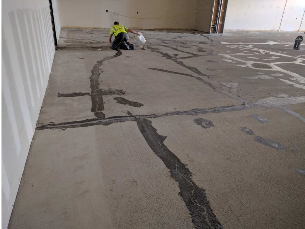
33. Retro-coat Gel application. View from W corner of sales area facing NE as in photo Nos 6, 70, and 96 (03/11/2017)
