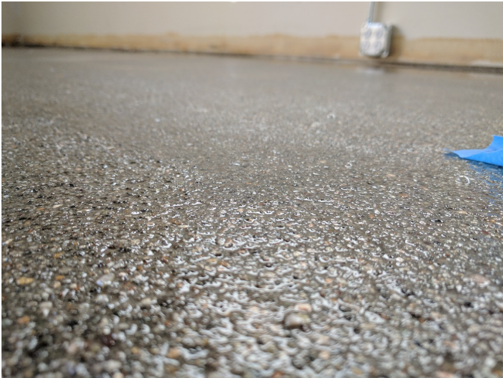
48. Representative close up of cured primer application (03/12/2017)
