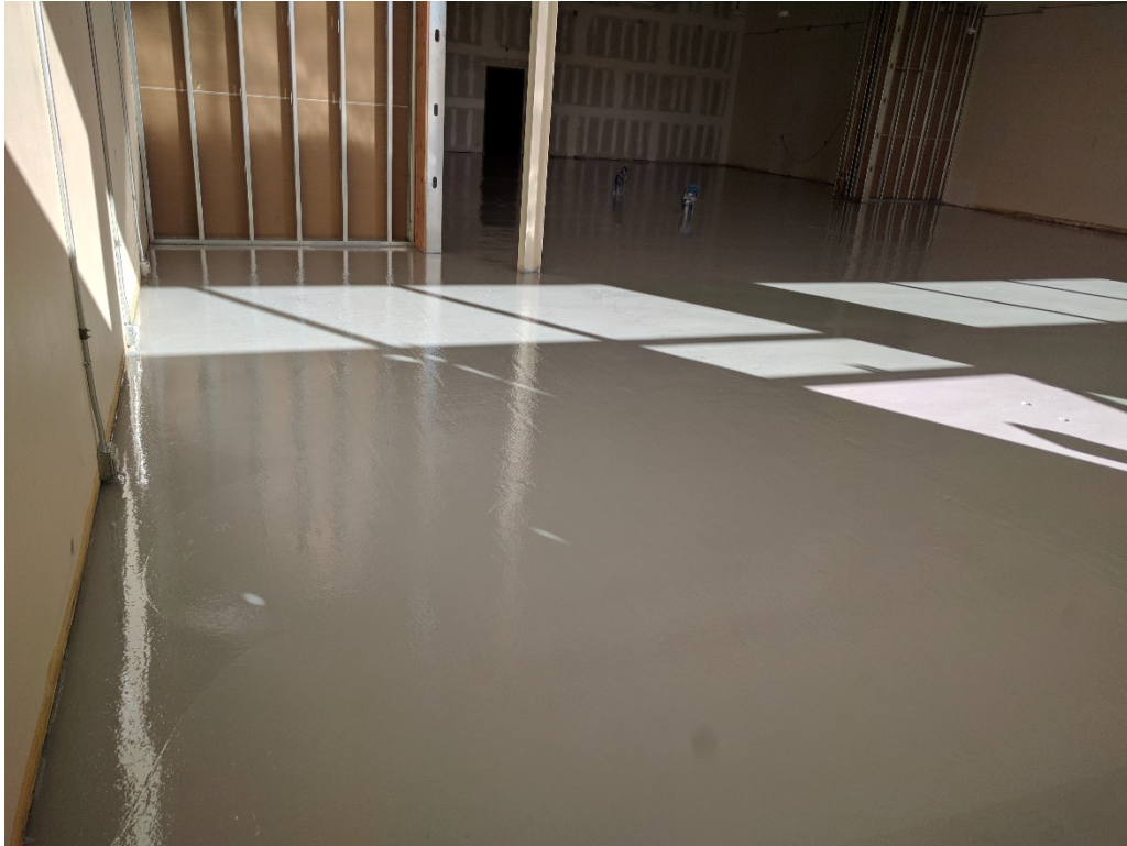
97. Cured and finished Retro-coat Core layer 2. View from S corner of sales are facing N as in photo Nos 4, 31, 46,
