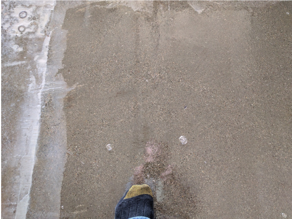
51. Close up of air bubbles in cured primer (3/12/2017)
