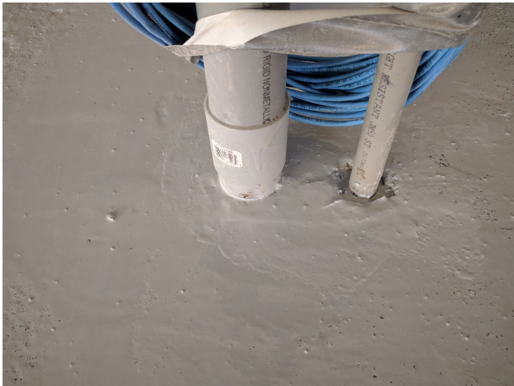
74. Cured Retro-coat Core layer 1 seal around electric and communications penetrations for POS podium in sales floor as in photo Nos 11, 82, and 108 (03/13/2017).
