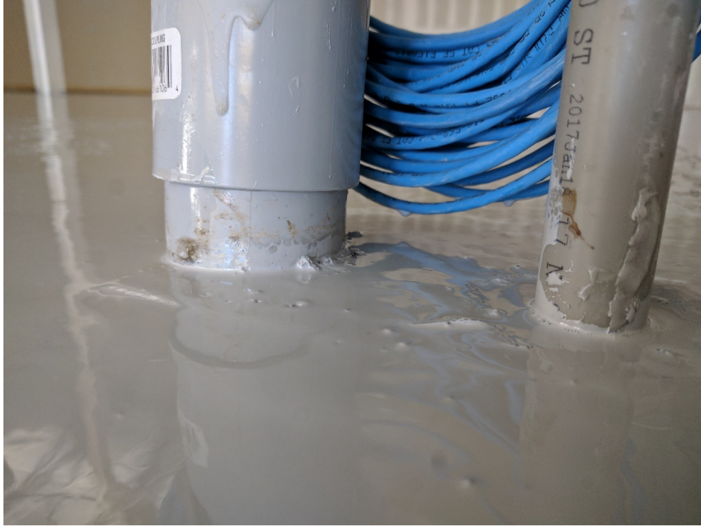
103. Representative seal from cured and finished Retro-coat Core layer 2 at penetration for electrical and communications lines for POS podium in sales floor as in photo Nos 11 and 74(03/14/2017)
