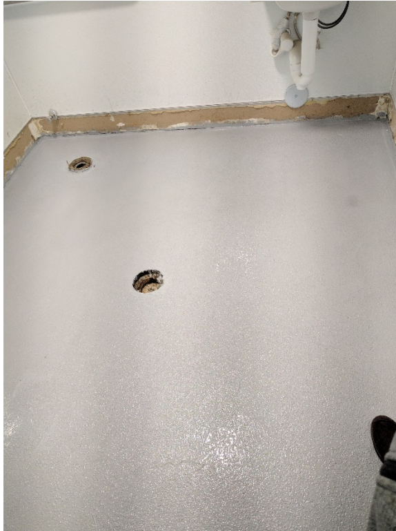
93. Cured and finished Retro-coat Core layer 2, women's restroom as in photo Nos 14, 45, and 67 (03/14/2017)
