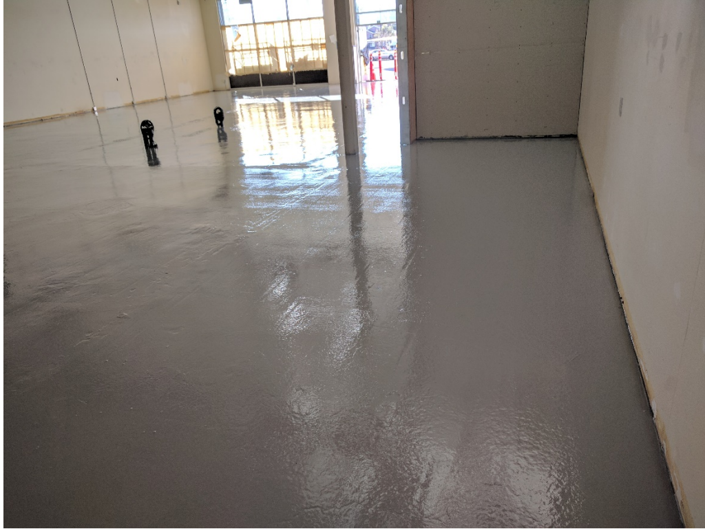
95. Cured and finished Retro-coat Core layer 2. View from W corner of sales area facing SE as in photo No 5, 32 and 69 (03/14/2017)
