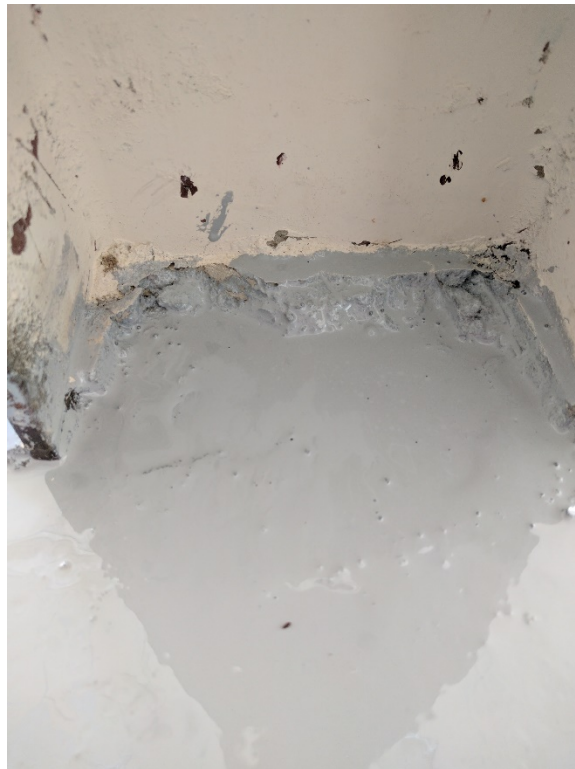
104. Representative cured and finished Retro-coat Core layer 2 at structural I-beam as in photo Nos 9 and 73 (03/14/2017).
