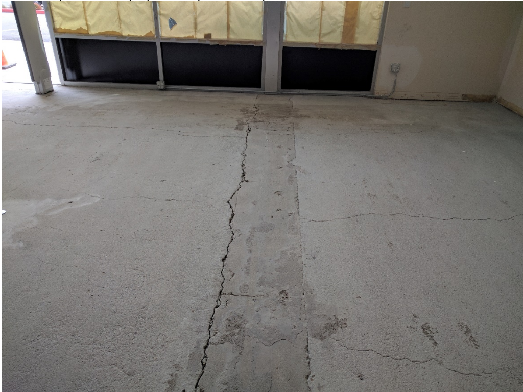
20. Cracks along grade beam, post surface preparation (03/10/2017)
