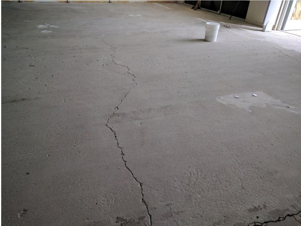
19. Representative cracks post surface preparation (03/11/2017)
