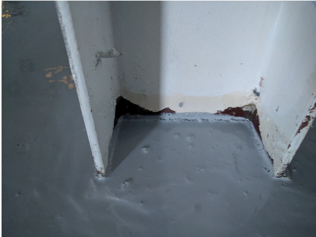
73. Representative cured Retro-coat Core layer 1 at structural I-beam as in photo Nos 9, 81, and 109 (03/13/2017)
