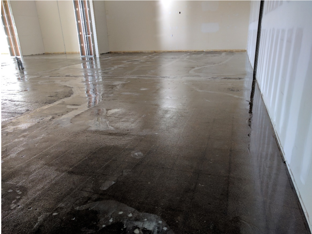
47. Cured primer application. View from E corner facing W as in photo Nos 68 and 94 (03/12/2017)
