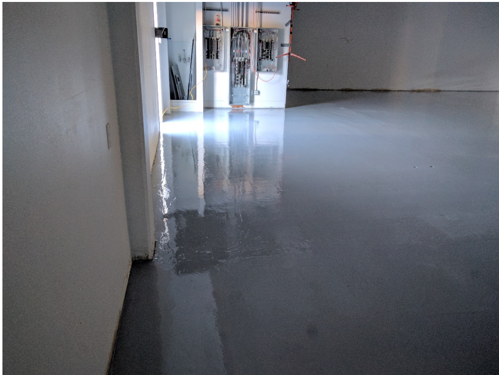
62. Cured Retro-coat layer 1. Photo taken from W corner of stock room facing N as in Photo Nos 28, 42, and 88 (03/13/2017)
