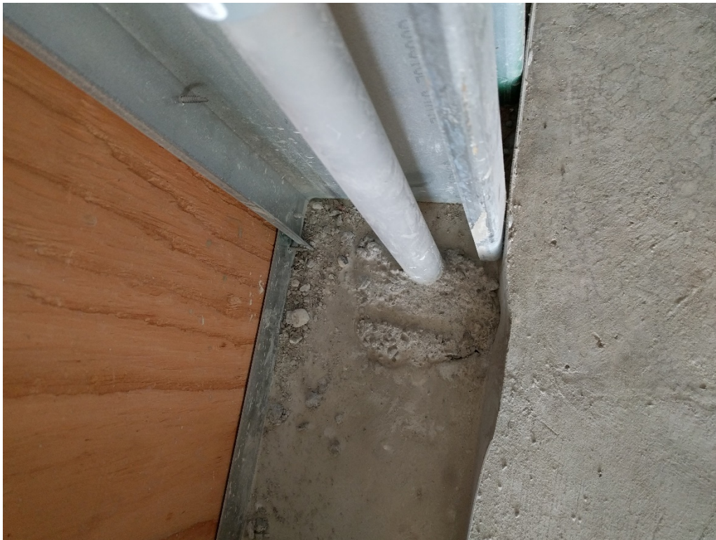
12. Penetration from ceiling for com/electric to sales floor POS podium as in photo No 71 (03/10/2017). Utilities run sub-grade to location of POS podium through a trench installed as part of TI.
