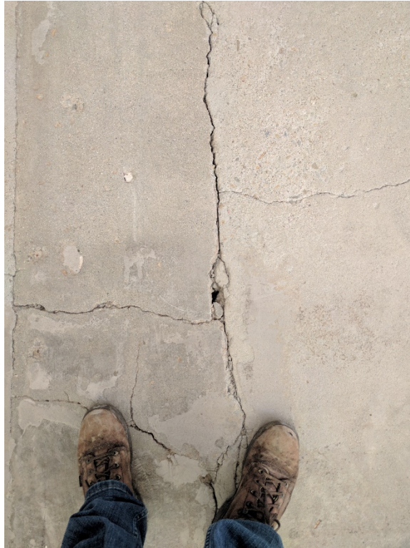
21. Cracks along grade beam, post surface preparation (03/10/2017)
