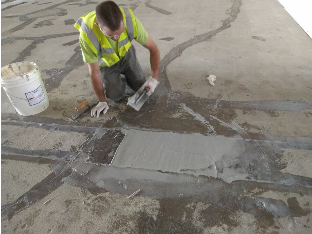
35. Floating of damaged trench area in sales area (see photo No. 26) using Retro-coat Gel (03/11/2017)
