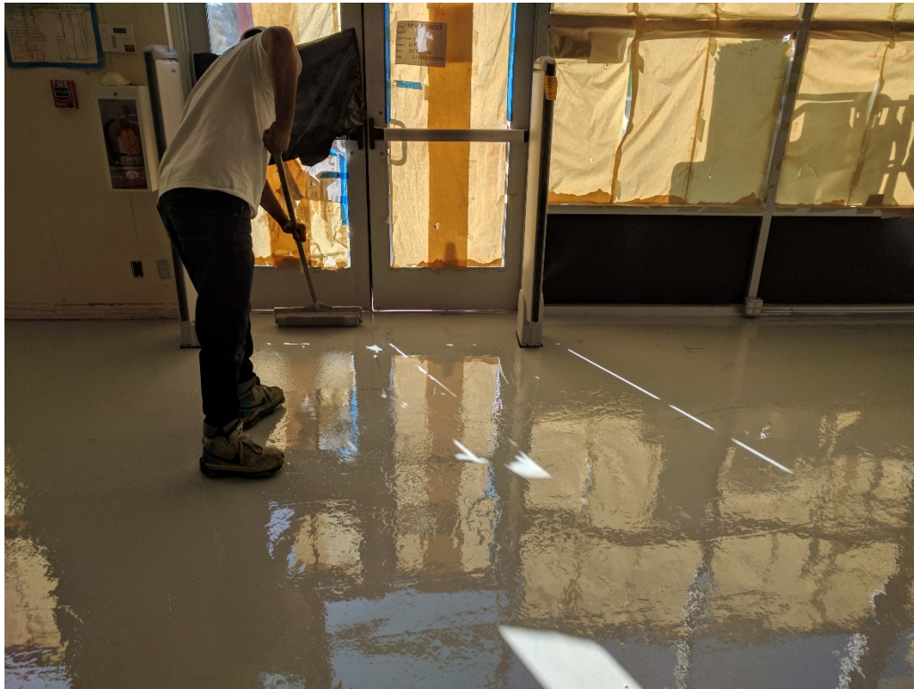
61. Representative backrolling of Retro-coat core layer 1 (03/12/2017)
