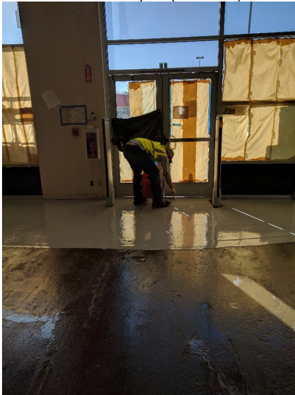
60. Representative detailing of Retro-coat Core layer 1 using a brush (03/12/2017)
