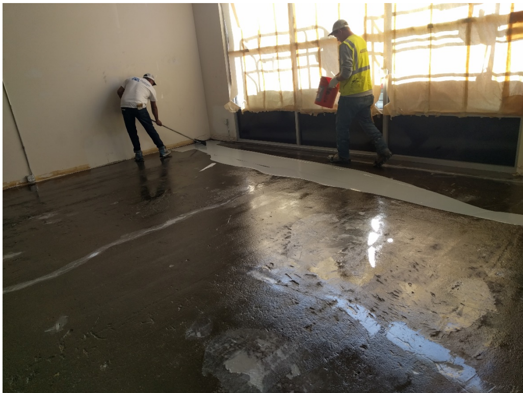
58. Representative ribbon pour of Retro-coat Core layer 1 (03/12/2017)
