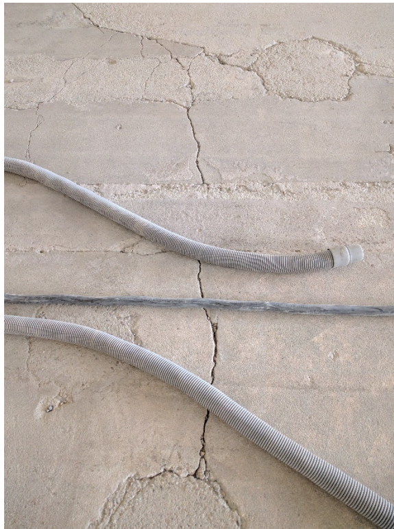
22. Representative cracks along historic penetrations and trenches. (03/10/2017)
