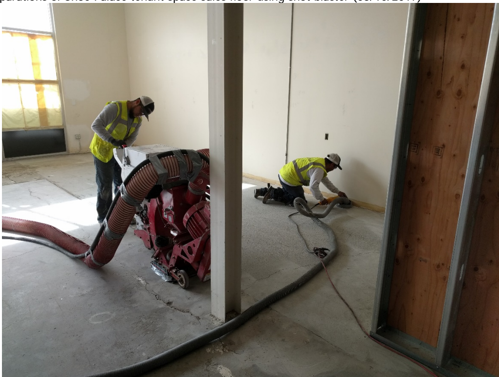
8. Surface preparations of Shoe Palace tenant space sales floor using shot blaster and grinder (03/10/2017)
