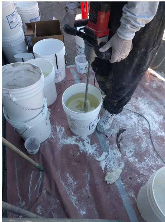
38. Retro-coat Primer preparation; 1 gallon of Part B into 3.5 gallons Part A, mixed for two minutes (03/11/2017)
