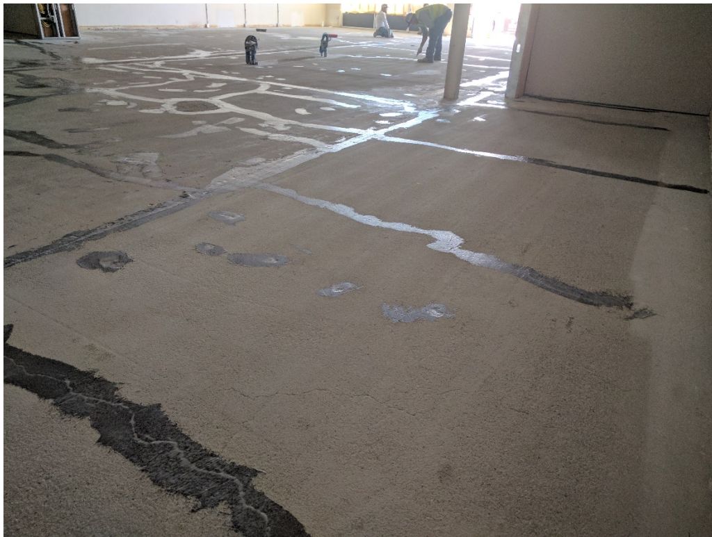
32. Retro-coat Gel application. View from W corner of sales area facing SE as in photo Nos 5, 69, and 95 (03/11/2017)
