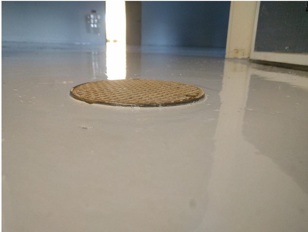
77. Representative Retro-coat Core layer 1 seal at access point
