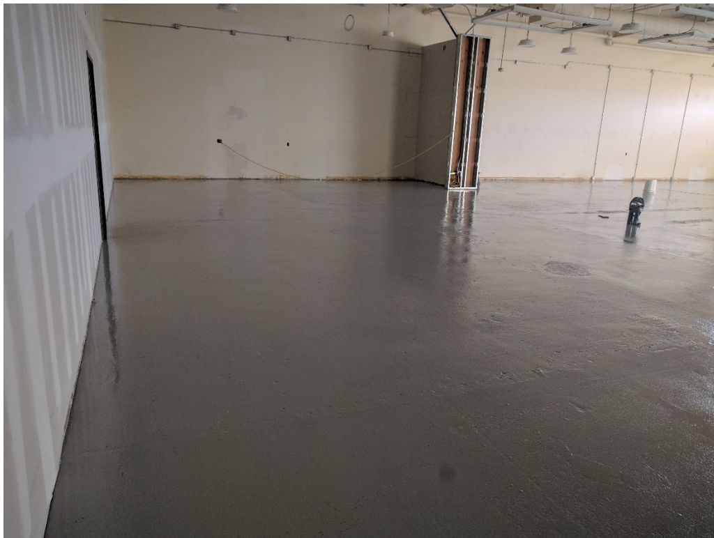
70. Cured Retro-coat Core layer 1. View from W corner of sales area facing NE as in photo Nos 6, 33, and 96 (03/13/2017)
