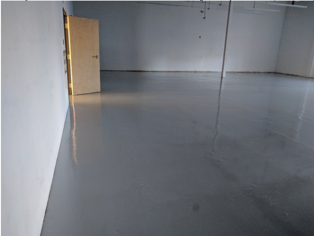
64. Cured Retro-coat layer 1. Photo taken from S corner of stock room facing W as in photo Nos 43 and 90 (03/13/2017)
