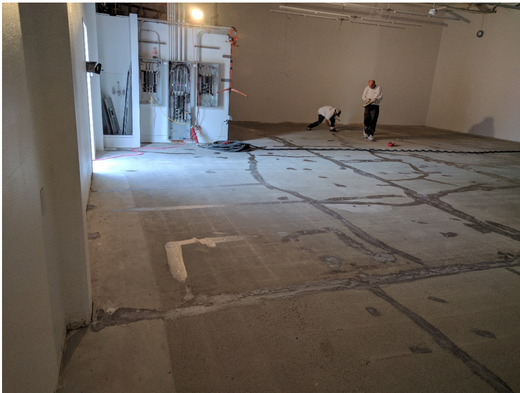
28. Application of Retro-coat Gel to seal cracks post surface preparation, but prior to primer application. Photo taken from W corner of stock room facing N as in photo Nos 42, 69, and 88 (03/11/2017)
