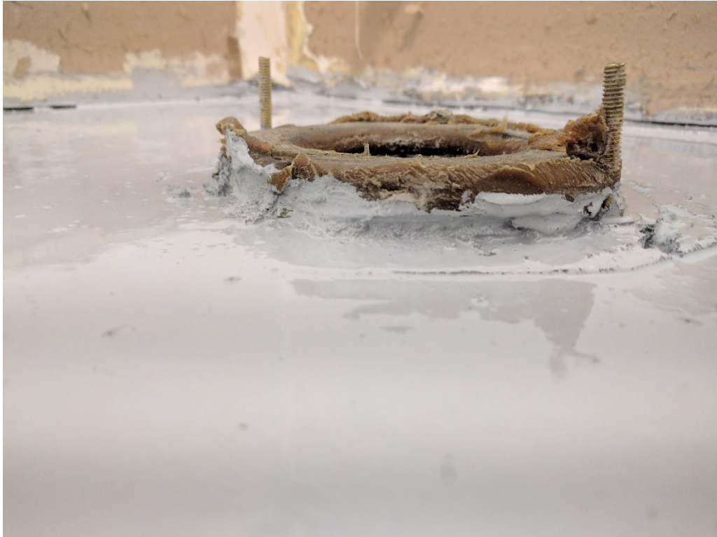
75. Cured Retro-coat Core seal around toilet (03/13/2017)
