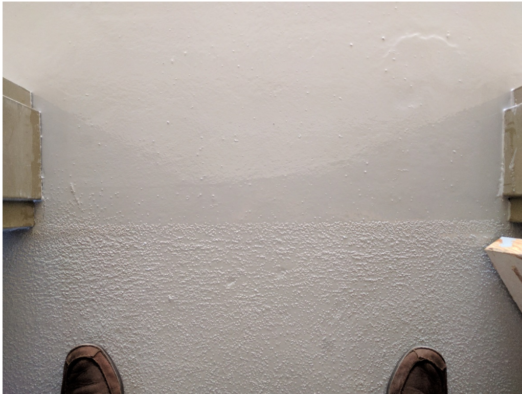
101. Transition from sales floor (no aggregate) to stock room (aggregate) for cured and finished Retro-coat Core layer 2 (03/14/2017)
