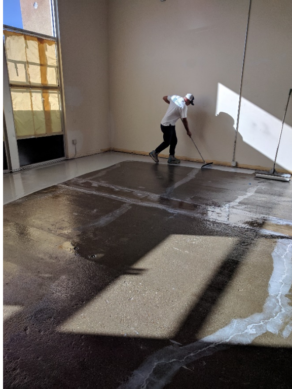
59. Representative squeegee application of Retro-coat Core layer 1 (03/12/2017)
