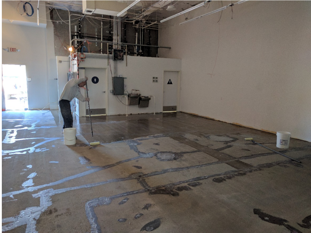
41. Representative application of Retro-coat Primer to an \approx 6 mil thickness as in photo Nos 65 and 91 (03/11/2017)
