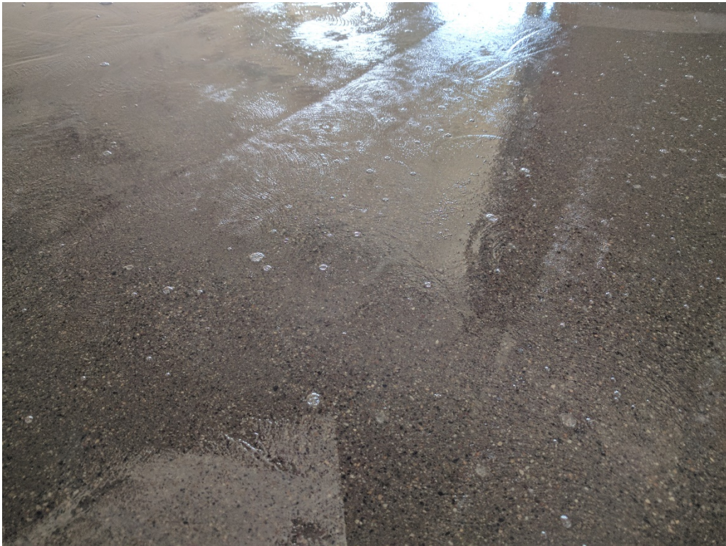
50. Air bubbles in cured primer (03/12/2017)
