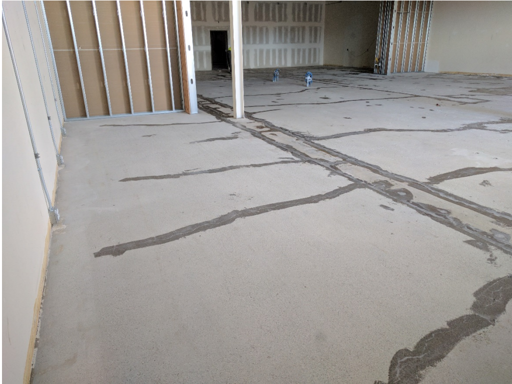
31. Retro-coat Gel application. View from S corner of sales area facing N as in photo Nos 4, 46, and 97 (03/11/2017)
