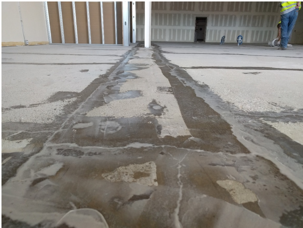
36. Close up of Retro-coat Gel application along grade beam. Photo taken from SE portion of sales area facing NW (03/11/2017)
