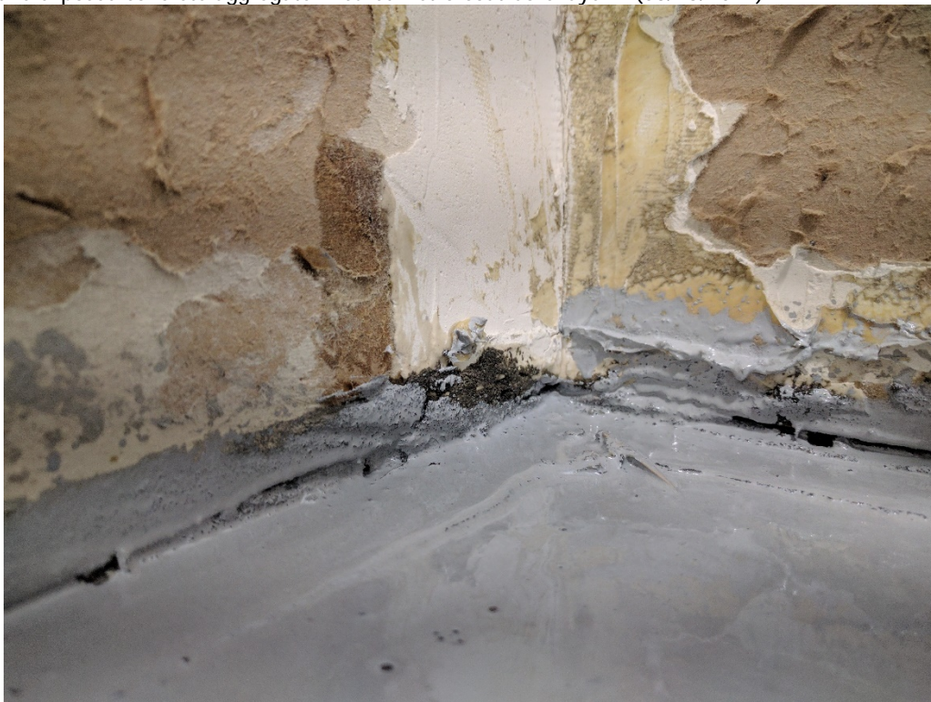
80. Representative Retro-coat Core layer 1 seal at vertical wall as in photo No 105 (03/13/2017)
