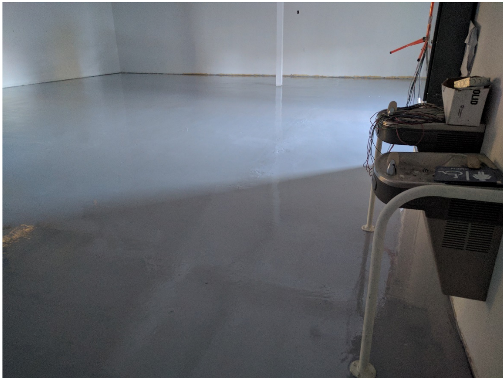
66. Cured Retro-coat layer 1. Photo taken from N corner of stock room facing S as in photo Nos 44 and 92 (3/13/2017)
