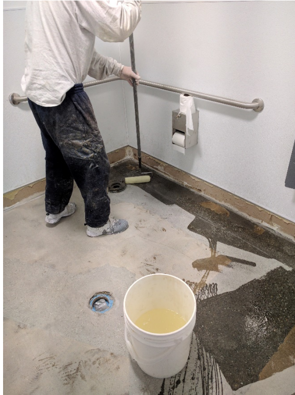
39. 6 mil application of Retro-coat Primer to mens restroom using soft roller (03/11/2017)
