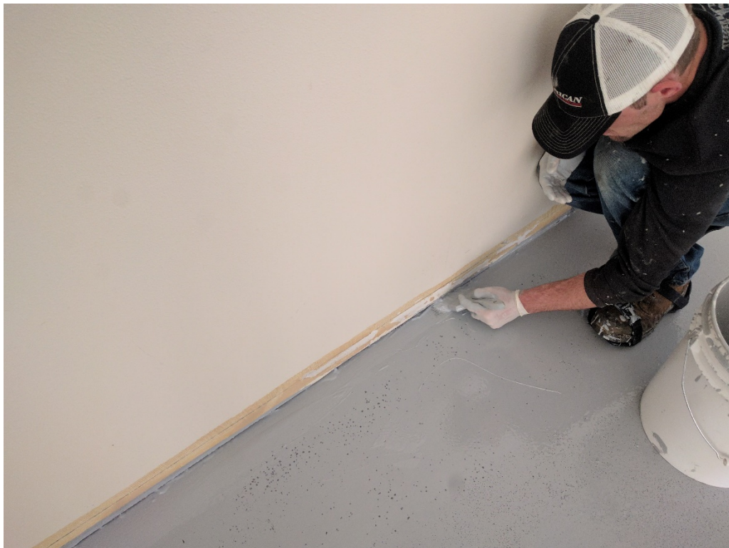
81. Representative cured Retro-coat Core application layer 1 around cox-colvin sub-slab and soil vapor probe locations as in photo Nos (03/13/2017)
