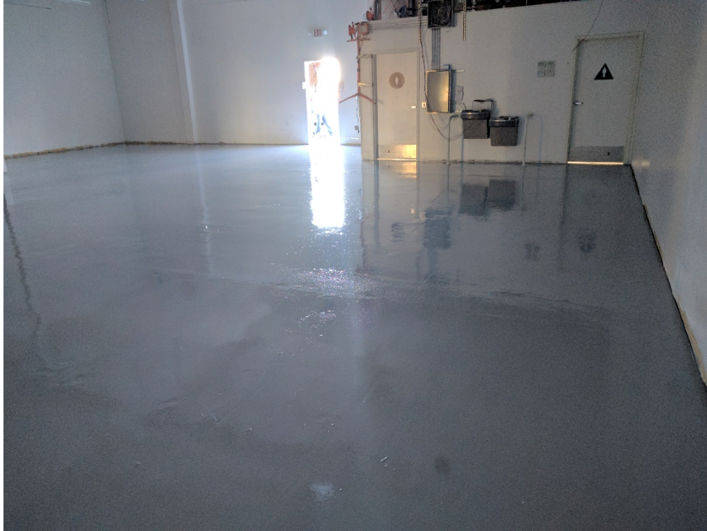
65. Cured Retro-coat layer 1. Photo taken from S corner of stock room facing NW as in photo Nos 41 and 91 (03/13/2017)
