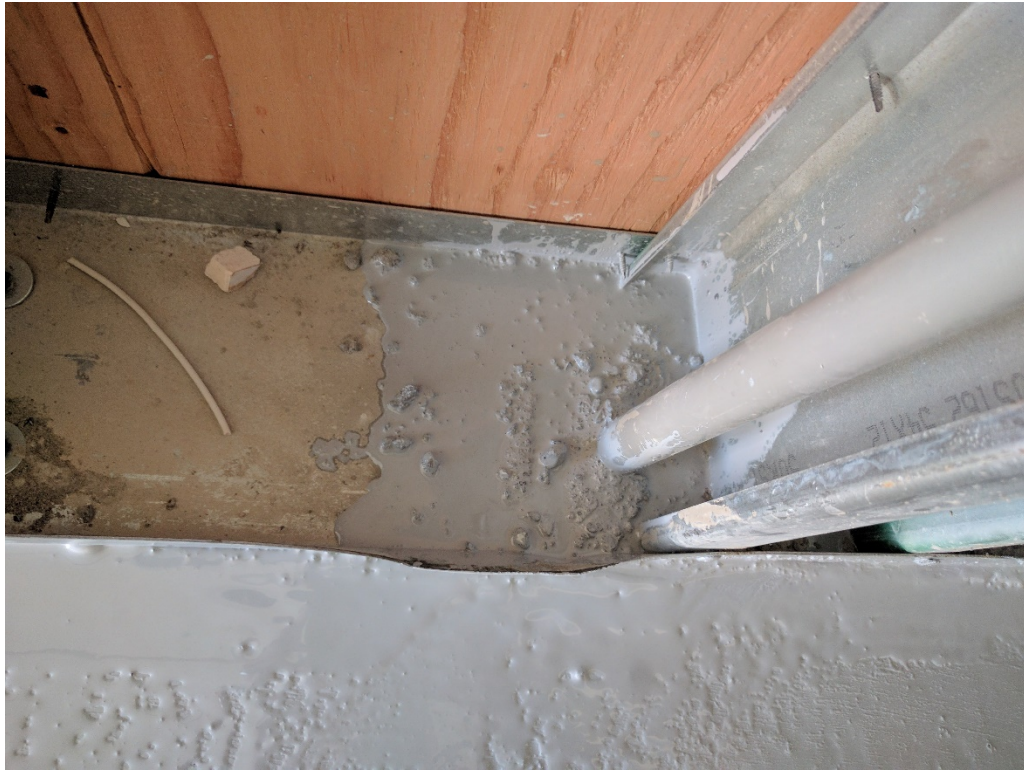
71. Retro-coat Core seal of penetration from ceiling for com/electric to sales floor POS podium as depicted in photo No 12 (03/13/2017)
