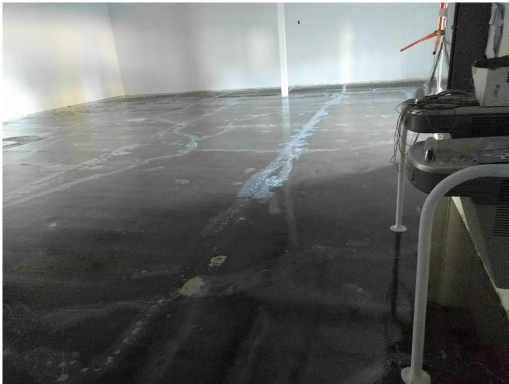
44. Cured primer application. Photo taken from N corner of stock room facing S as in photo Nos 66 and 92 (3/12/2017)
