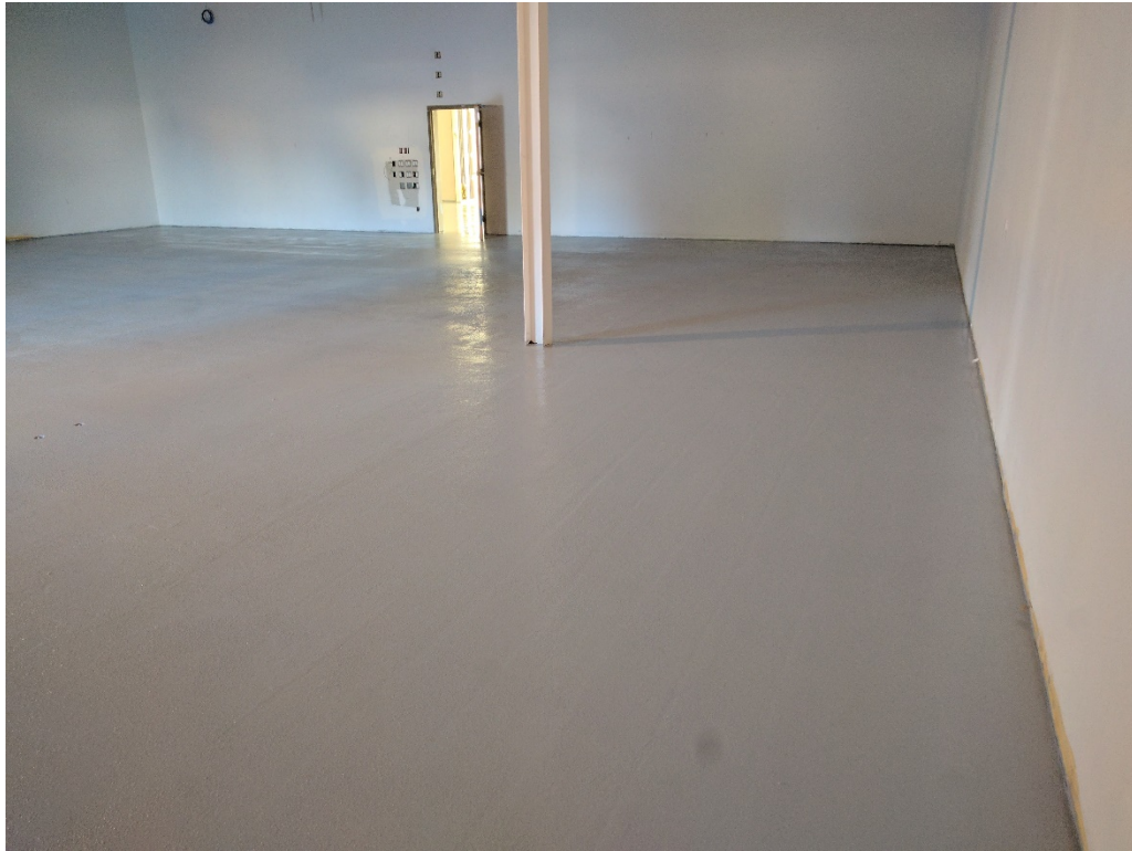
89. Cured and finished Retro-coat Core layer 2 with sand aggregate. Photo taken from W corner of stock room facing E as in photo 63 (03/14/2017)
