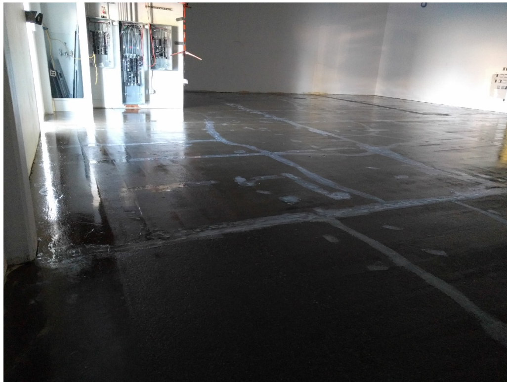
42. Cured primer application. Photo taken from W corner of stock room facing N as in photo Nos 28, 62, and 88 (03/12/2017)
