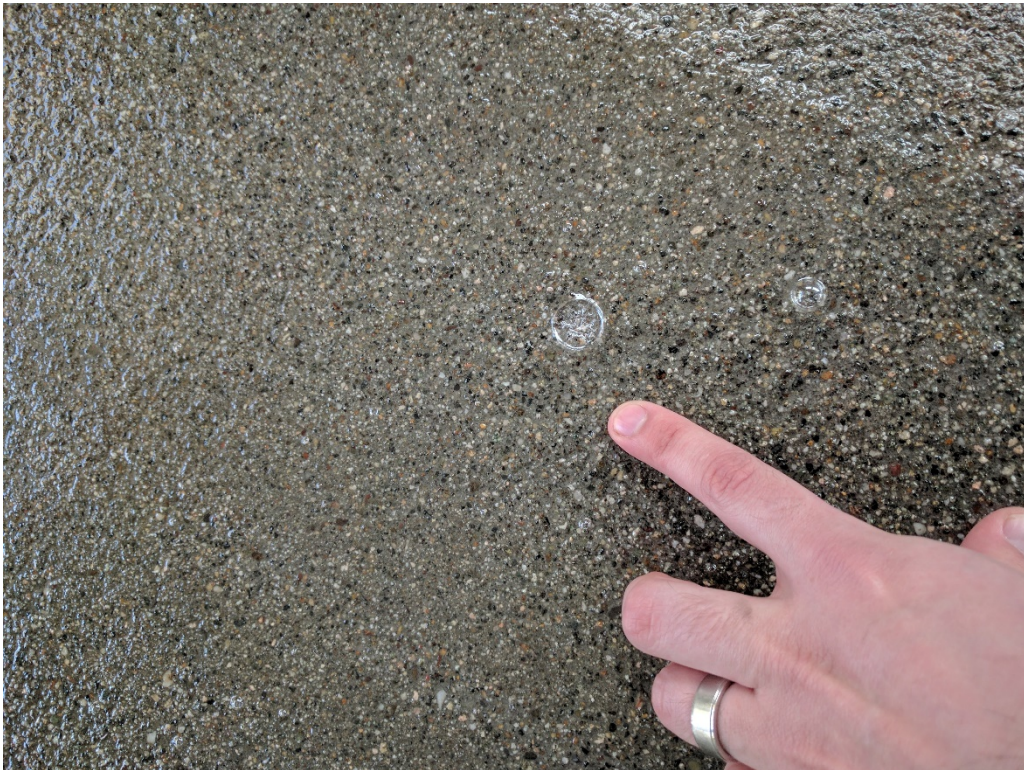
52. Close up of air bubbles in cured primer (03/12/2017)
