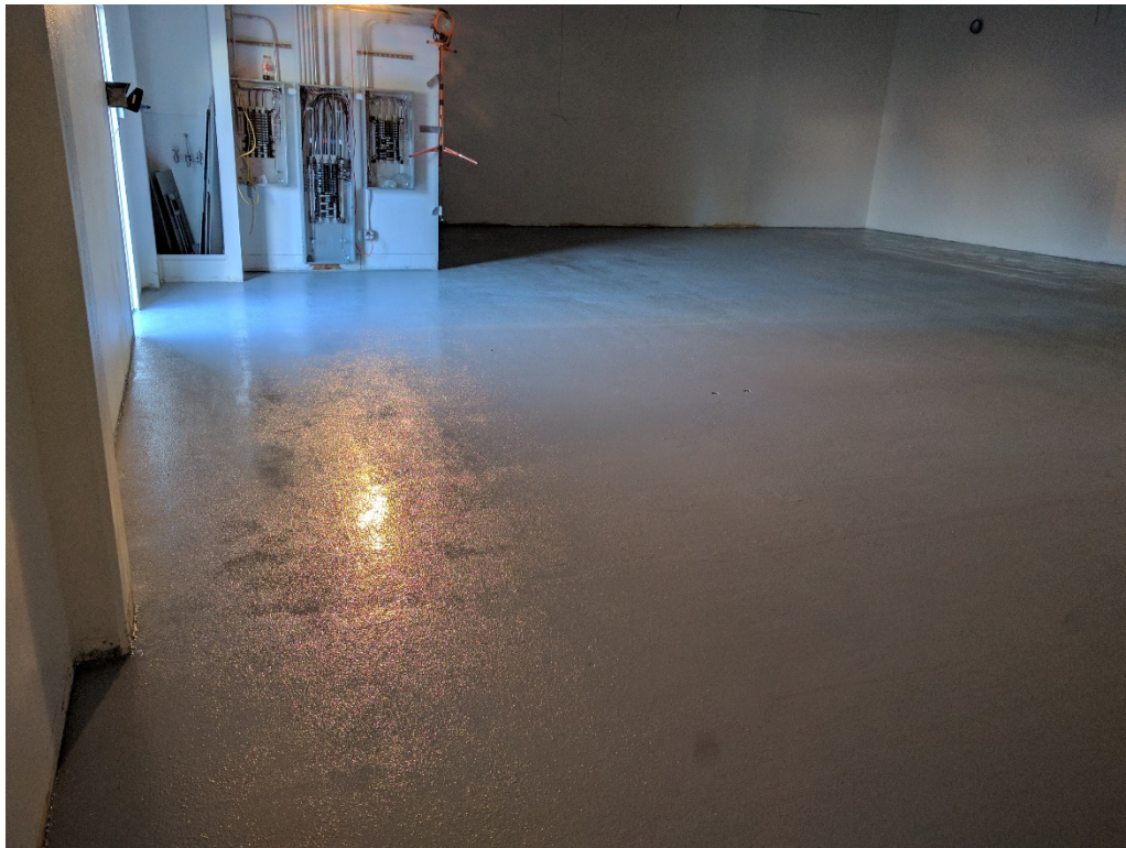
88. Cured and finished Retro-coat Core layer 2 with sand aggregate. Photo taken from W corner of stock room facing N as in Photo Nos 28, 42, and 62 (03/14/2017)
