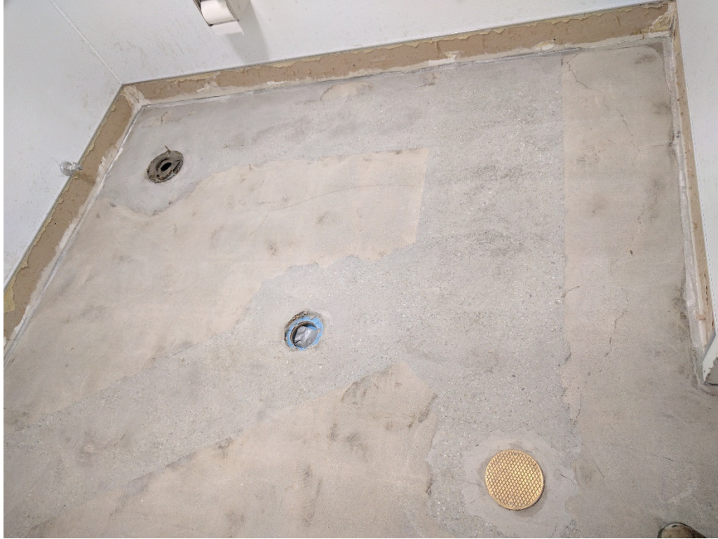
15. Mens restroom, post surface preparation. Location of utility trenches installed as part of TI visible (3/11/2017)
