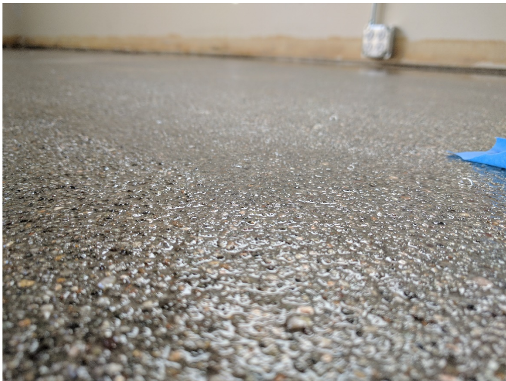
48. Representative close up of cured primer application (03/12/2017)
