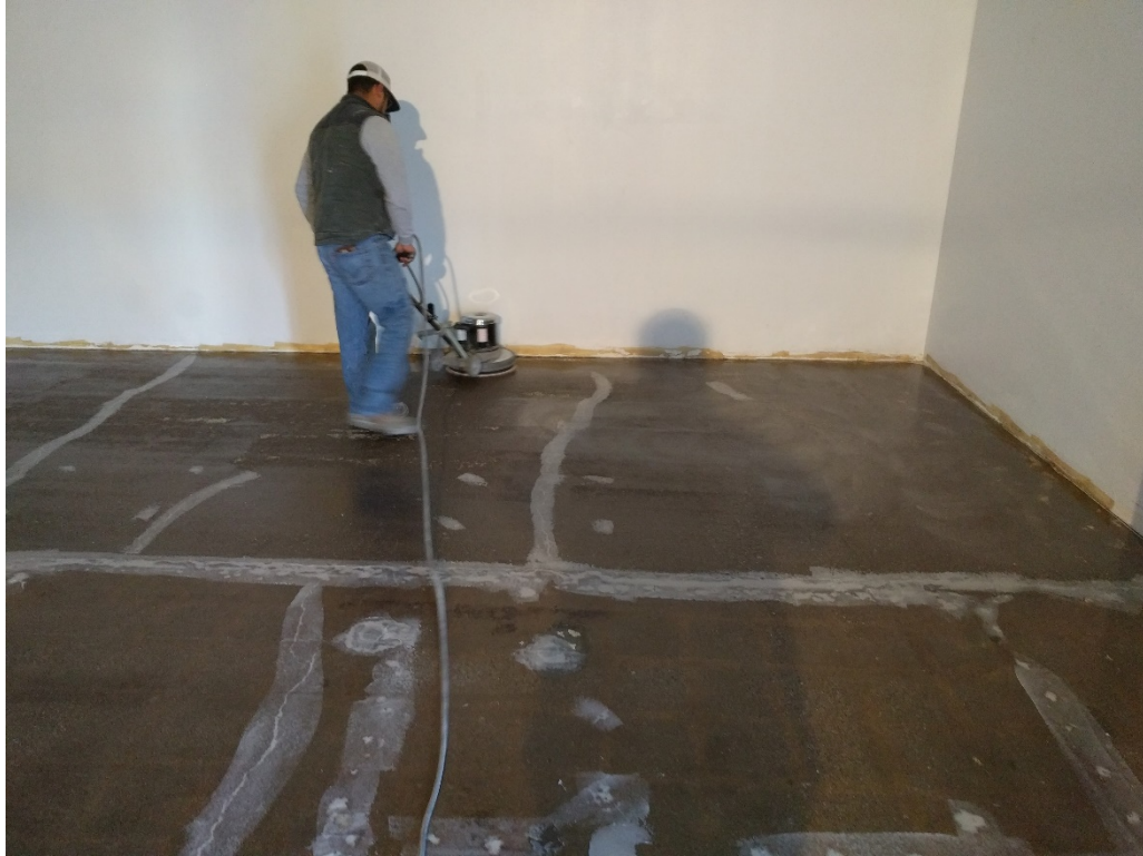
57. Removal of bubbles in primer using fine grit sander (03/12/2017)
