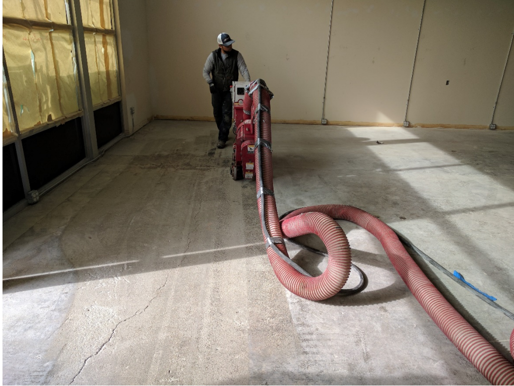
7. Surface preparations of Shoe Palace tenant space sales floor using shot blaster (03/10/2017)
