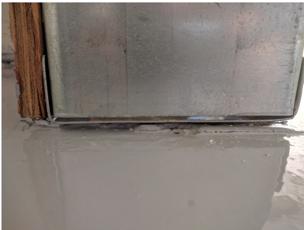
102. Representative cured and finished Retro-Coat Core layer 2 at delimiting wall on sales floor.
