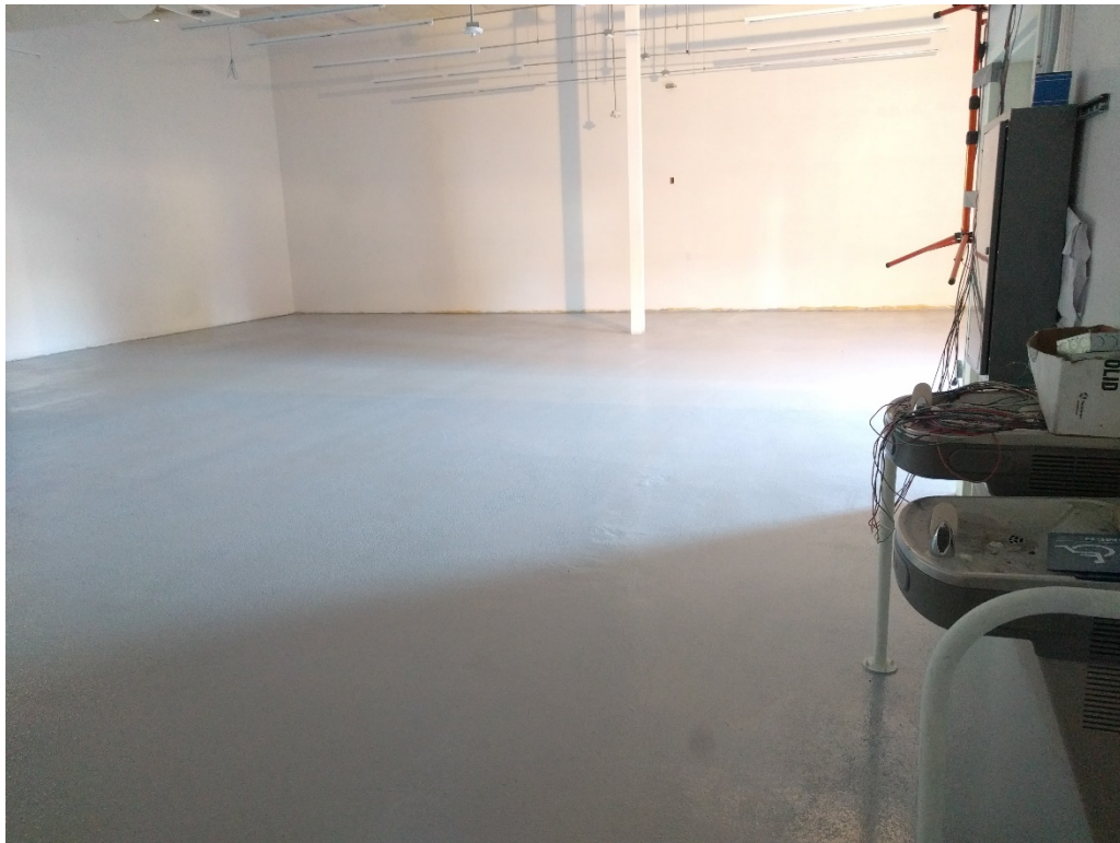
92. Cured and finished Retro-coat Core layer 2 with sand aggregate. Photo taken from N corner of stock room facing S as in photo Nos 66 (3/14/2017)
