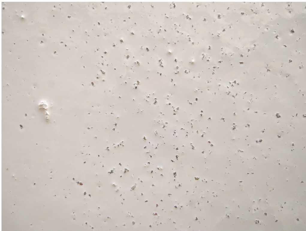
78. Representative exposed concrete aggregate in cured Retro-coat Core layer 1 (03/13/2017)
