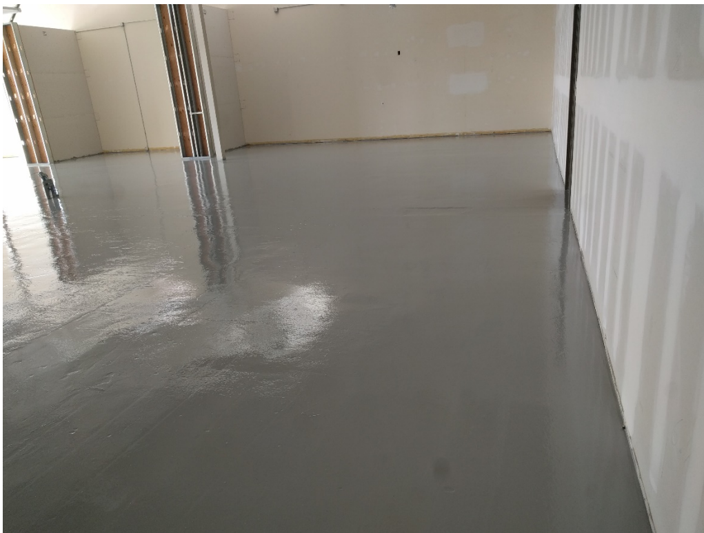
94. Cured and finished Retro-coat Core layer 2. View from E corner facing W as in photo Nos 47 and 68 (03/14/2017)
