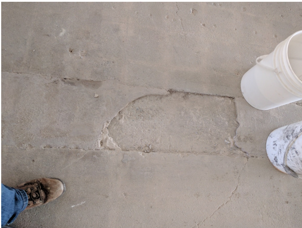
26. Damage to trenching between sales area and stock area as in photo No 35 (03/11/2017)
