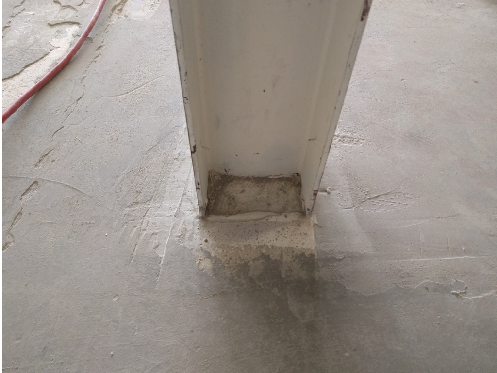
9. Surface penetration, representative structural I-beam as in photo Nos 73, and 104 (03/10/2017)
