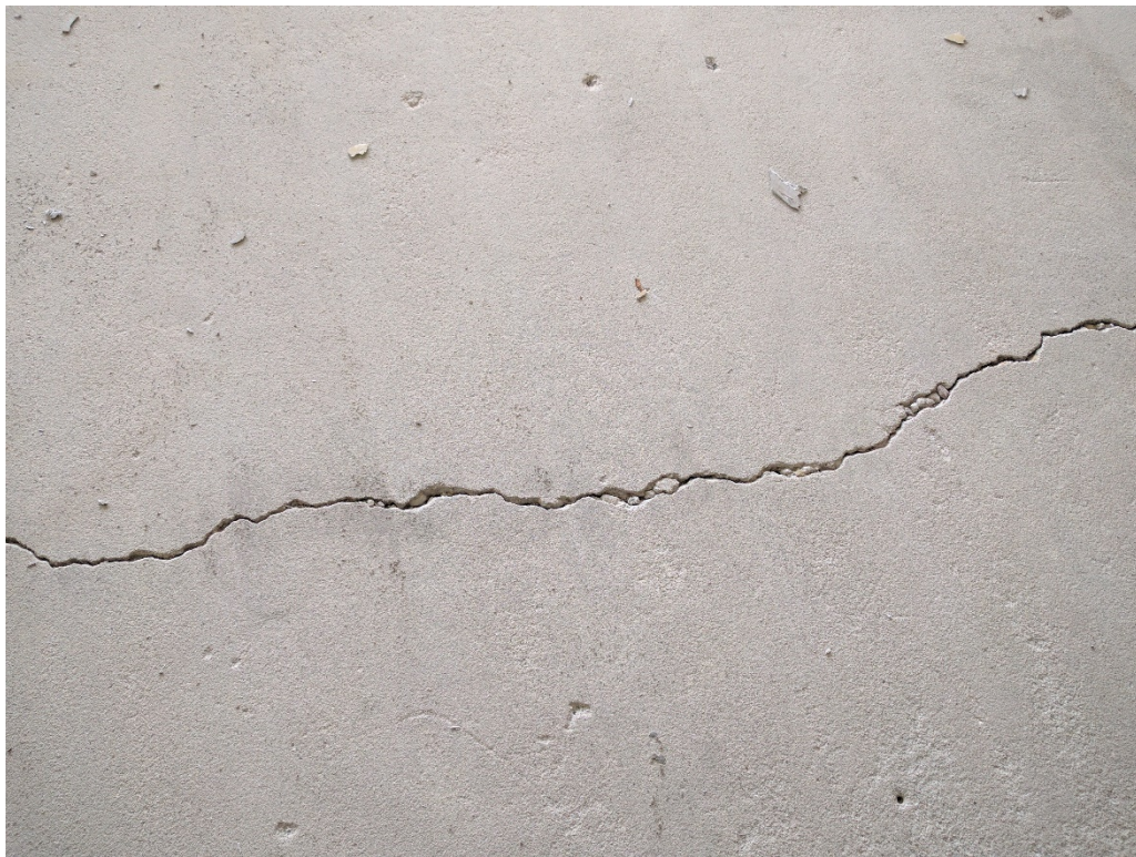
18. Representative cracks post surface preparation (03/11/2017)
