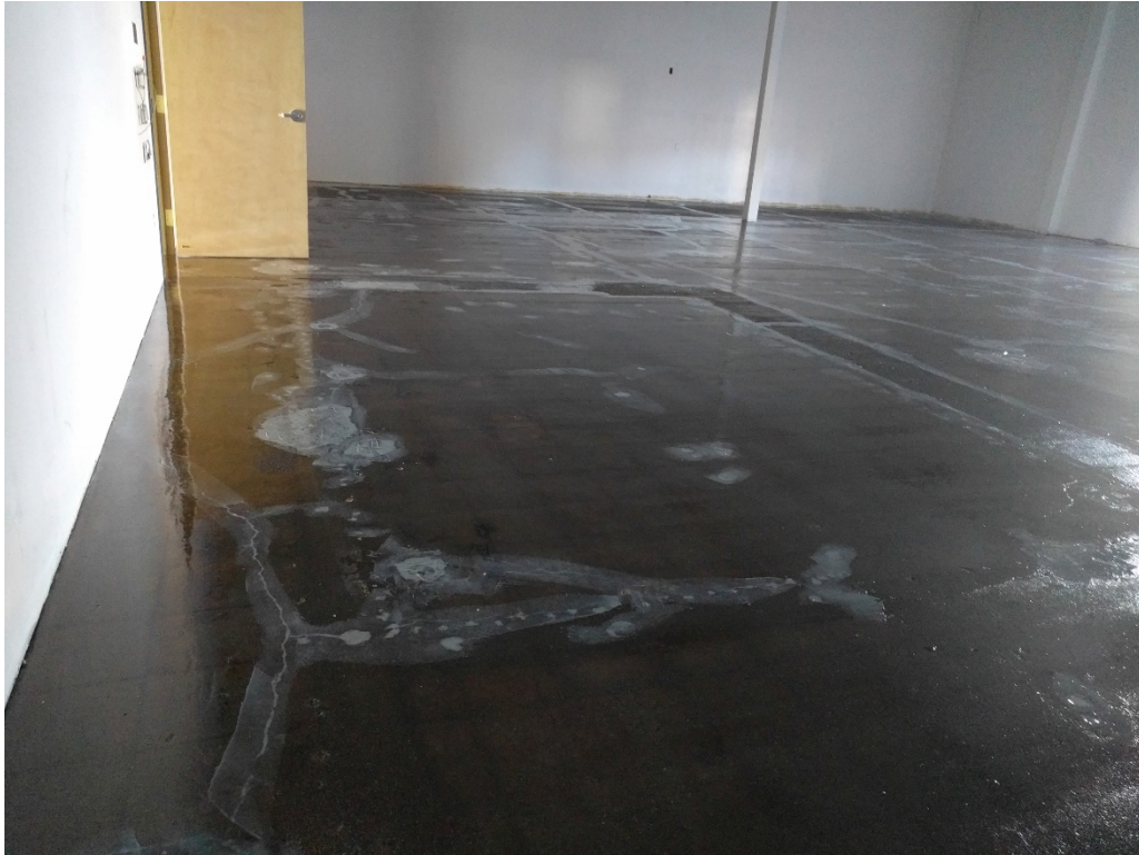
43. Cured primer application. Photo taken from S corner of stock room facing NW as in photo Nos 64 and 90 (03/12/2017)
