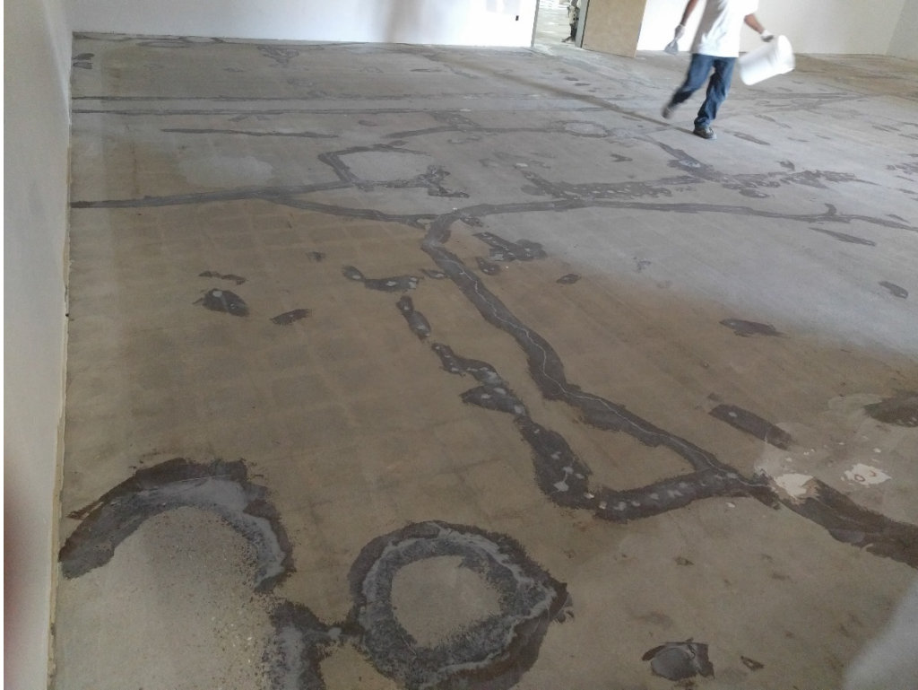
29. Application of Retro-coat Gel to seal cracks post surface preparation, but prior to primer application. Photo taken from N corner of stock room facing SE (03/11/2017)
