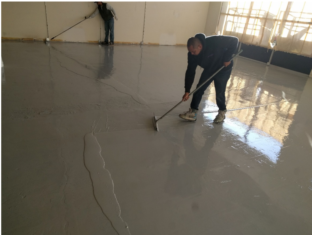
84. Representative squeegee application of Retro-coat Core layer 2. Backrolling visible in the background (03/13/2017)
