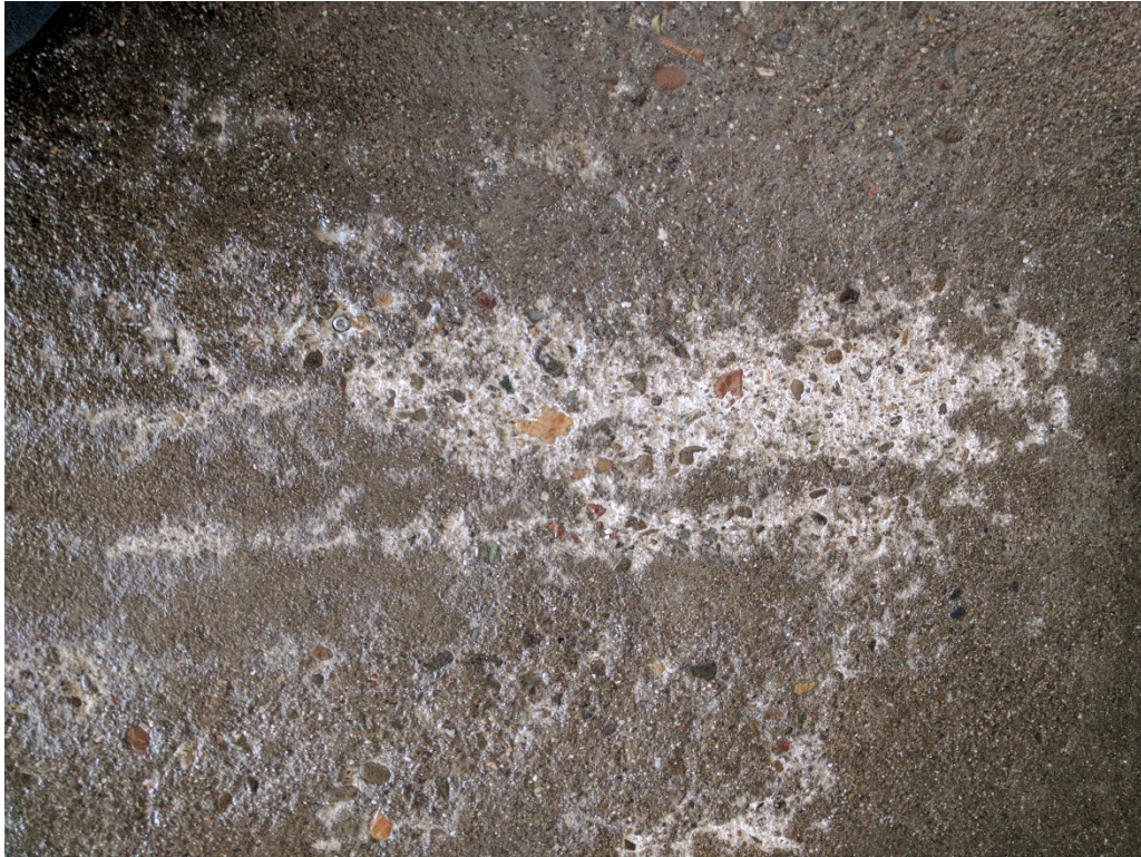
55. Area of primer percolation in high porosity concrete (03/12/2017)
