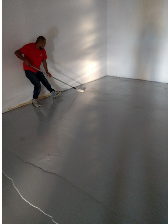
87. Backrolling post addition of sand aggregate to Retro-coat Core layer 2 (03/13/2017)
