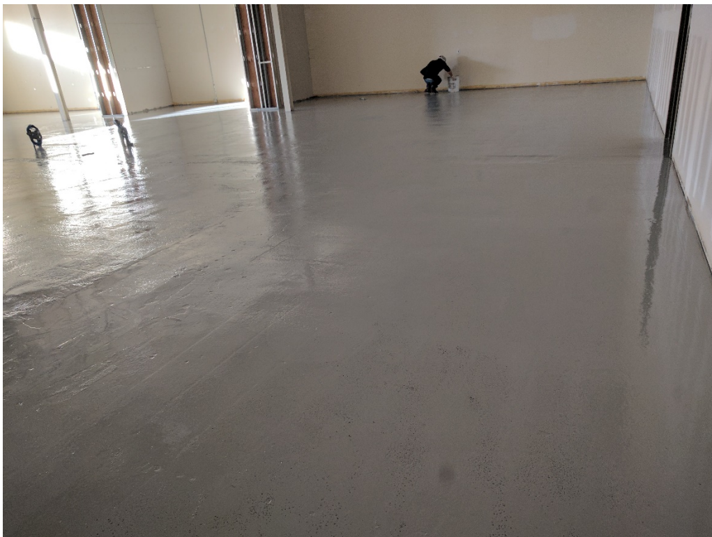
68. Cured Retro-coat layer 1. View from E corner facing W as in photo Nos 47 and 94 (03/12/2017)
