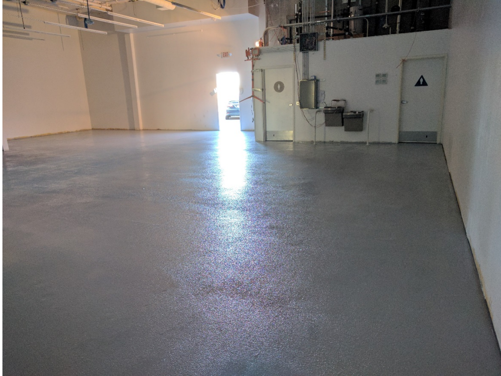
91. Cured and finished Retro-coat Core layer 2 with sand aggregate. Photo taken from S corner of stock room facing NW as in photo Nos 41 and 65 (03/14/2017)
