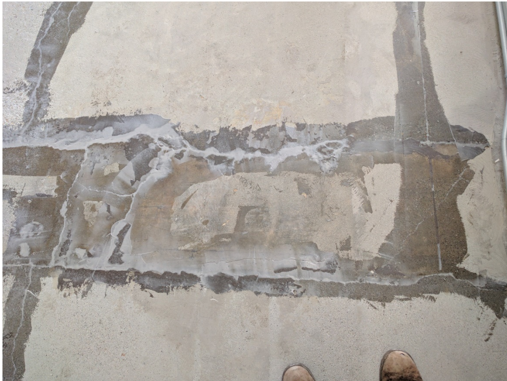
30. Representative Retro-coat Gel application (03/11/2017)
