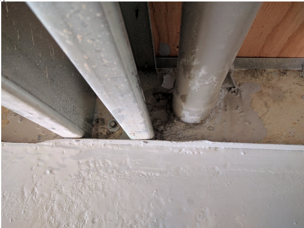
72. Retro-coat Core seal of penetration from ceiling for com/electric to sales floor POS podium as depicted in photo No 13 (03/13/2017)
