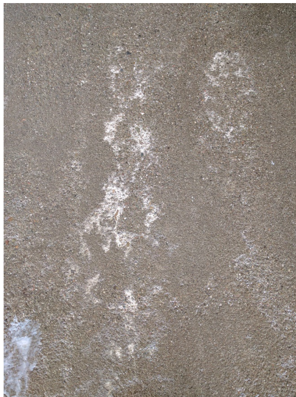
56. Area of primer percolation in high porosity concrete (03/12/2017)
