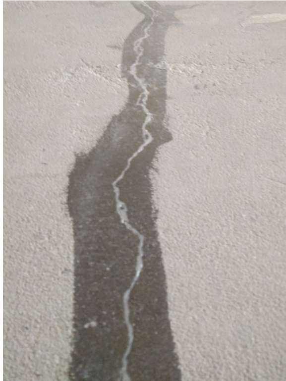
37. Close up of representative crack repair using Retro-coat Gel (03/11)
