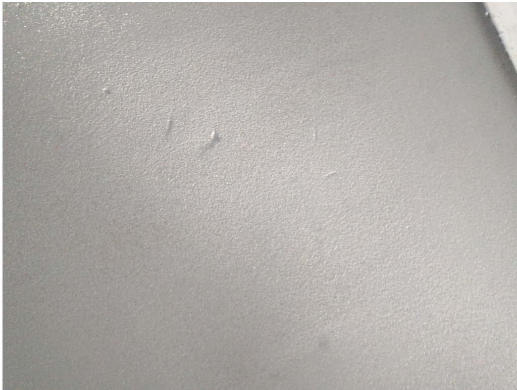
86. Representative sand addition post application of Retro-coat Core layer 2 (03/13/2017)
