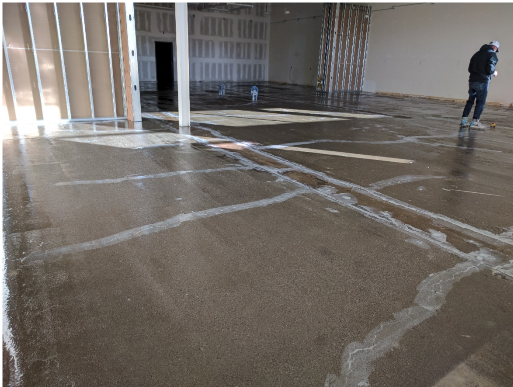
46. Cured primer application. View from S corner of sales area facing N as in Photo Nos 4, 31, 97 (03/12/2017)
