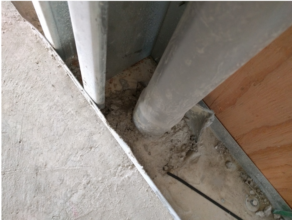
13. Penetration from ceiling for com/electric to sales floor POS podium as in photo No 72 (03/10/2017)
