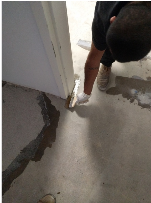
40. Representative application of Retro-coat Primer around vertical terminations using brush (03/11/2017)
