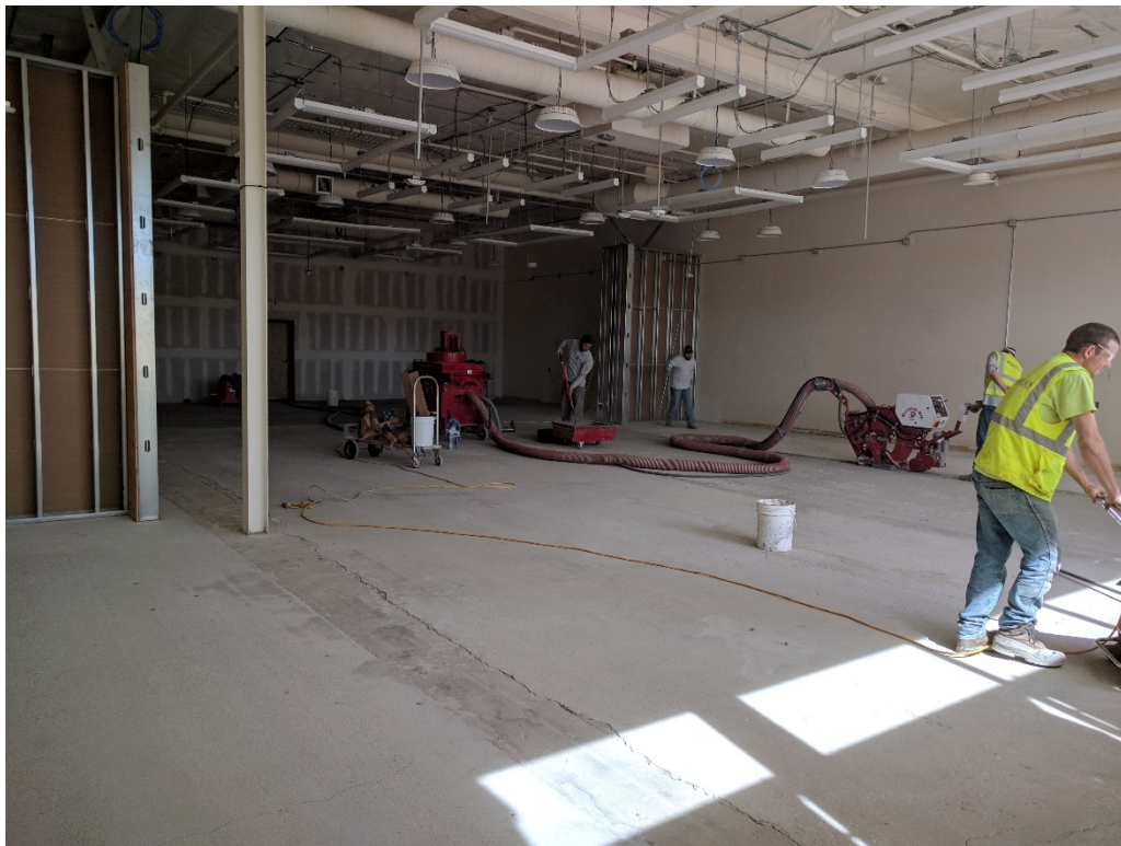
4. Surface abrasion using shot blaster and grinder. View from S corner of sales area facing N as in photo Nos 31, 46 and 97 (03/11/2017)
