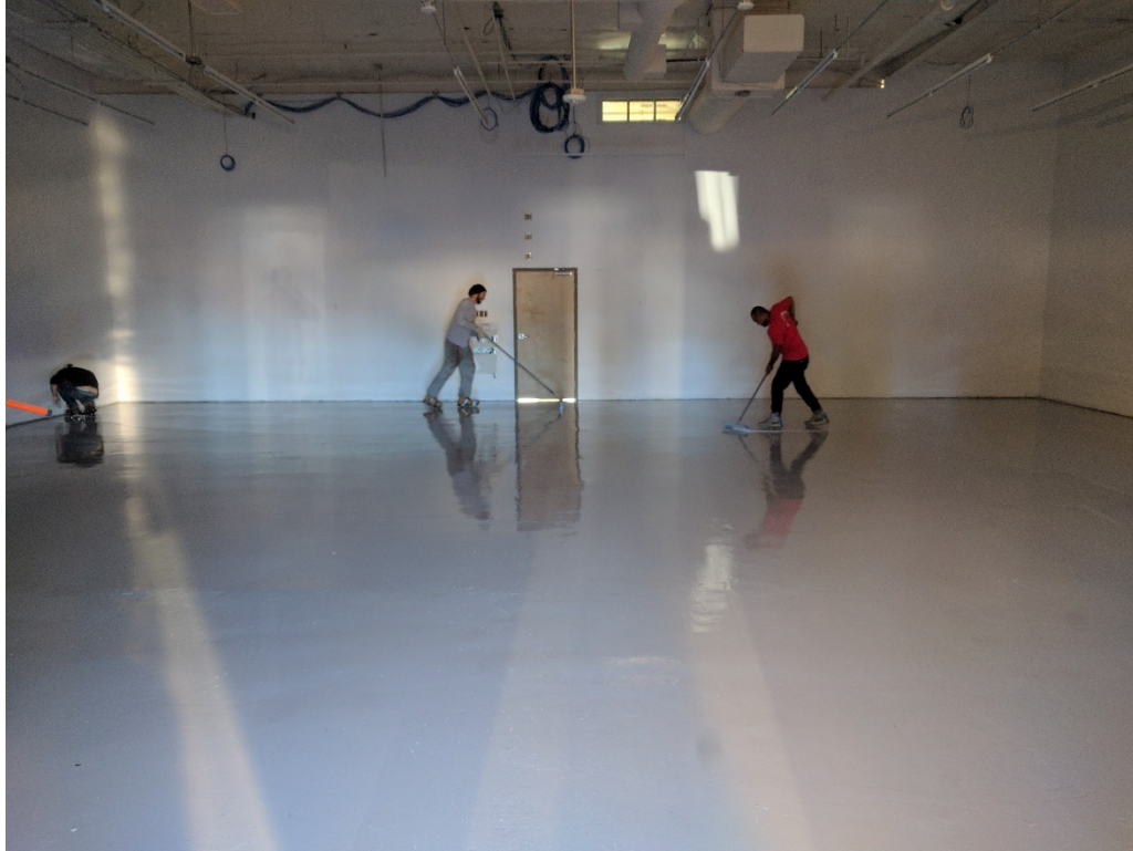
85. Squeegee application and backrolling of Retro-coat Core layer 2 to stock area (03/13/2017)
