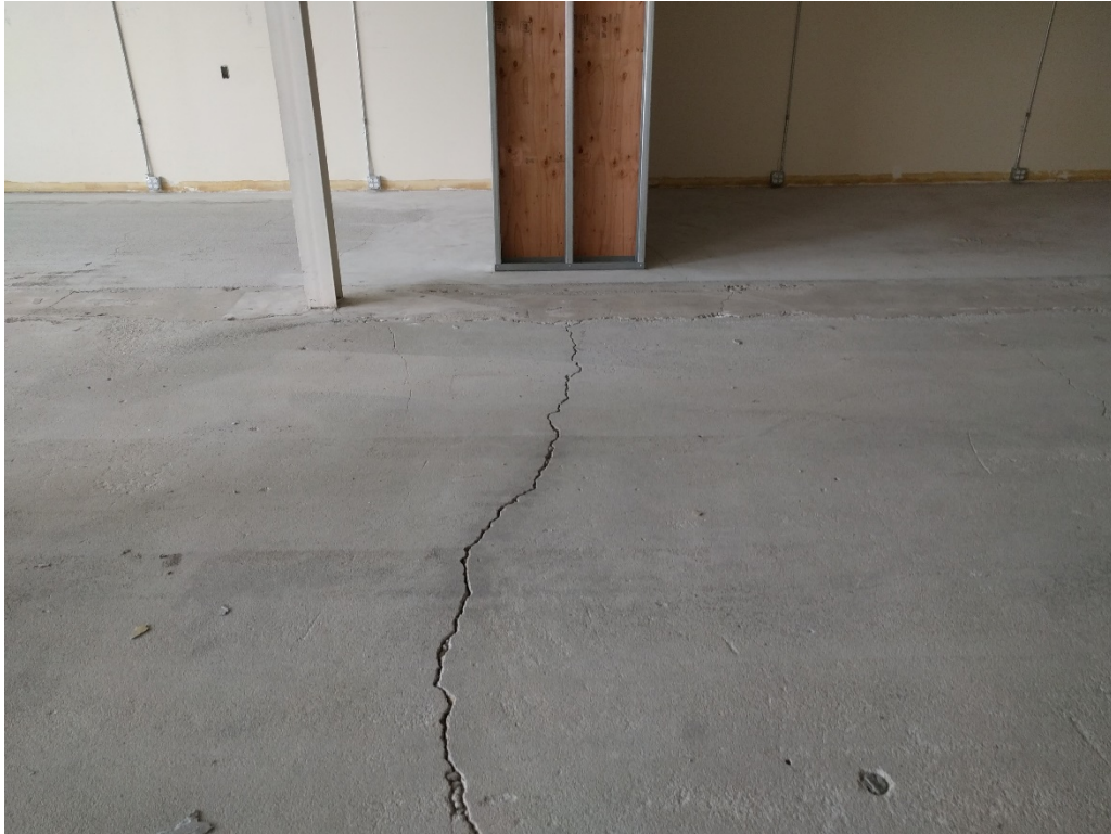
17. Representative cracks post surface preparation (03/11/2017)
