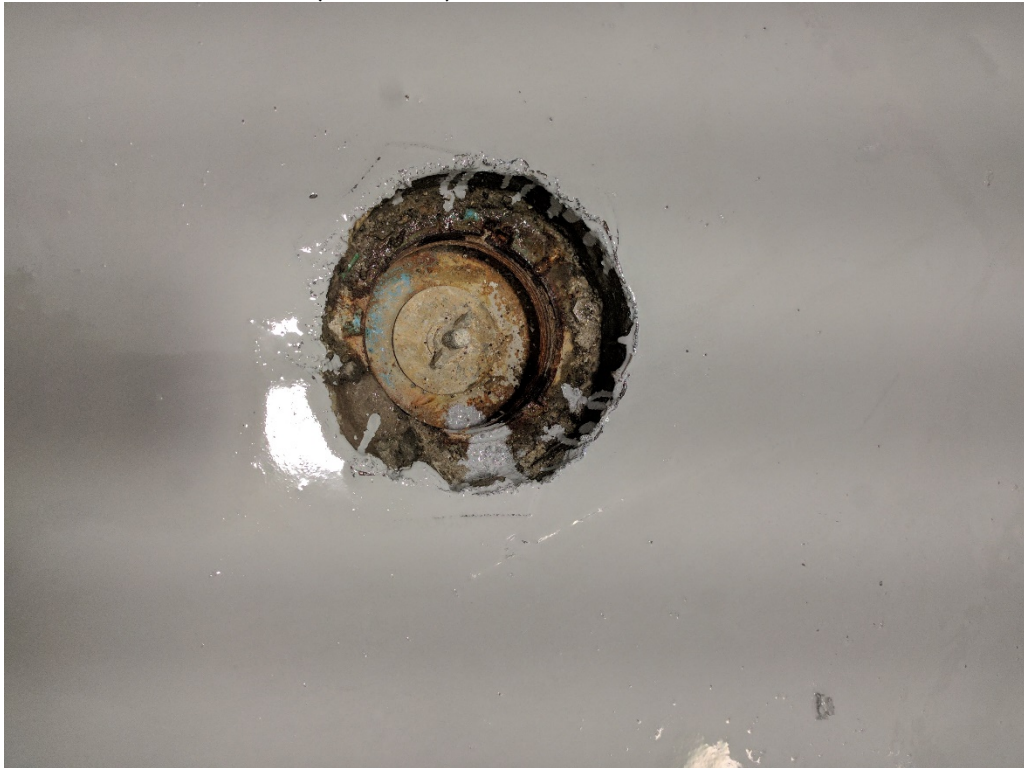
76. Women's restroom penetration Retro-coat Core layer 1 seal (03/13/2017)
