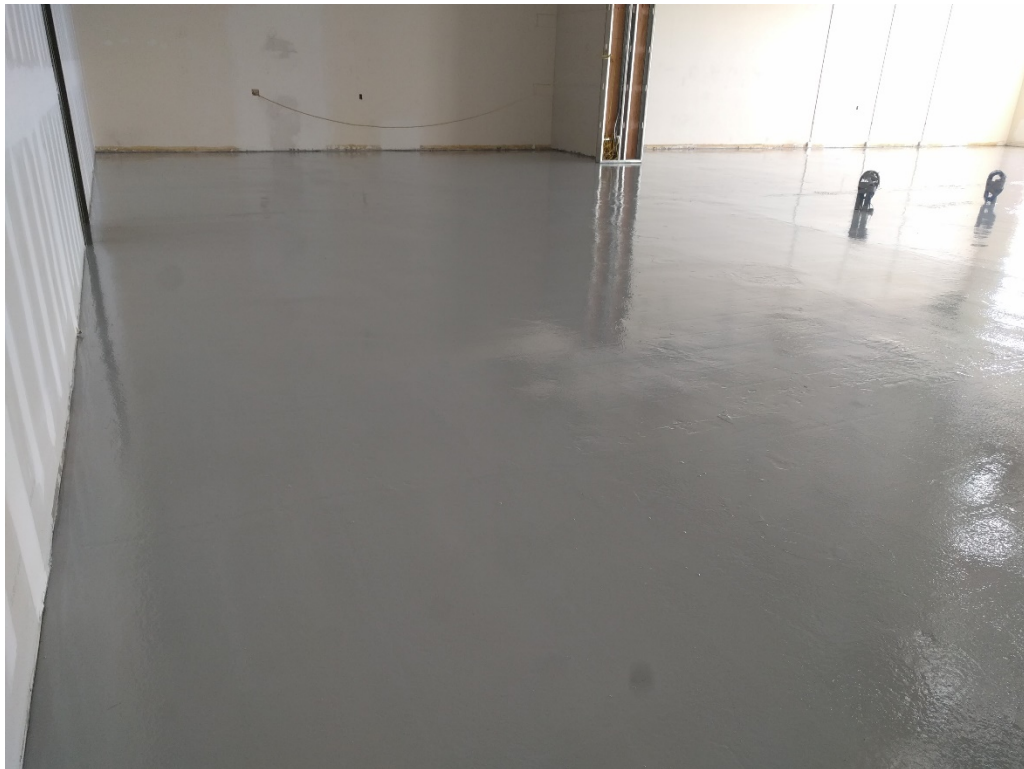
96. Cured and finished Retro-coat Core layer 2. View from W corner of sales area facing NE as in photo Nos 6, 33, and 70 (03/14/2017)
