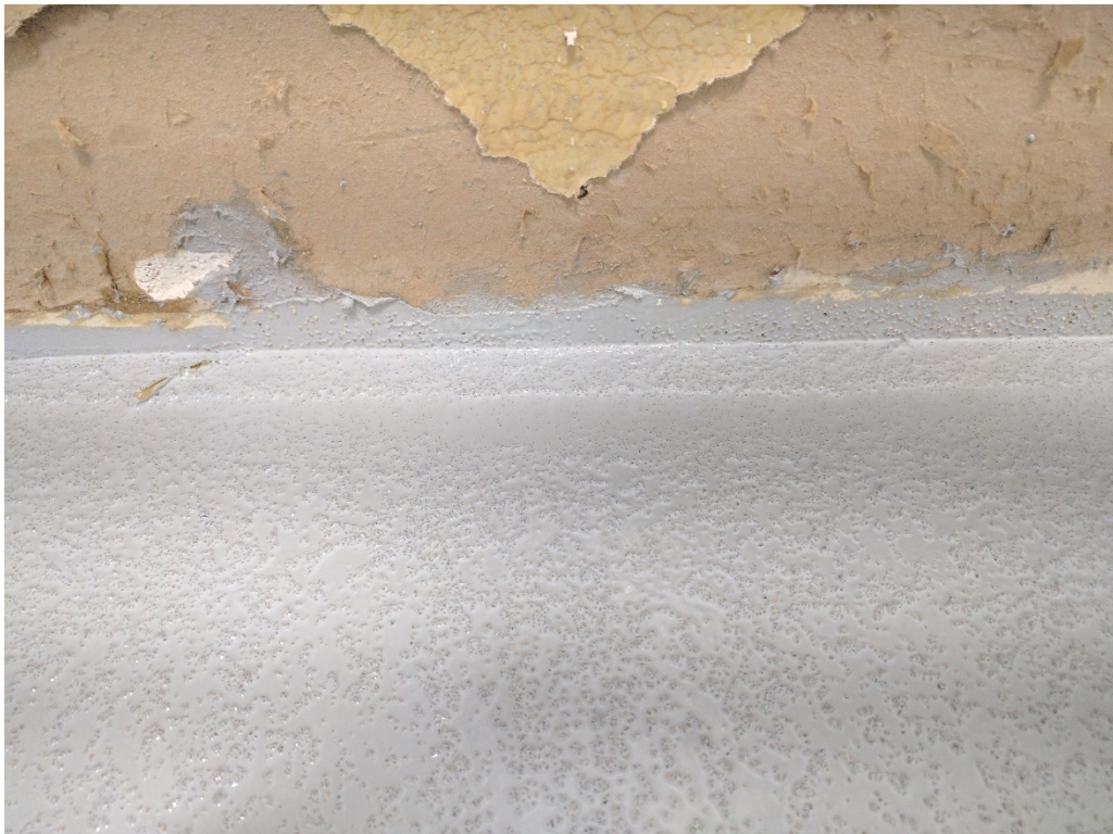
100. Representative cured and finished Retro-coat Core layer 2 at vertical termination as in photo no 80 (03/14/2017)
