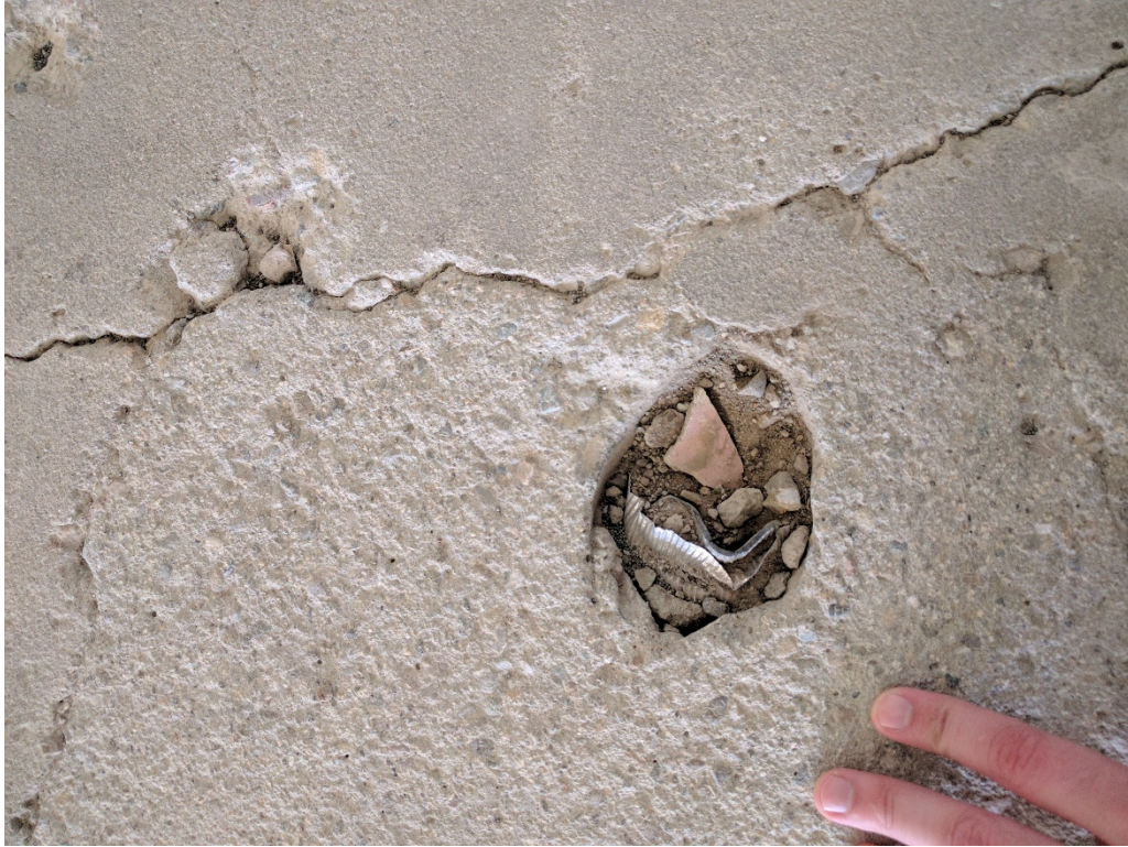
23. Historic electrical conduit identified post surface abrasion (03/10/2017)
