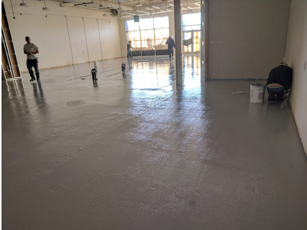
69. Cured Retro-coat Core layer 1. View from W corner of sales area facing SE as in photo Nos 5, 69, and 95 (03/13/2017)
