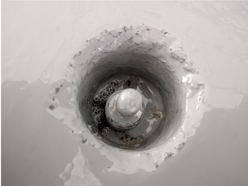
105. Representative cured and finished Retro-coat Core layer 2 at interior of vapor pin (03/14/2017)
