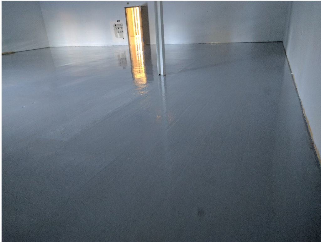
63. Cured Retro-coat layer 1. Photo taken from W corner of stock room facing E as in photo No 89 (03/13/2017)
