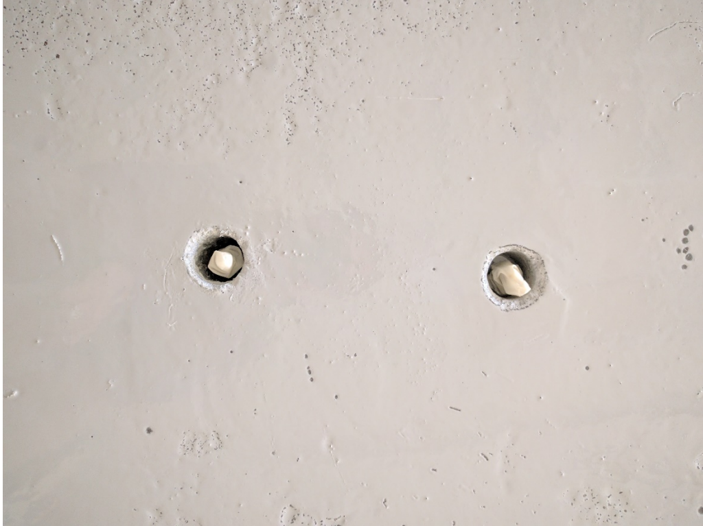
81. Representative cured Retro-coat Core application layer 1 around cox-colvin sub-slab and soil vapor probe locations as in photo Nos (03/13/2017)
