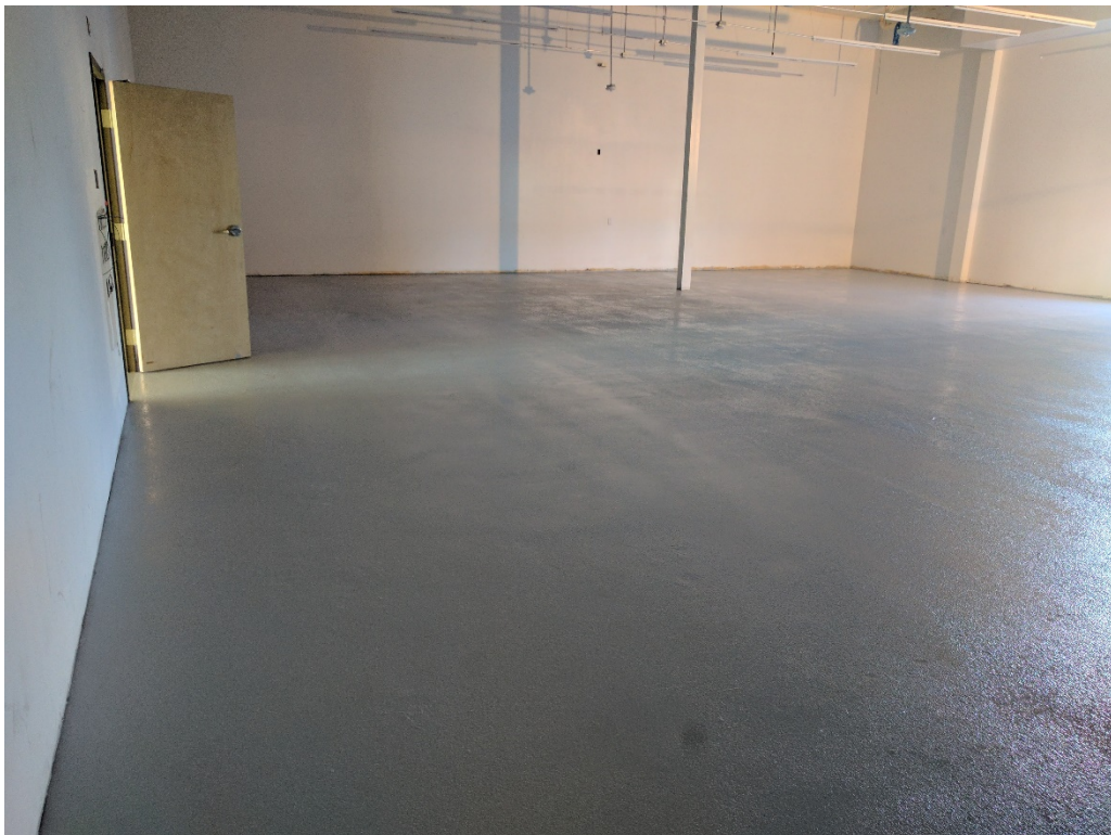
90. Cured and finished Retro-coat Core layer 2 with sand aggregate. Photo taken from S corner of stock room facing W as in photo Nos 43 and 64 (03/14/2017)
