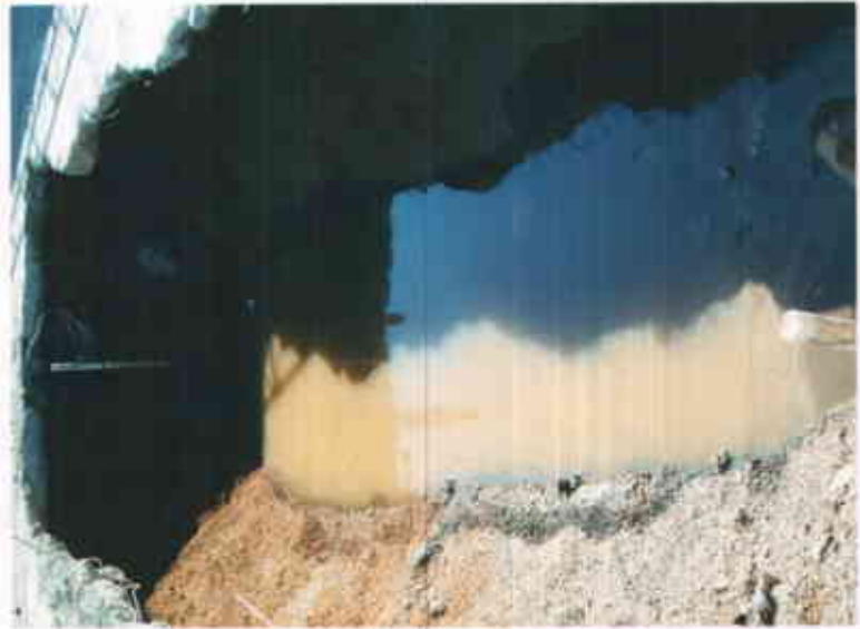
H 2 O IN EXCAVATION DIESEL FLOATING
