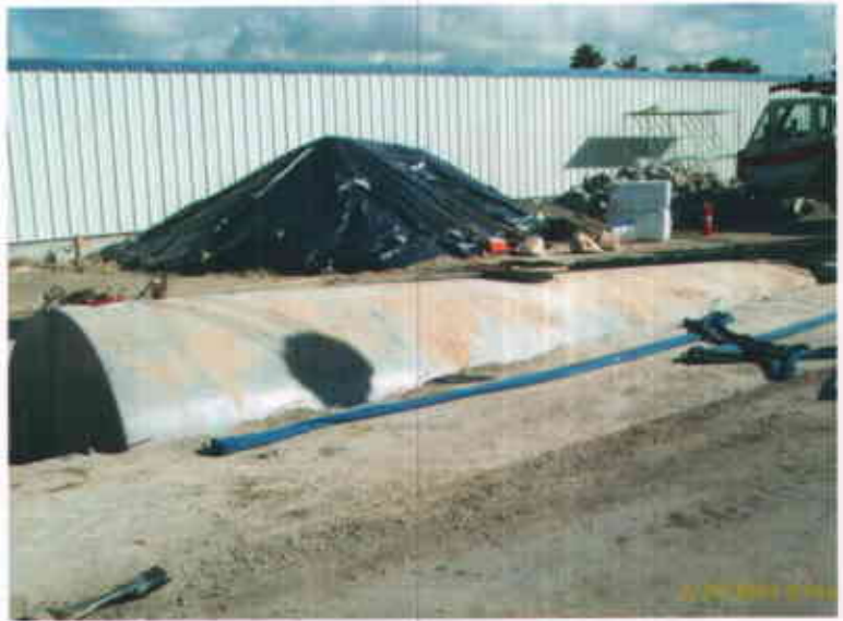
TANK FLOATING IN EXCAVATION
