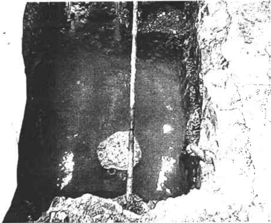
Tank in excavation ready for removal
