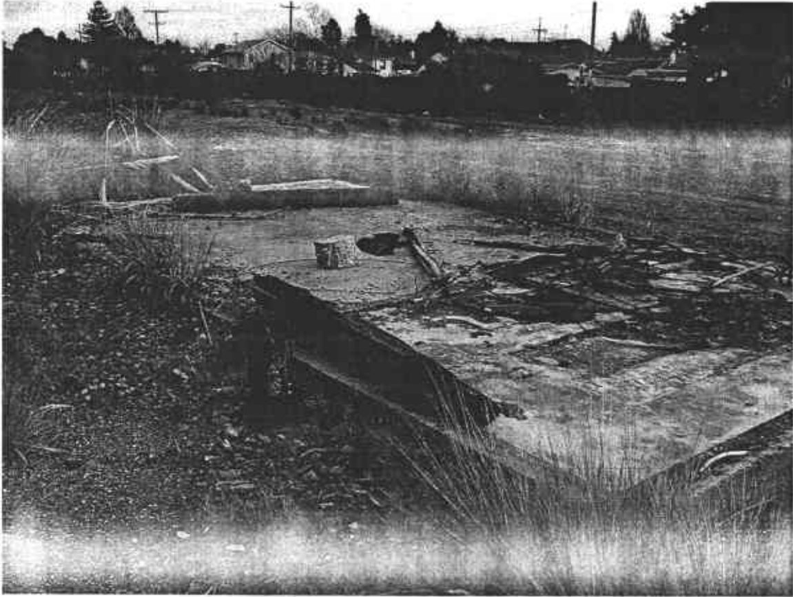
Figure 2. Concrete Pad and Pipe
