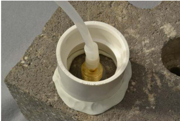
Figure 6. Water dam used for leak detection.
