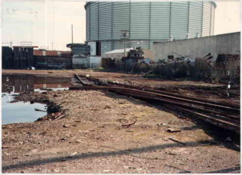
BAILER IS TO THE LEFT. POND W/ FLOATING OIL, CONTAMINATED SOIL
