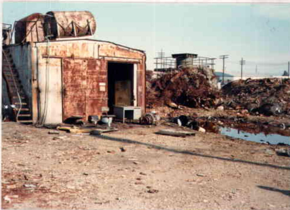
BAILER POND W/ FLOATING OIL, CONTAMINATED SOIL
