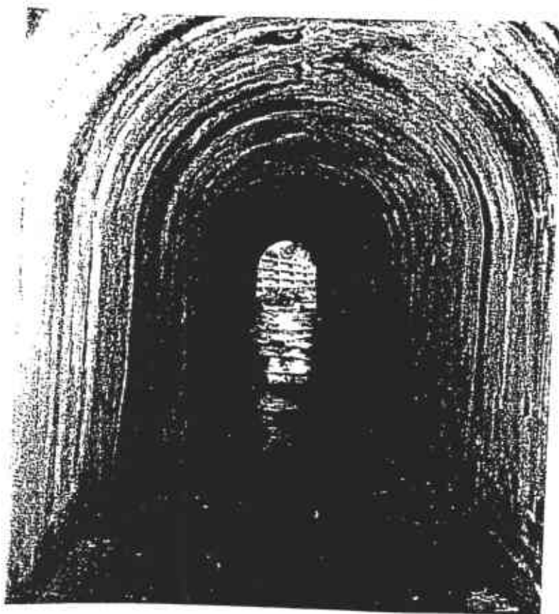
PHOTO 2: A view from inside of culvert (looking north).
