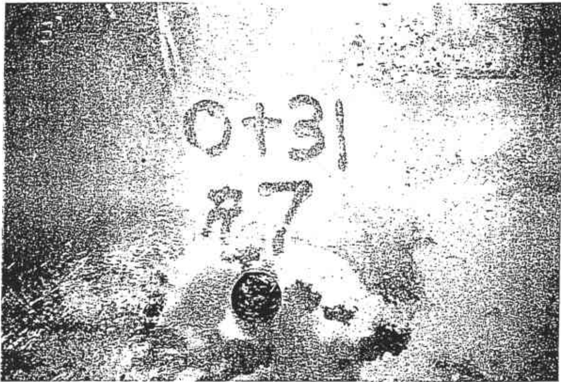
PHOTO 11: A view of cored location @ Sta. 0+31 east.
