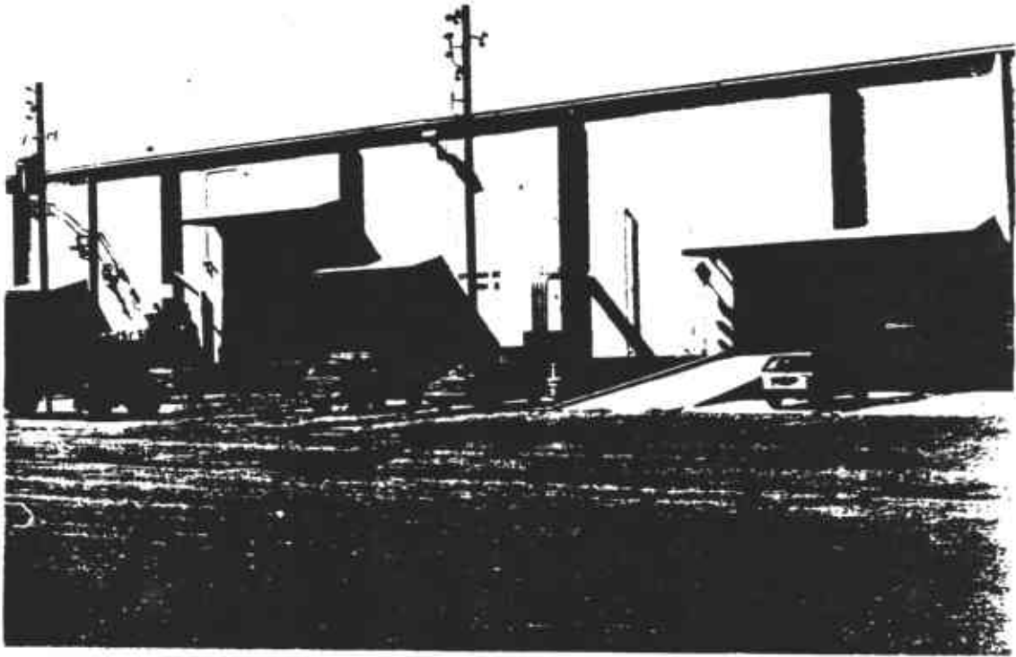
1. NORTHEAST SIDE OF 1964 WILLIAMS STREET WAREHOUSE.
