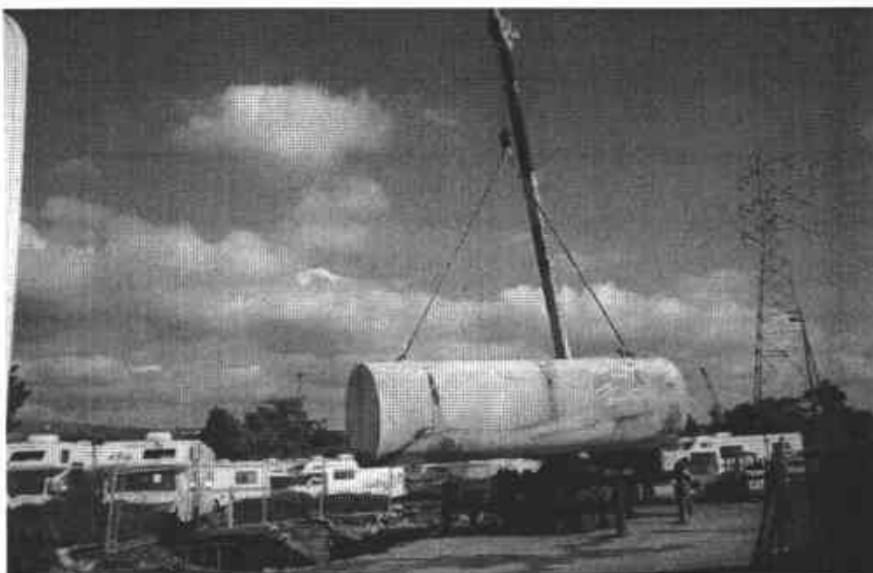
9. The tank is removed from the excavation by a crane.
