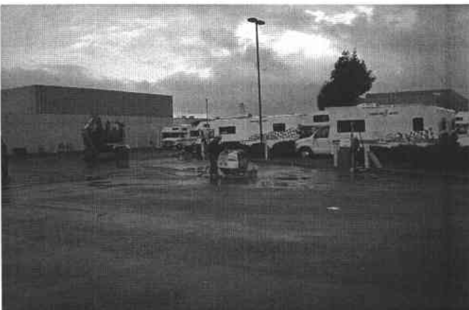
3. Saw cutting of the concrete pad.
