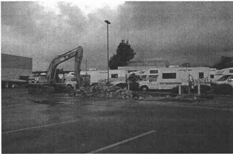
4. Excavator removing concrete pad.
