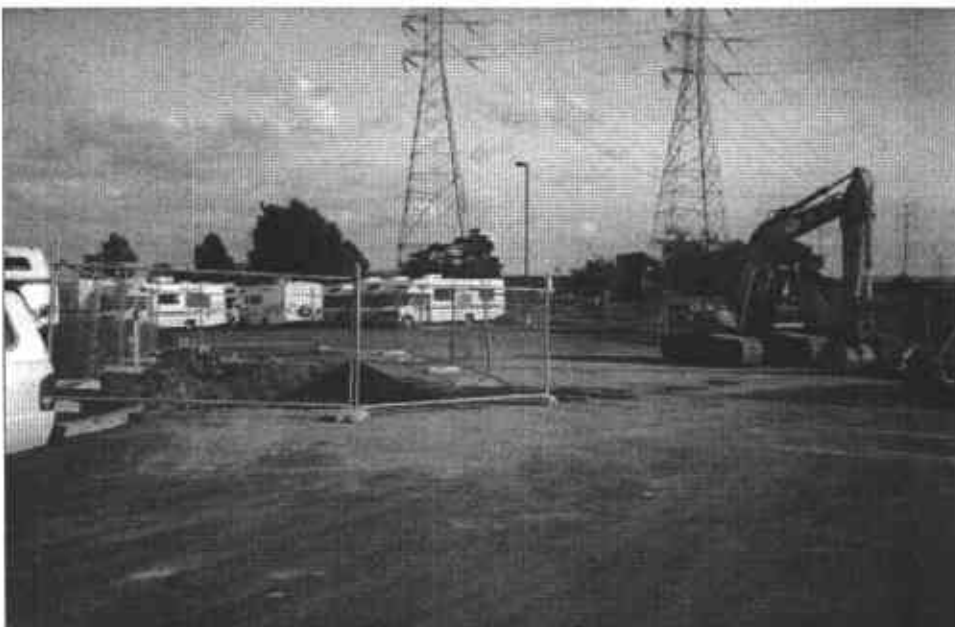
12. The excavation was fenced off at the end of the day.
