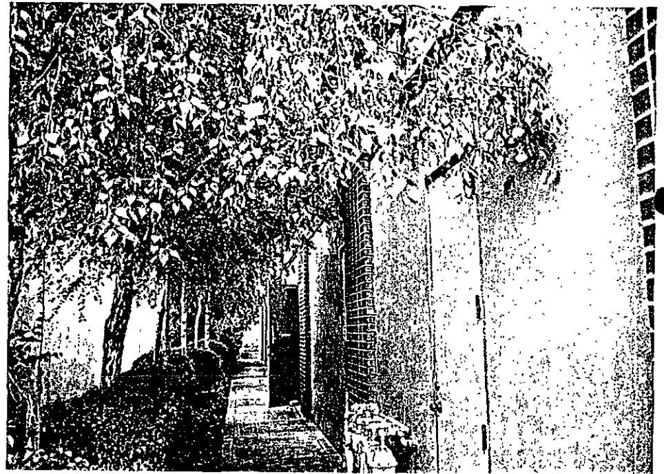
DUBLIN RETAIL CENTER REAR OF BUILDING
