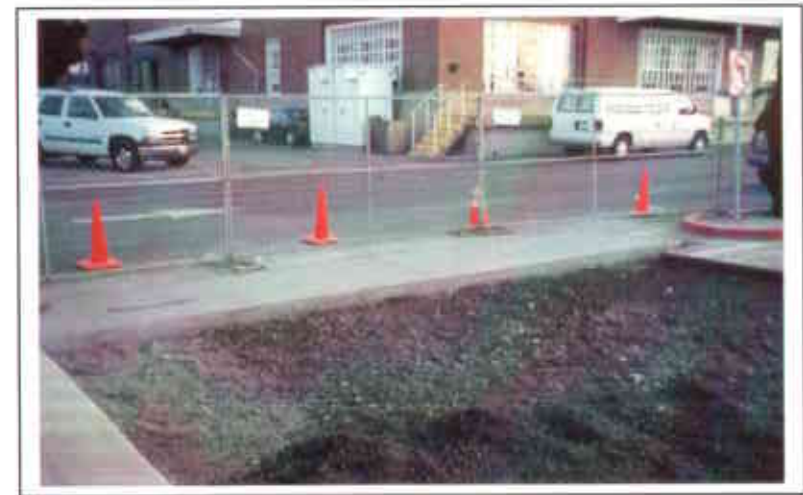
Photo 37. New gutter on northeastern side of excavation.
