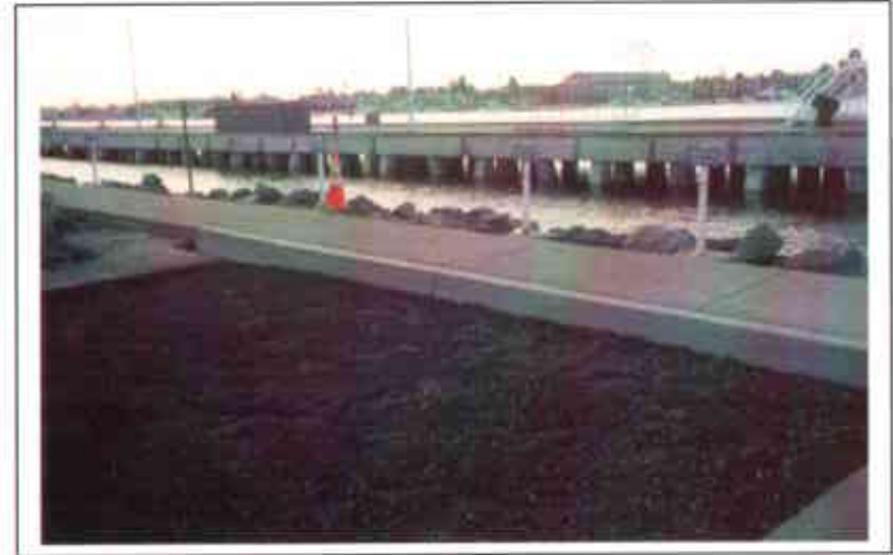
Photo 36. New curb on southwestern side of excavation.
