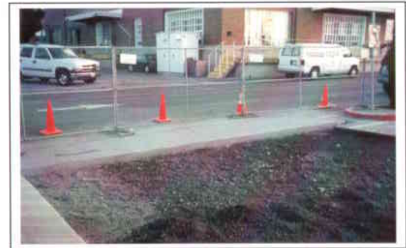
Photo 37. New gutter on northeastern side of excavation.
