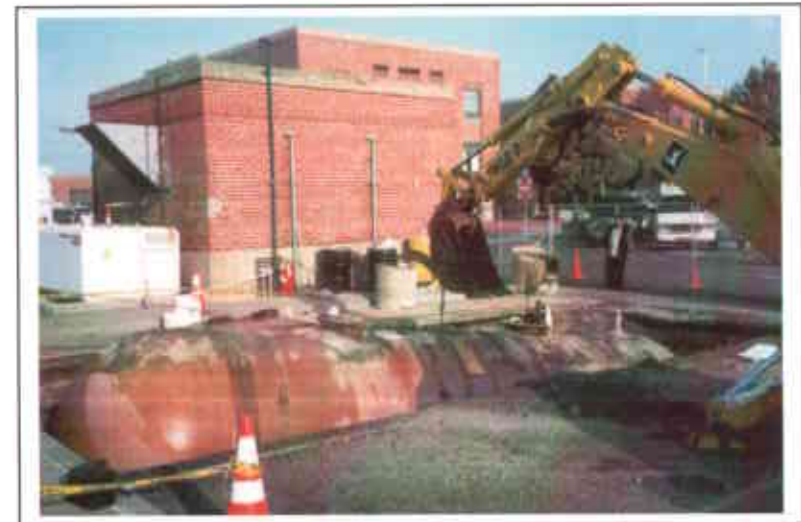
Photo 8. Tank being pulled after cutting of piping.
