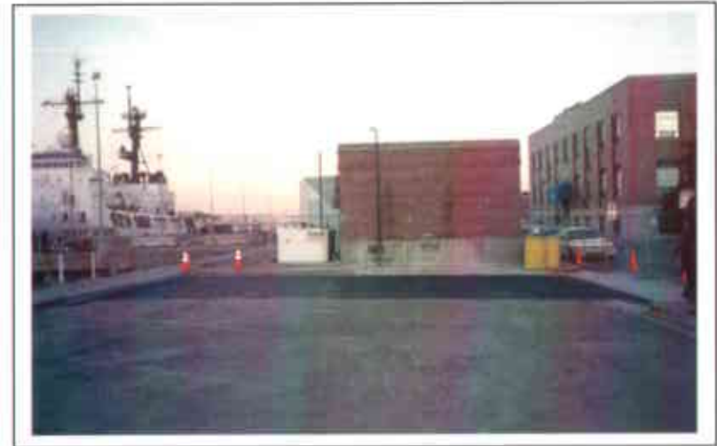
Photo 39. Overview of site after completion of tank closure.
