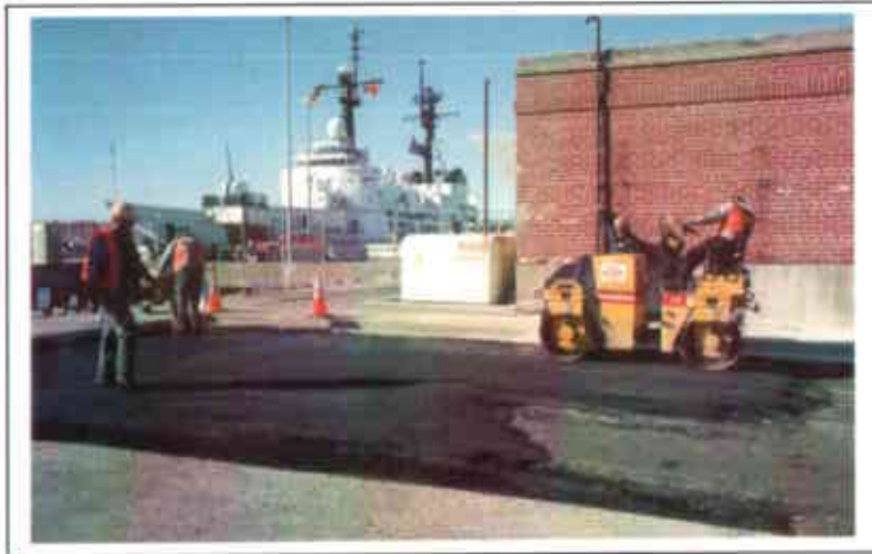
Photo 38. Application of asphalt.
