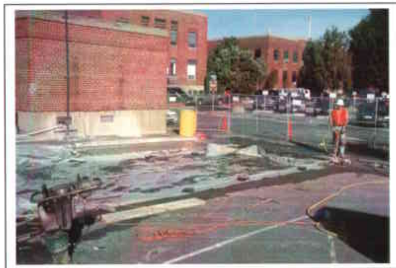
Photo 34. Removal of undermined gutter before repouring with concrete.
