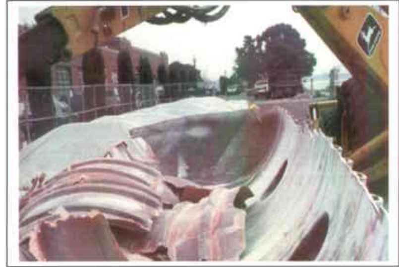
Photo 18. Completion of tank destruction.
