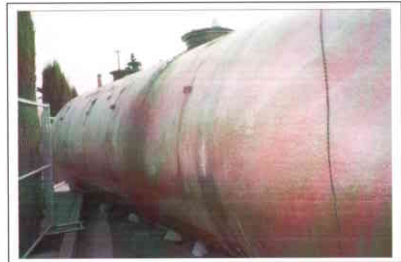
Photo 12. Northern side of tank.
