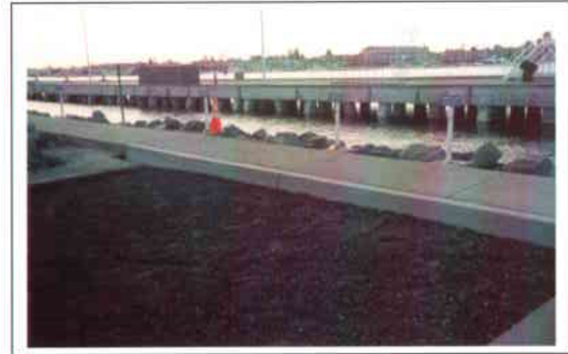
Photo 36. New curb on southwestern side of excavation.
