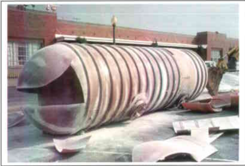
Photo 17. Beginning of tank destruction.
