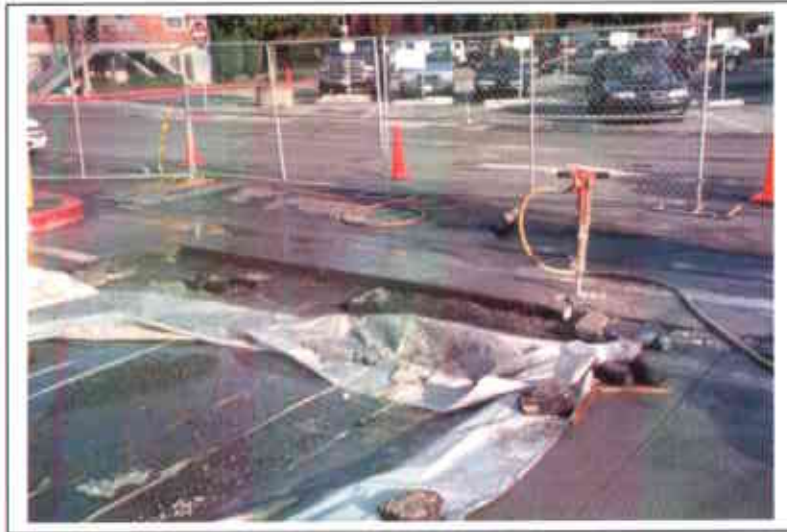
Photo 32. Removal of undermined concrete gutter on northeastern side of excavation pit.
