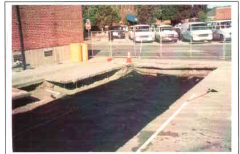
Photo 27. Geotextile fabric above pea gravel. The gravel rock layer will be compressed on top of it.
