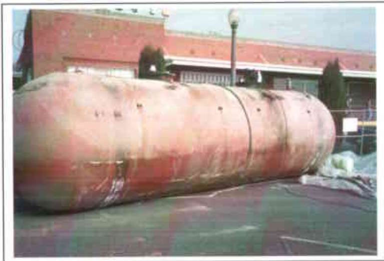
Photo 11. Southern side of tank.
