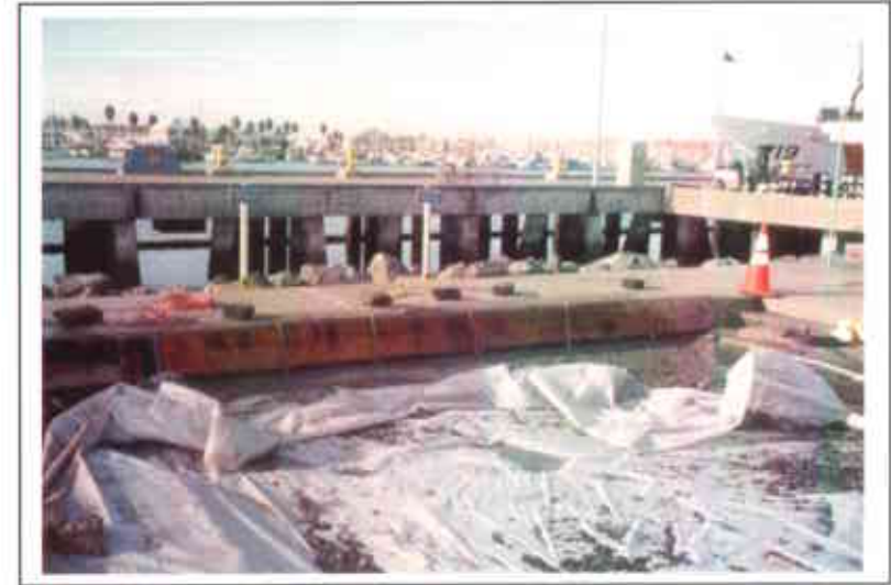
Photo 33. Preparation for pouring of new curb.
