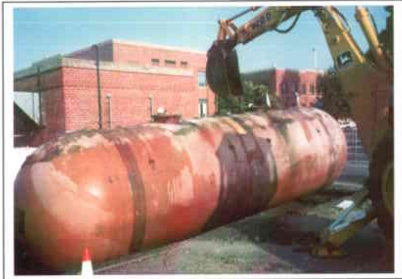
Photo 9. Tank was being removed in one complete piece from excavation.
