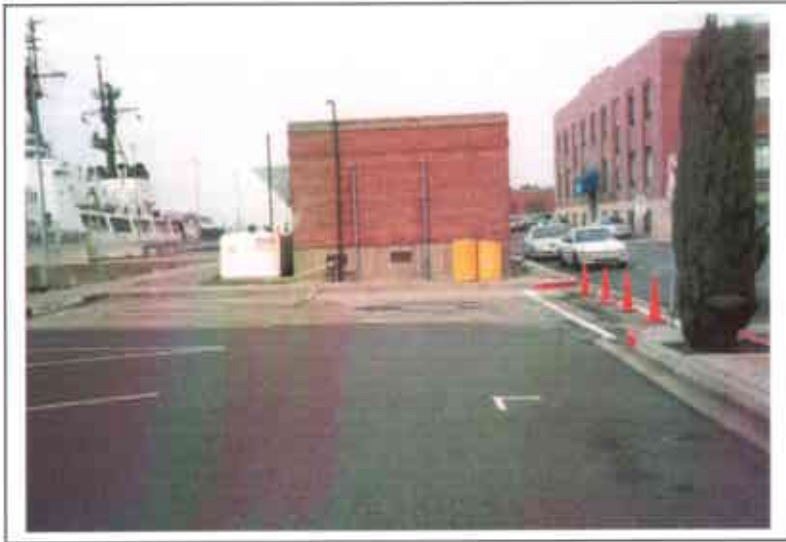
Photo 1. Overview of UST tank site before excavation towards northwest. The tank site is located on parking lot in front of Building 44. The bay is located to the left of Building 44.
