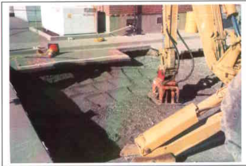
Photo 28. Gravel rock compaction process.
