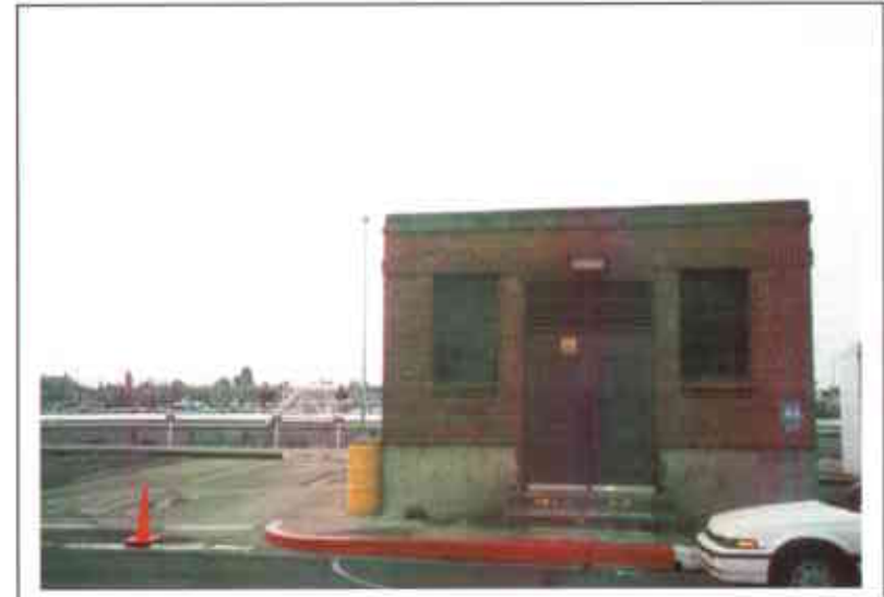
Photo 2. Overview of UST tank site before excavation towards southwest. The bay is located behind Building 44.
