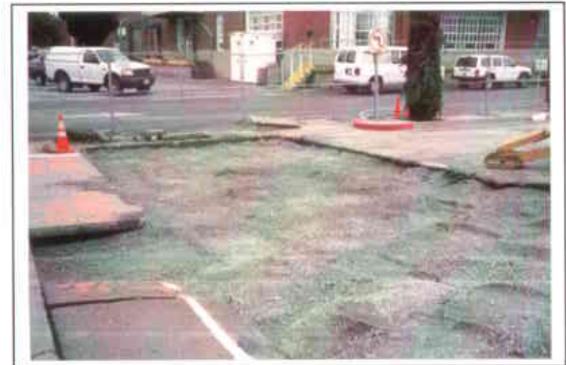
Photo 31. Compacted excavation area.
