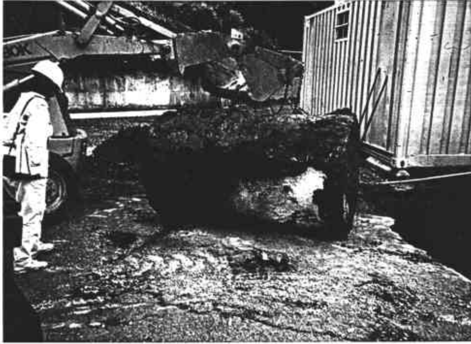
Waste oil tank 15422 immediately after removal from the tank pit.
