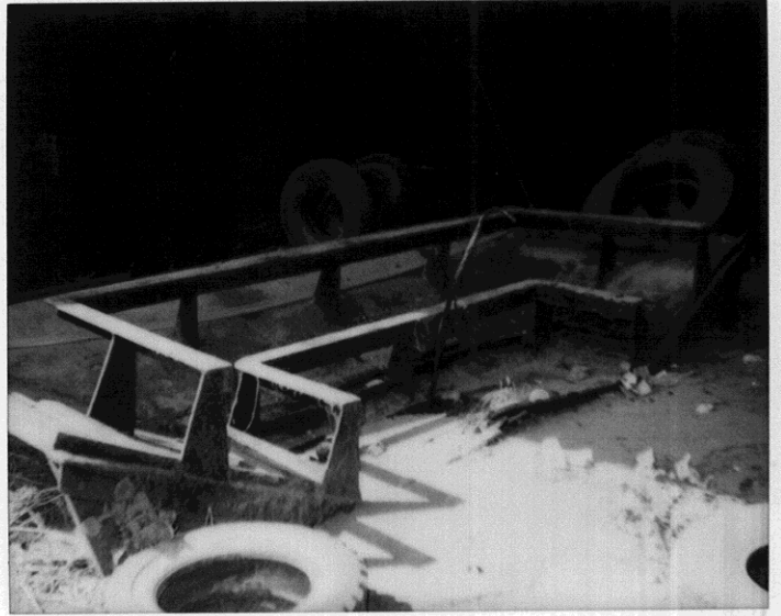
Sump containing Barry substance next to Vicker's Concrete. Buettner & Hoyt property Meekland Av., Hayward. 5-30-91
