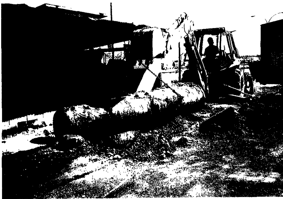
Photograph 1. Underground Storage Tank Being Removed from the Excavation
