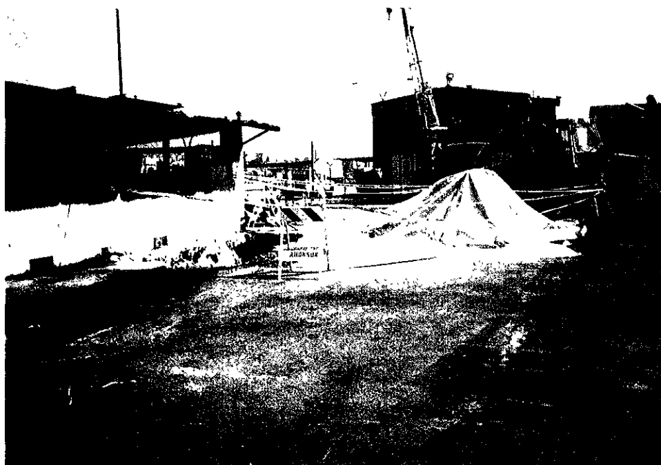
Photograph 4. Current Condition of Underground Storage Tank Excavation and Stockpile Site (November 1991)
