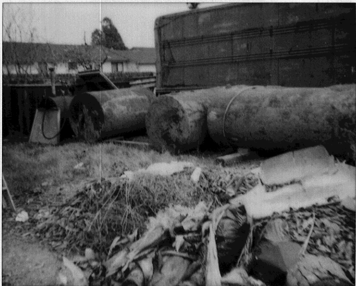
848 Blossom Way, Hayward 2-21-91 4 Tanks 3 at 500 gal Rear of property 1 ~ 1000 gal
