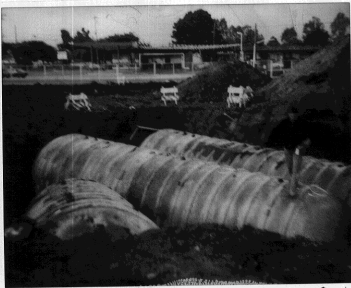
997 Grant Av., San Lorenzo. 12-18-90. 3 fuel tanks before removal.
