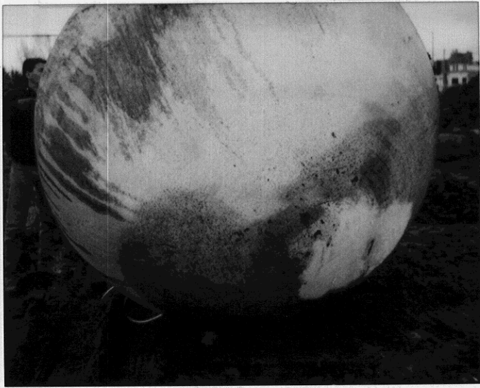
997 Grant Av. San Lorenzo. 12-18-90. Waste oil tank - bottom. No noticeable breaches.
